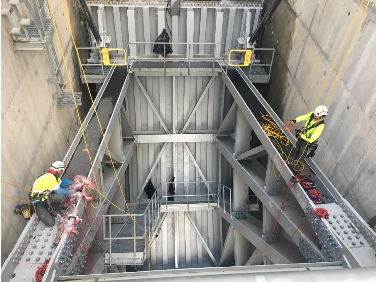
Figure 7 Folsom Dam Control Gates – USACE / Bureau of Reclamation, Folsom, CA
