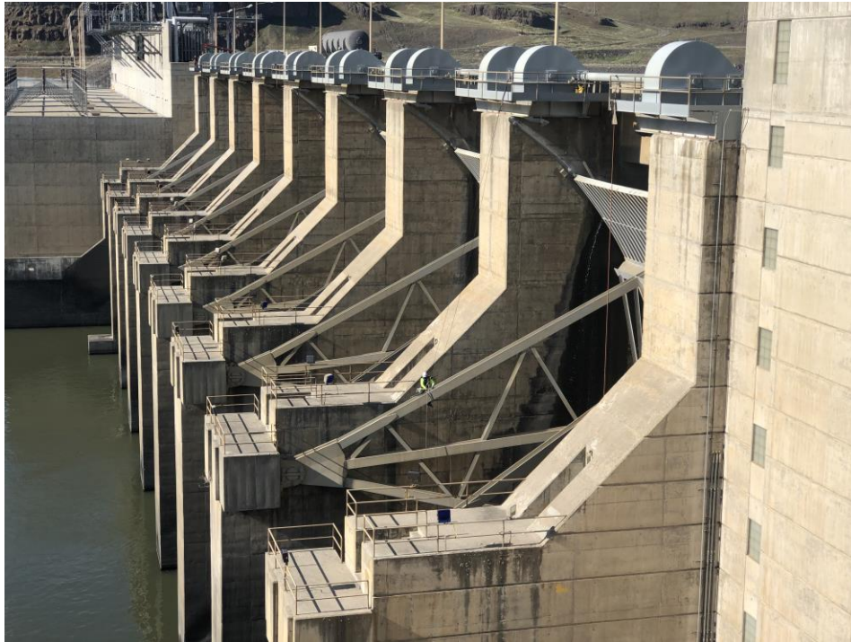
Figure 5 Lower Monumental Lock & Dam, Kahlotus, WA – USACE – Walla Walla District
