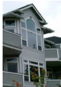
Windows with visually prominent trim
