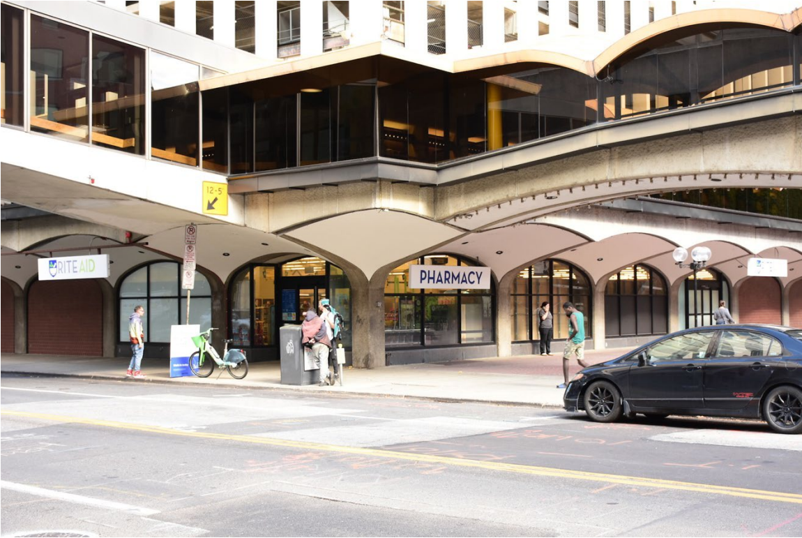
13. Southwest corner-west façade, Rite Aid main entrance, looking northeast (10/2023)
