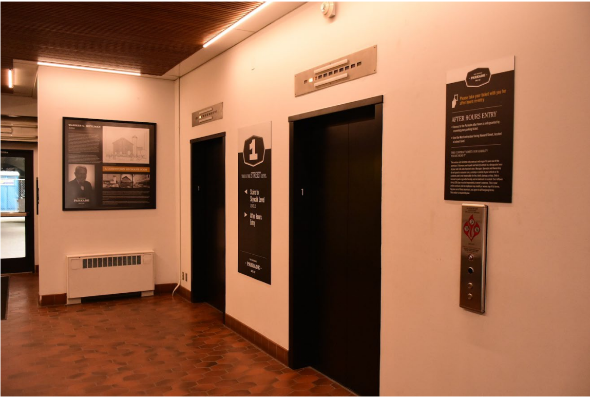
21. Ground floor - elevator/stair lobby looking east (9/2023)
