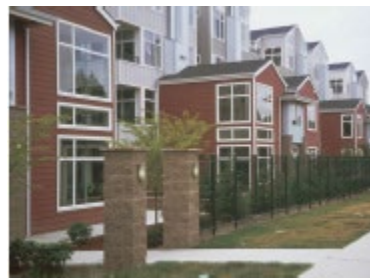
Windows facing street
