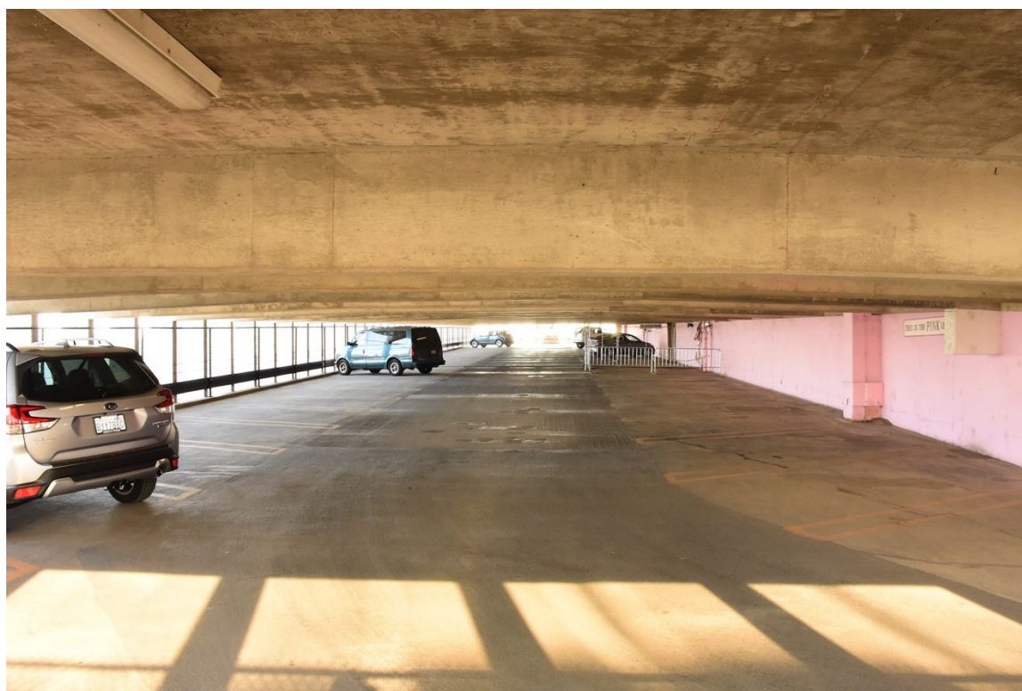
32. Pink level parking ramp - north side, looking east (9/2021)
