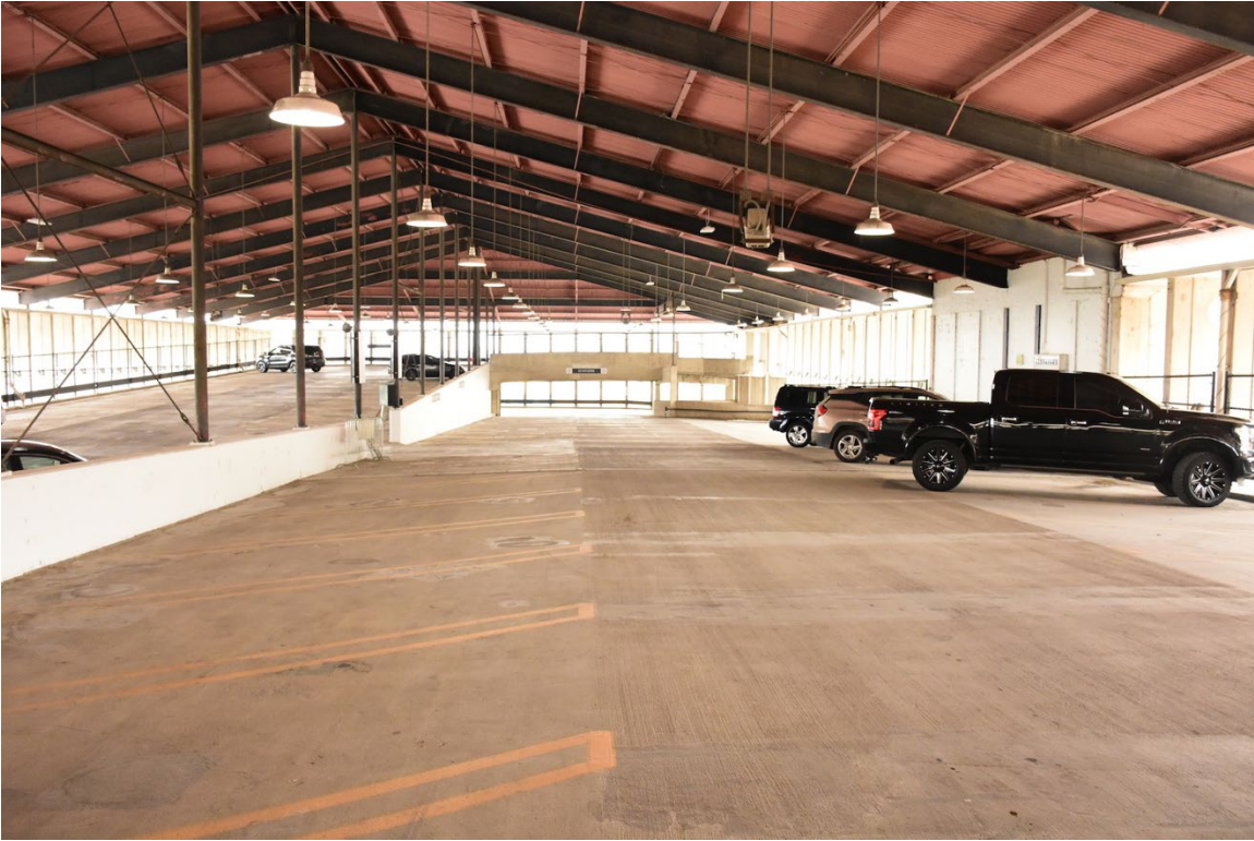
33. Top floor (yellow) showing ramps, lighting and roof structure, looking east (1/2021)
