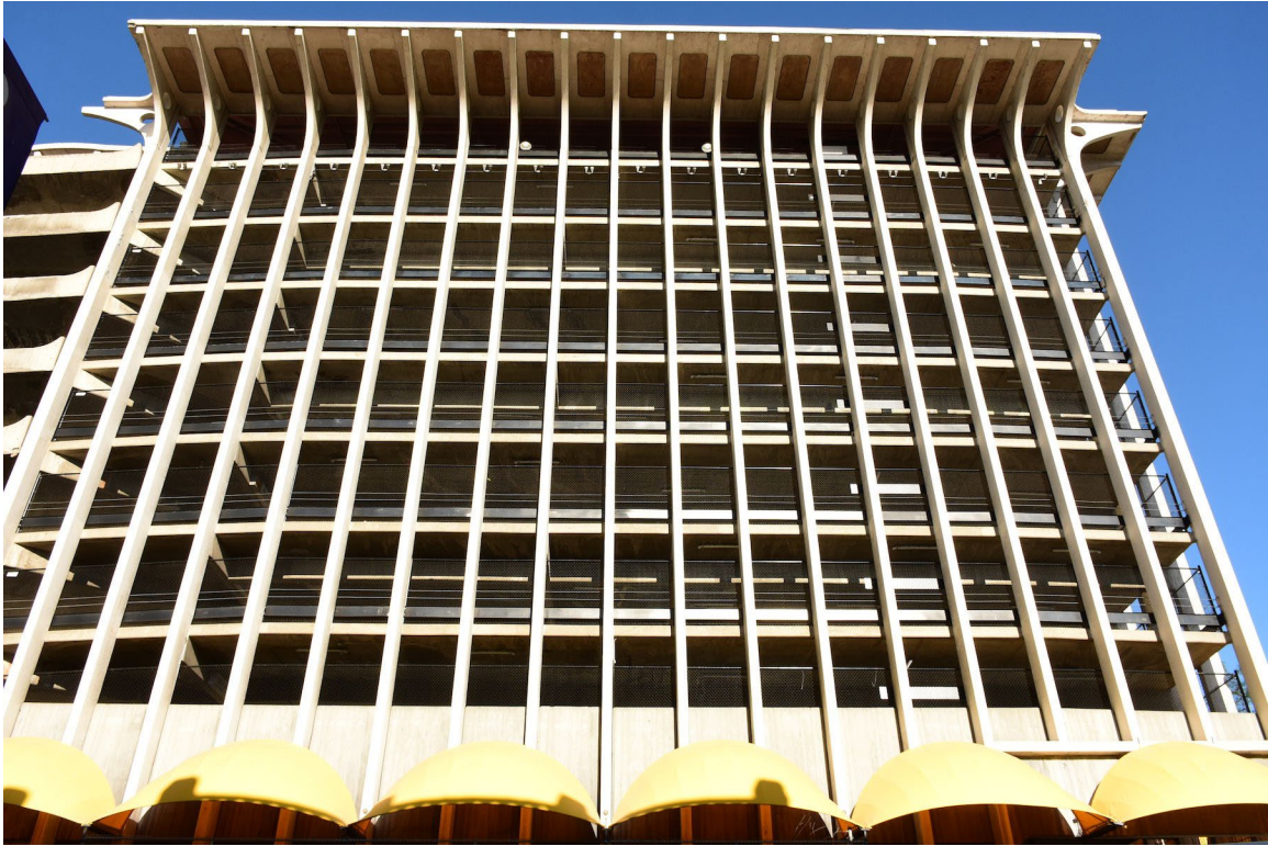
10. East facade, floors 2-10, looking west (7/2023)
