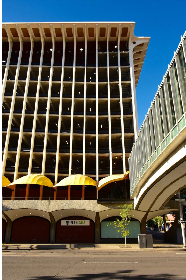
5. West end of north façade, skywalk across Main Avenue on west, looking south (9/2023)
