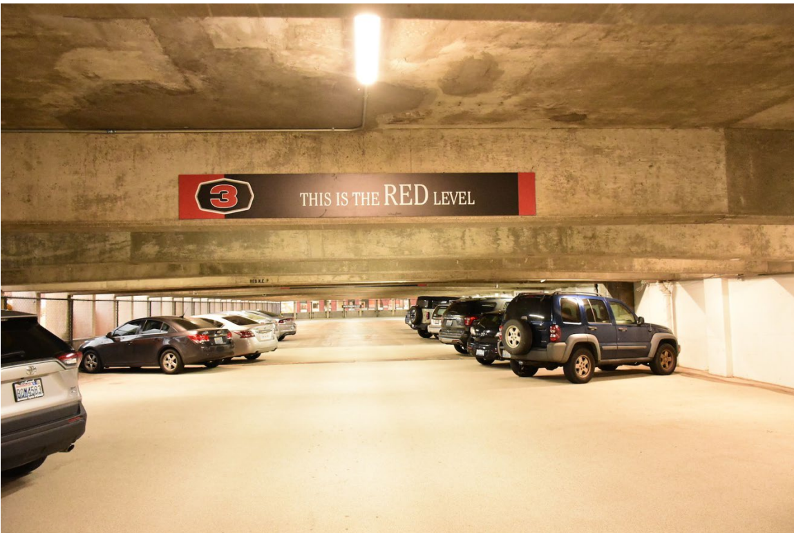
30. Red level (floor 3)- ramp deck drive lane and stalls, looking west (10/2023)
