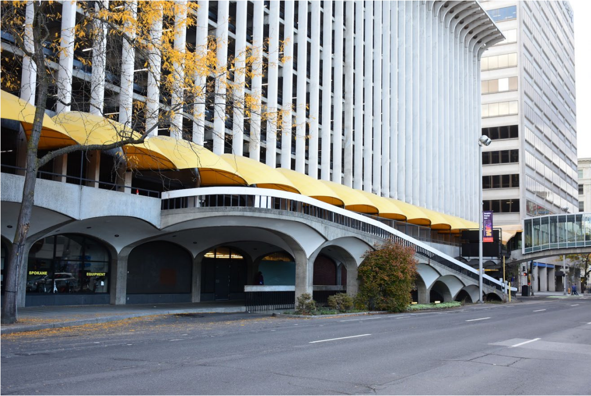
6. North facade - ramp from Main Avenue to parking garage entry, looking west (10/2023)
