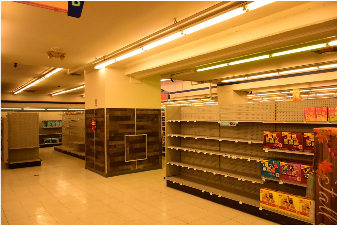
16. Ground floor (Rite Aid) - central column and beam repaired (9/2023)
