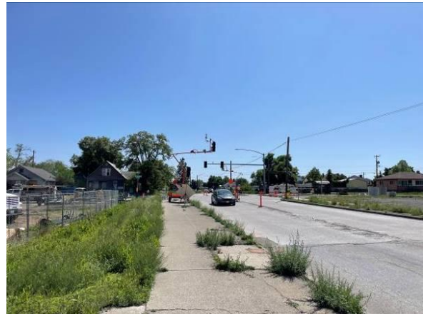
View of North Haven Street Facing South
