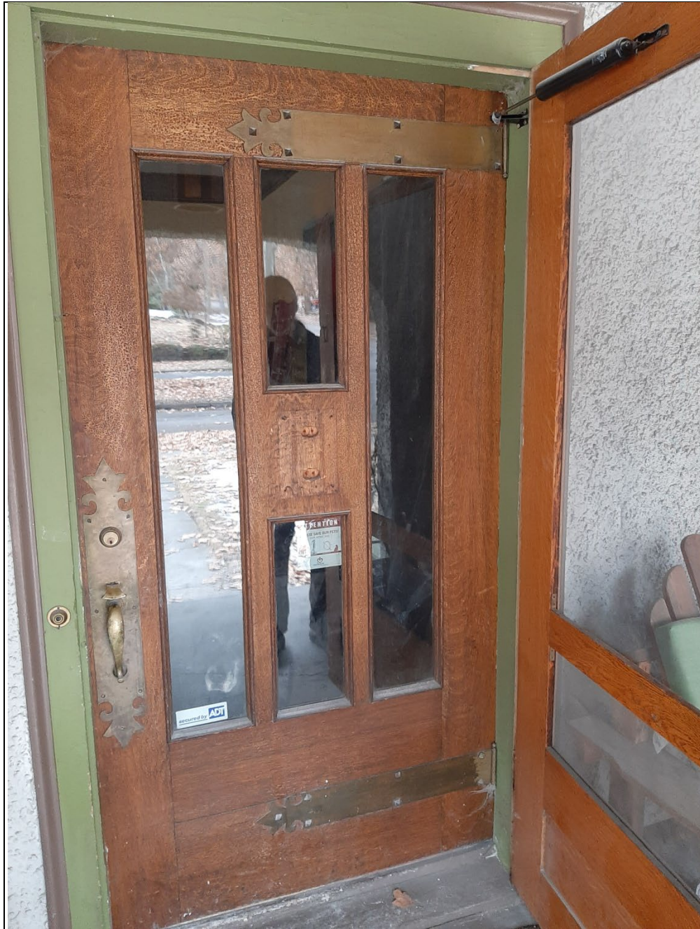
Photo 9 The circa-1914 solid oak front door of the Ritter House in 2023 with its original design and brass hardware
