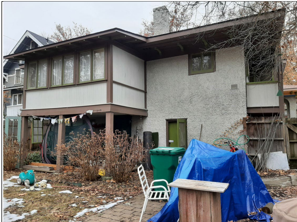
Looking south at the north rear elevation of the Ritter House in 2023
