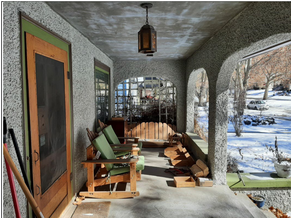
Photo 4 The south facade front porch of the Ritter House, looking east in 2023
