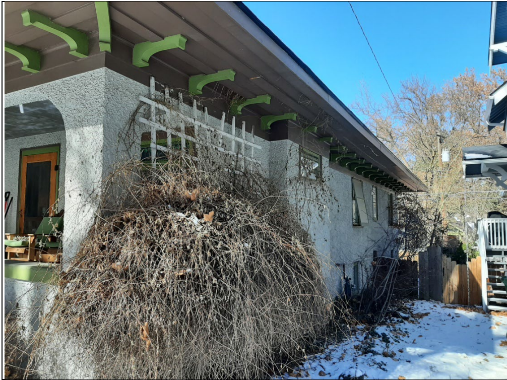
Looking north at the east elevation of the Ritter House in 2023
