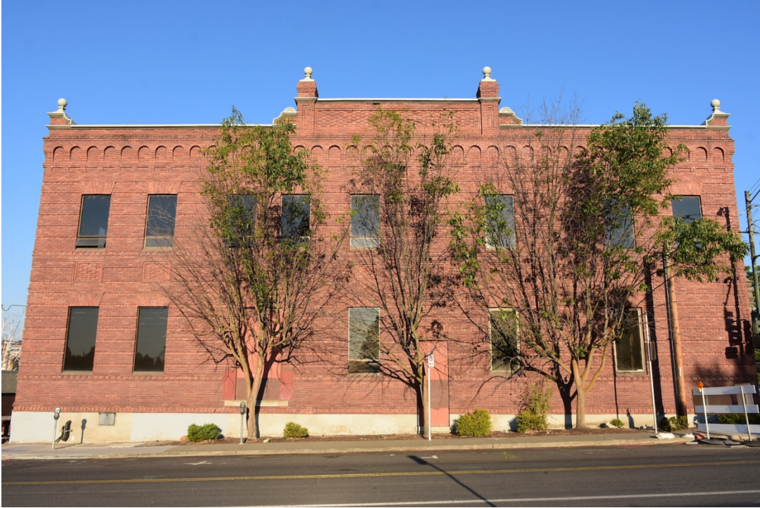
#5. East facade, looking west
