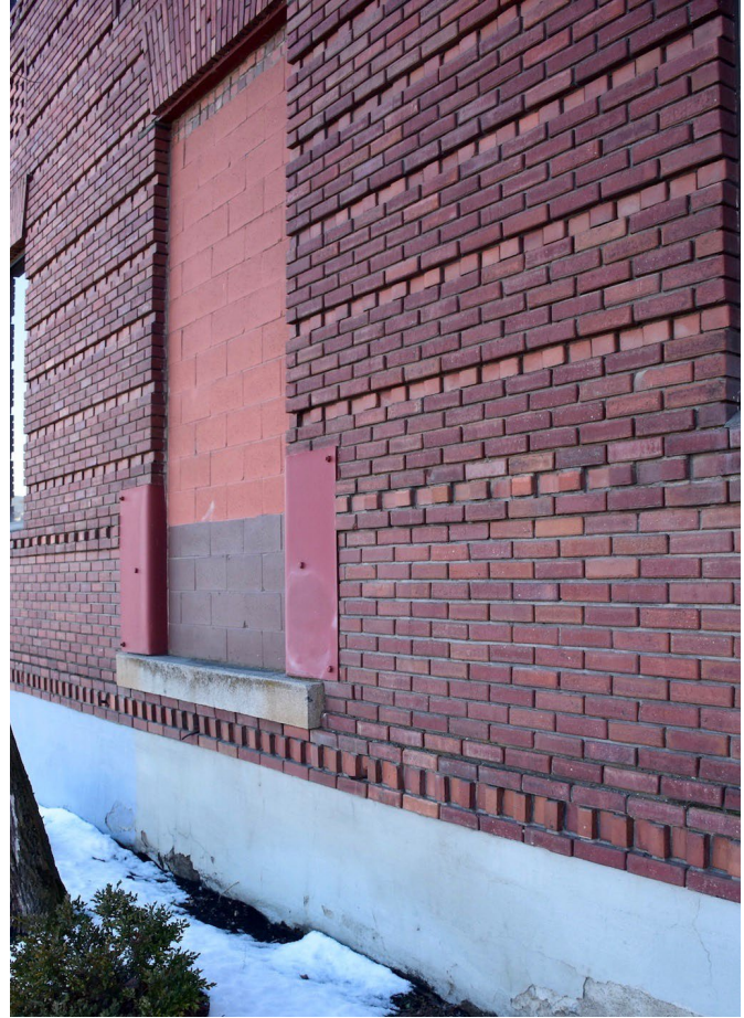
Figure 2: Detail of brickwork on the east elevation along Lincoln St.
