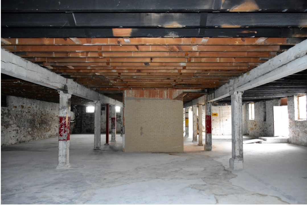
5. Basement, looking south from north wall
