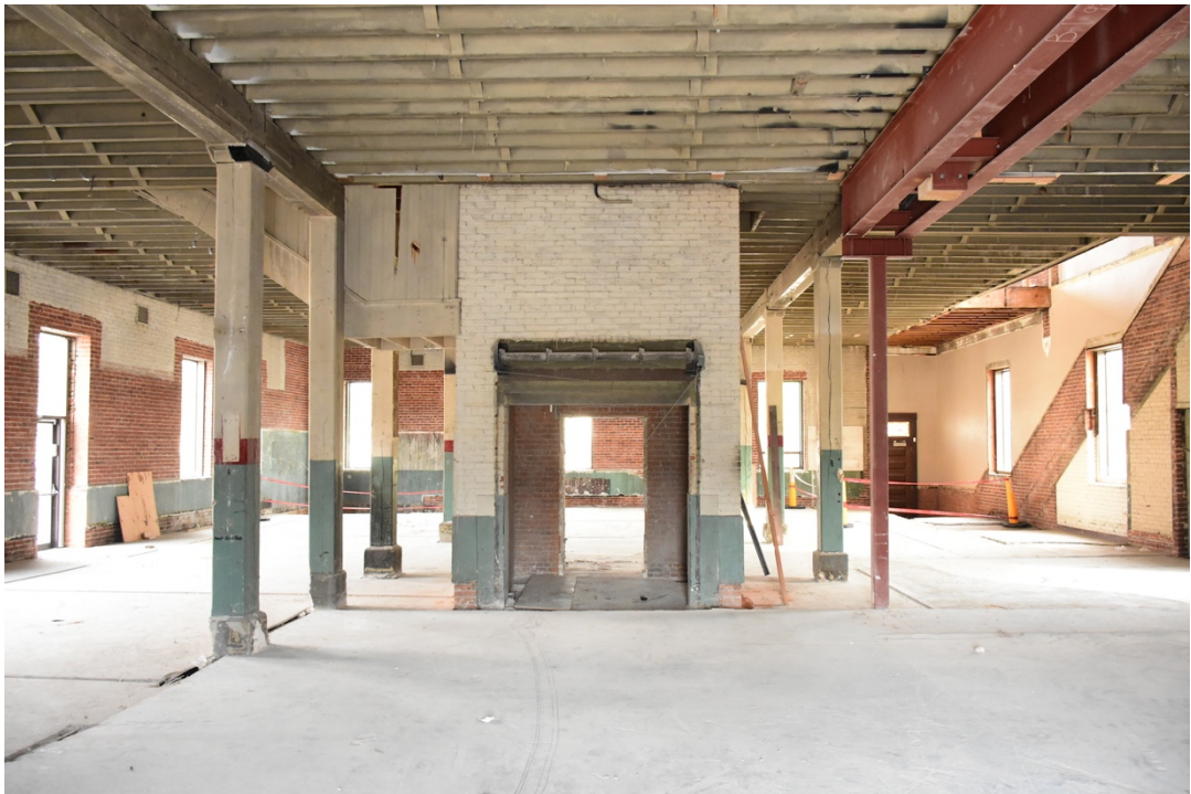
6. First floor, looking north from south wall
