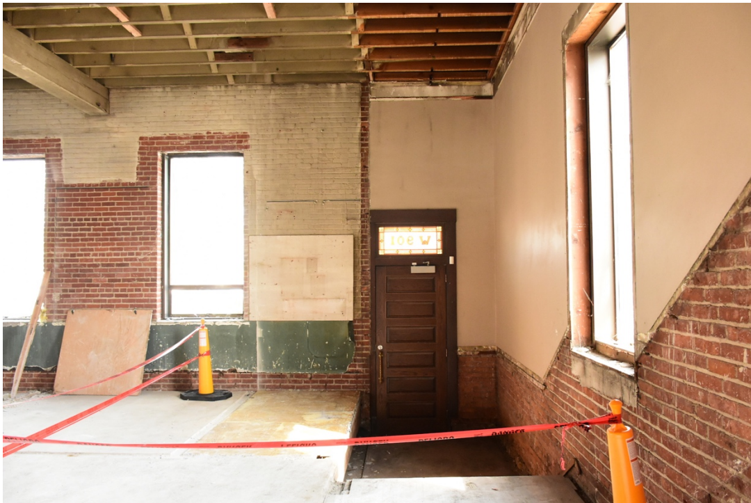
8. First floor, main entry in northeast corner, looking north
