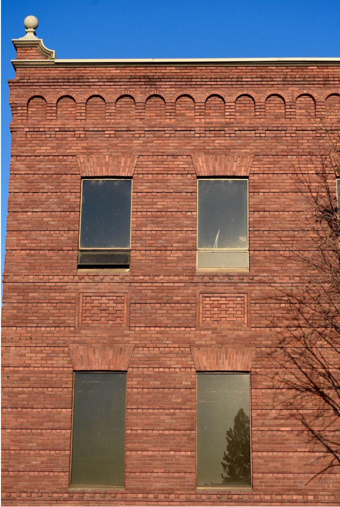
#11. Wall and parapet detail at southeast corner, looking west
