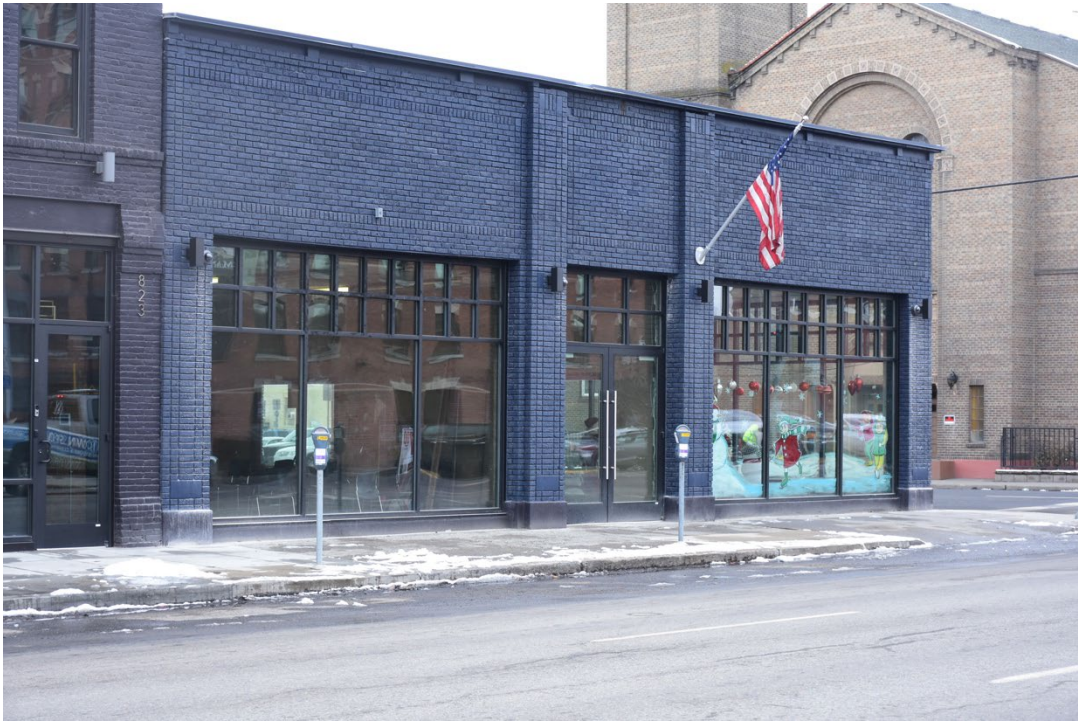
3. Northeast Corner - front facade, looking southwest
