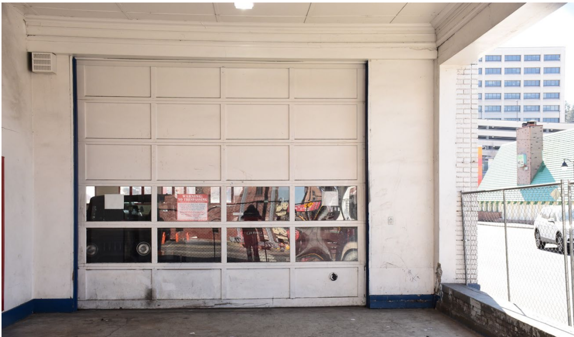
14. Looking south from reception and porte-cochere entry (enclosed as office space in 2022)
