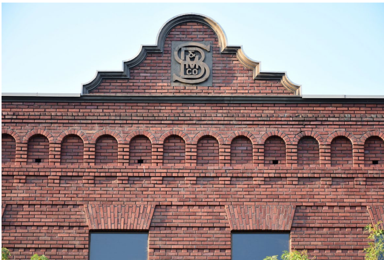
Figure 6: Central pediment detail, north elevation
