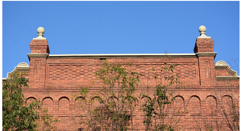
Figure 5: Parapet terminating east elevation
