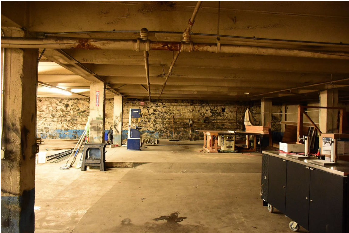
25. Basement, looking west
