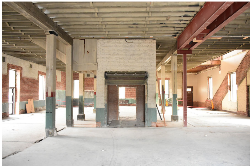
Figure 13: First floor looking north from south wall
