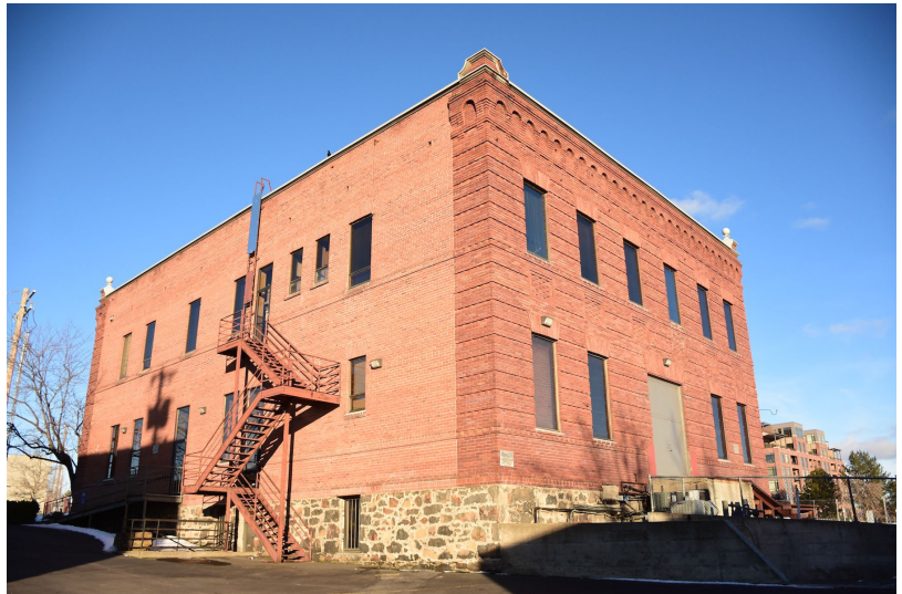
Figure 12: Southwest corner - south and west façades, looking northeast.
