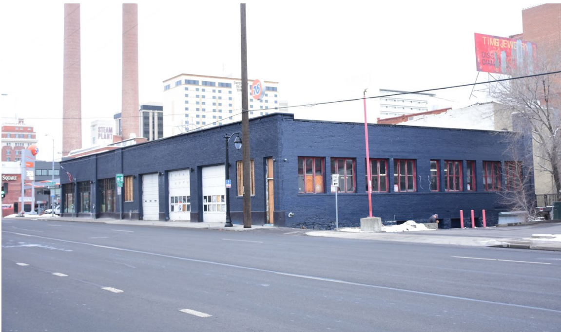
8. Southwest Corner - west and south facades, looking northeast
