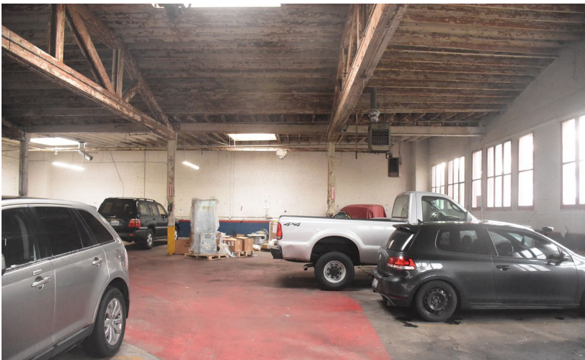
20. Garage, looking east along south wall
