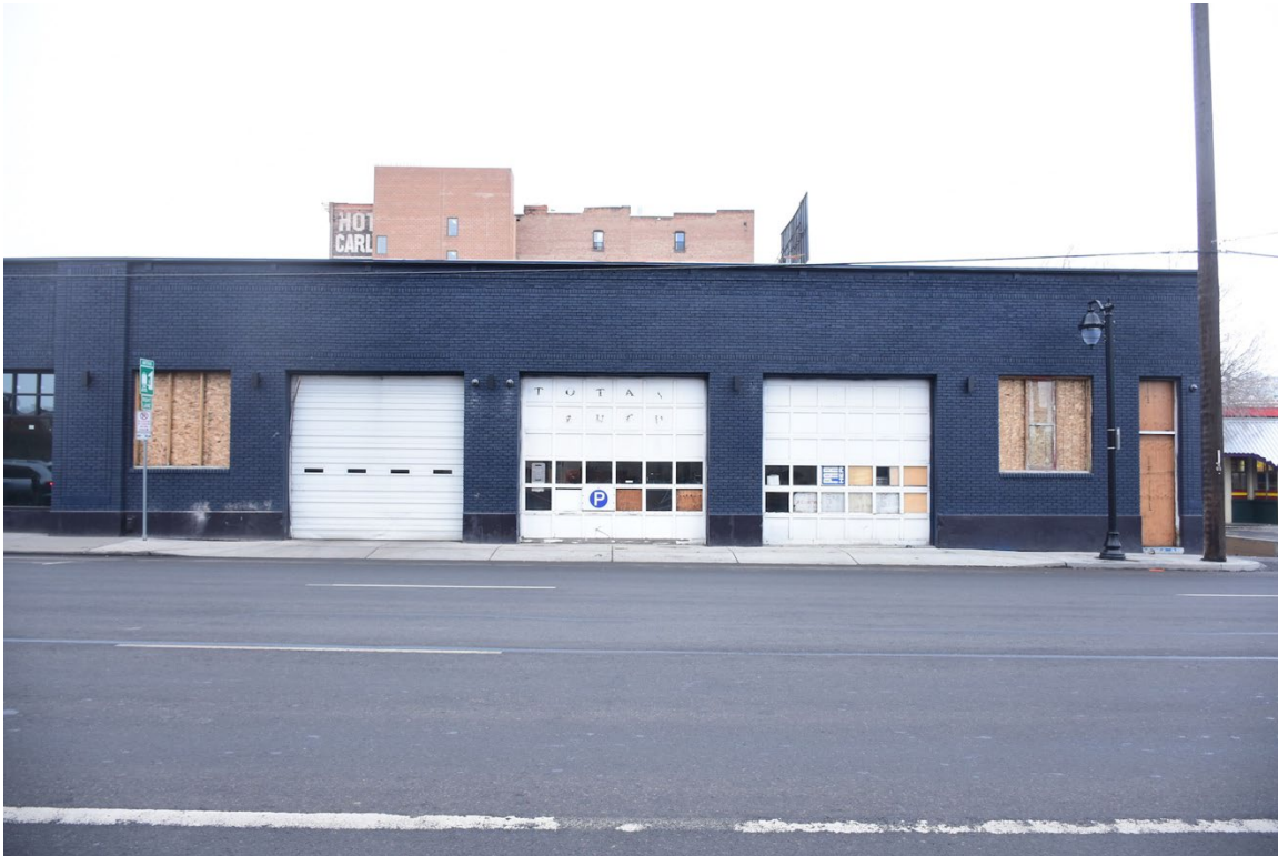
7. West Facade -south half, looking east.
