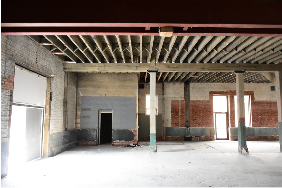
7. First floor, looking west at southwest corner
