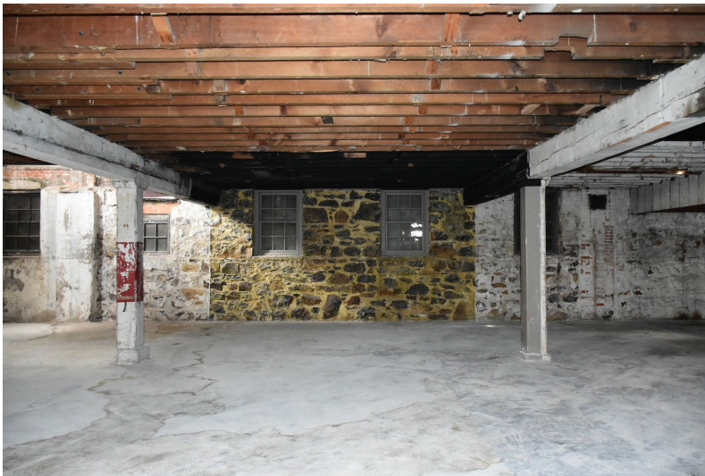
Figure 13: Basement looking north at the north wall – original daylight windows
