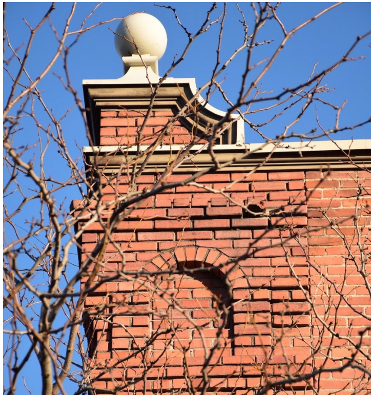
#10. Corner finial atop northwest corner, looking east
