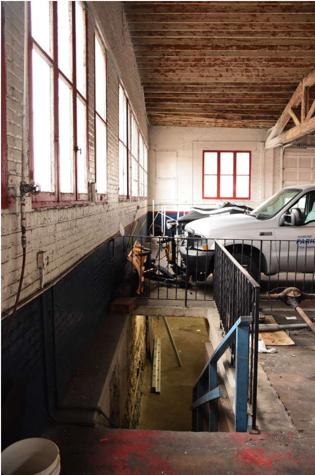
23. Garage, looking west along south wall showing stairs to basement
