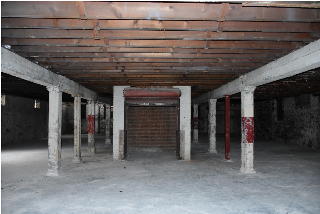
4. Basement - mid-section showing freight elevator, looking north
