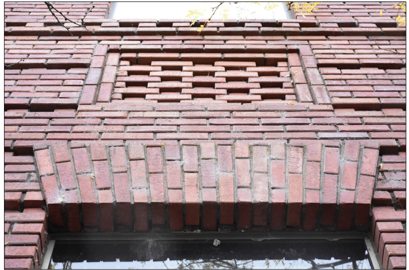
Figure 9: Window, brick detail
