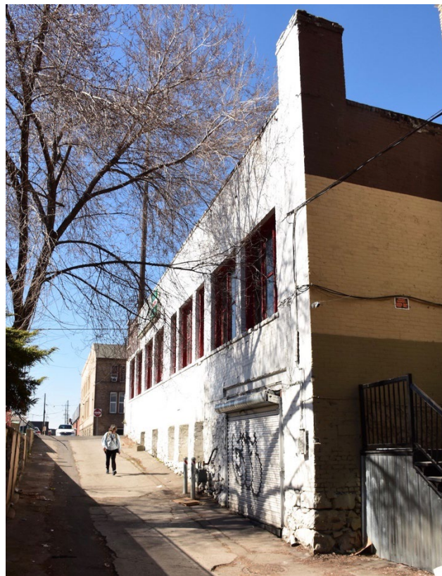
10. Southeast corner, looking west
