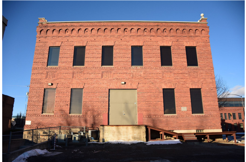
Figure 11: South (rear) elevation
