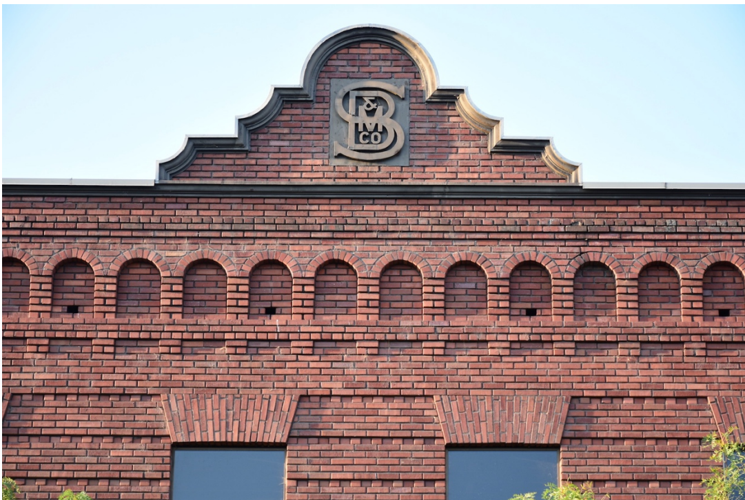
#8. Central pediment detail, looking south
