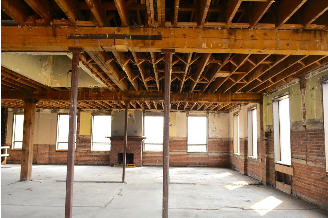
9. Second floor, looking east at southeast corner and fireplace
