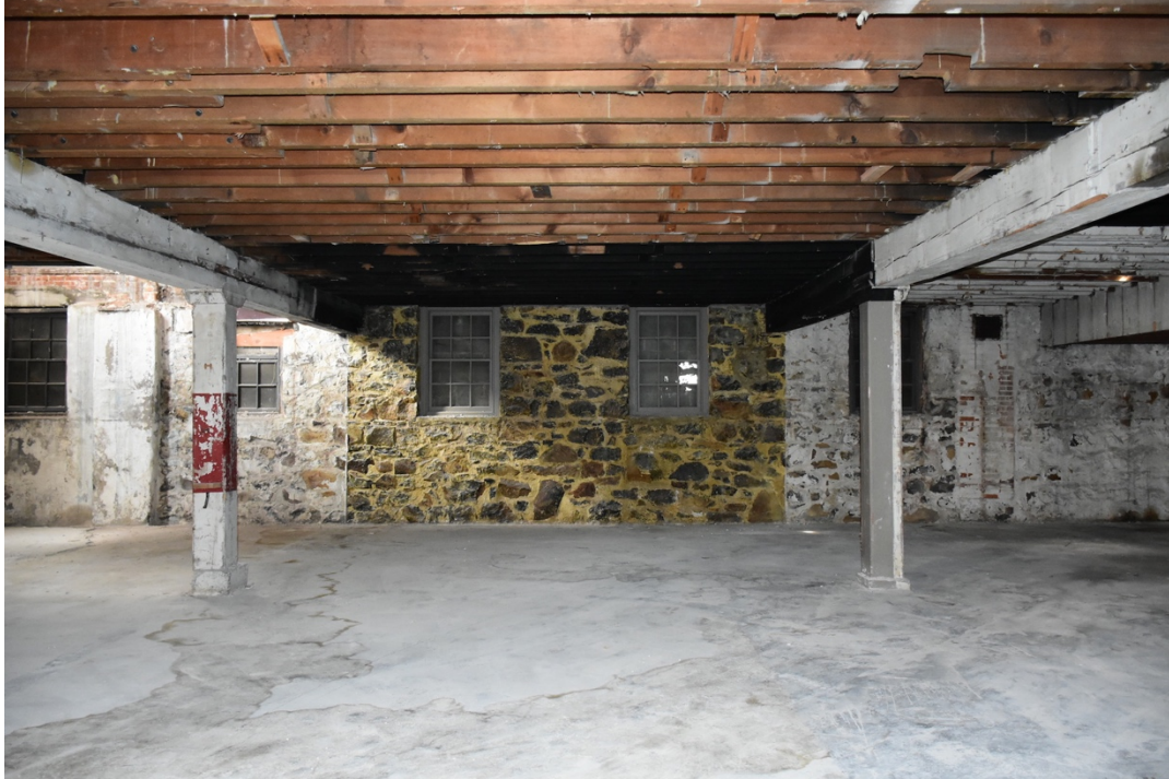
3. Basement - looking north at north wall - original daylight windows
