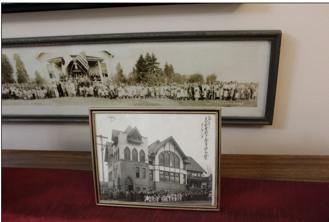
Photo 10: View of Grant Street Church, foreground, in vestibule display
