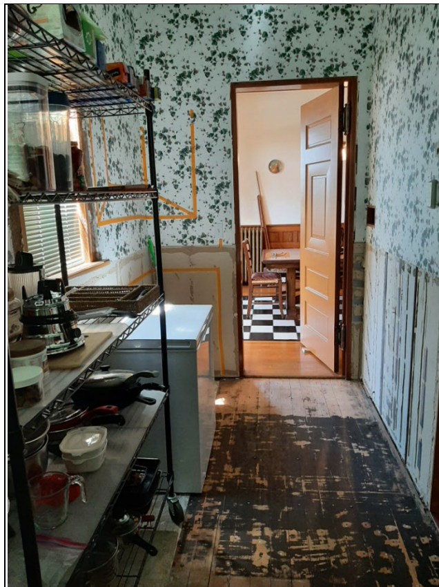
Photo 14—2021 photograph of the butler's pantry, looking north to the dining room
