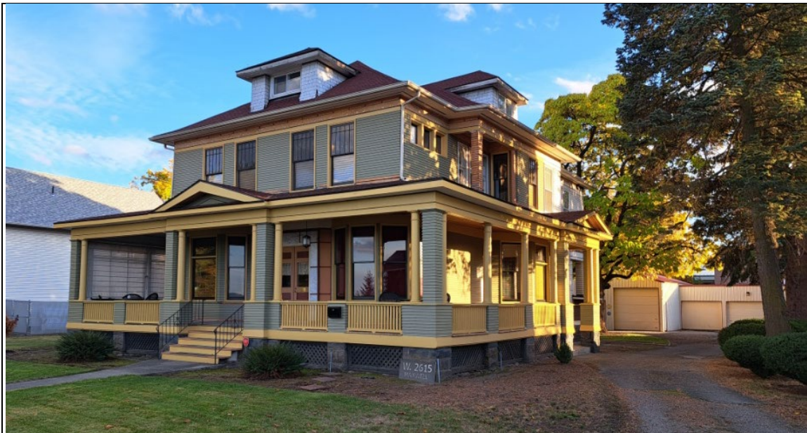
Photo 2 2022 photograph of the northwest façade corner of the Judge Blake House, looking south (notice 1980 garage/shop behind the house)
