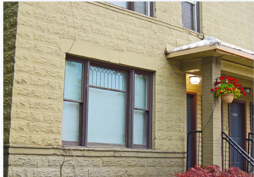
Windows at the small apartment building at 820 S Monroe are intact and include a decorative leaded glass transom.
