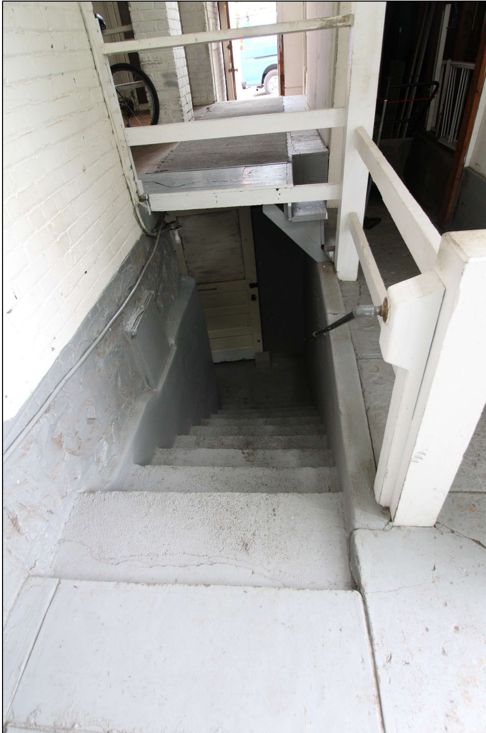
Photo 18: Stair to basement, north addition
