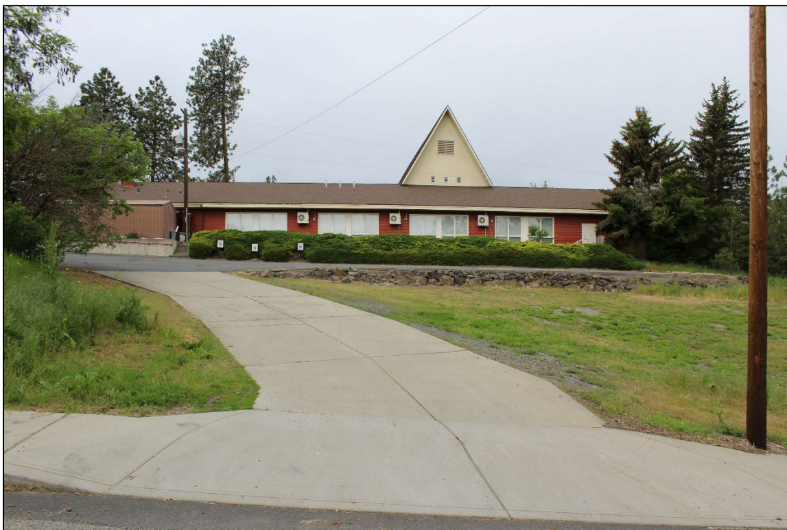
Photo 5: Rear view of Ellis Hall and Butler Chapel, looking west
