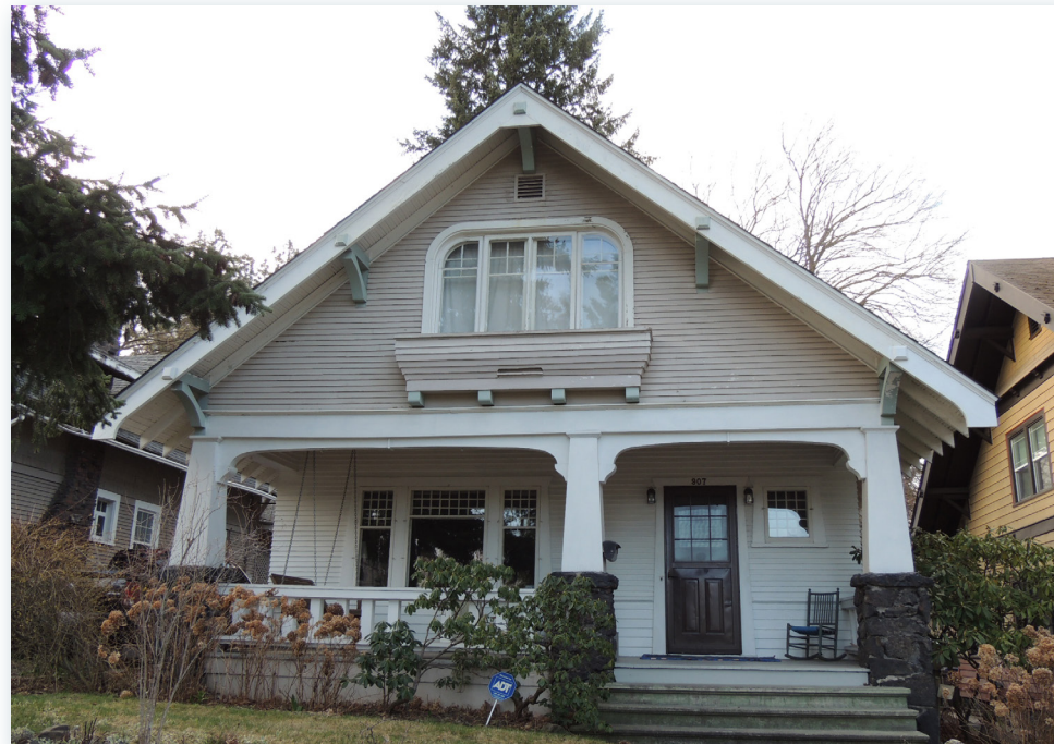
907 W Twelfth Avenue: Craftsman style columns and masonry foundation
