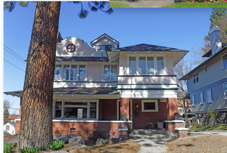
The house at 1128 W Eighth Avenue shows a hip roof, exposed eaves, and a mission style parapet.
