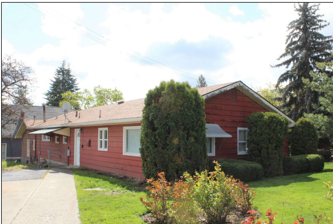
Photo 15: Parsonage, north (rear) and west facades, looking southeast
