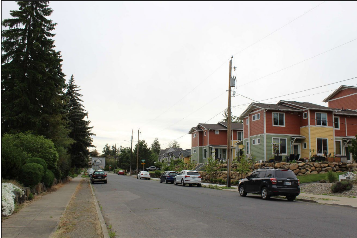
Photo 22: Setting – view toward east along E. Hartson Avenue
