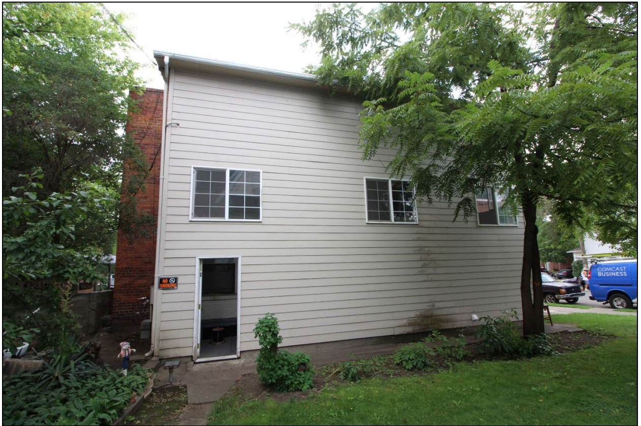
Photo 7: North façade, looking south
