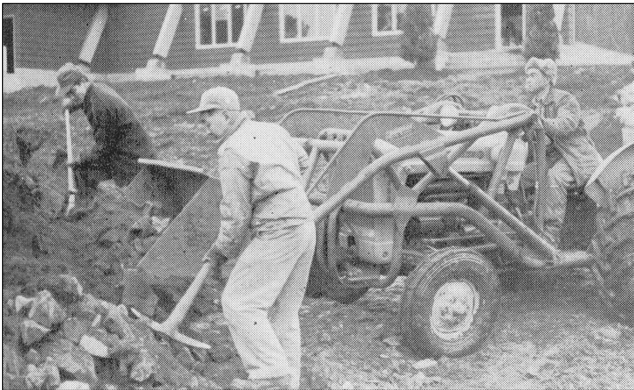
Figure 20: Garden construction underway, ca 1958
