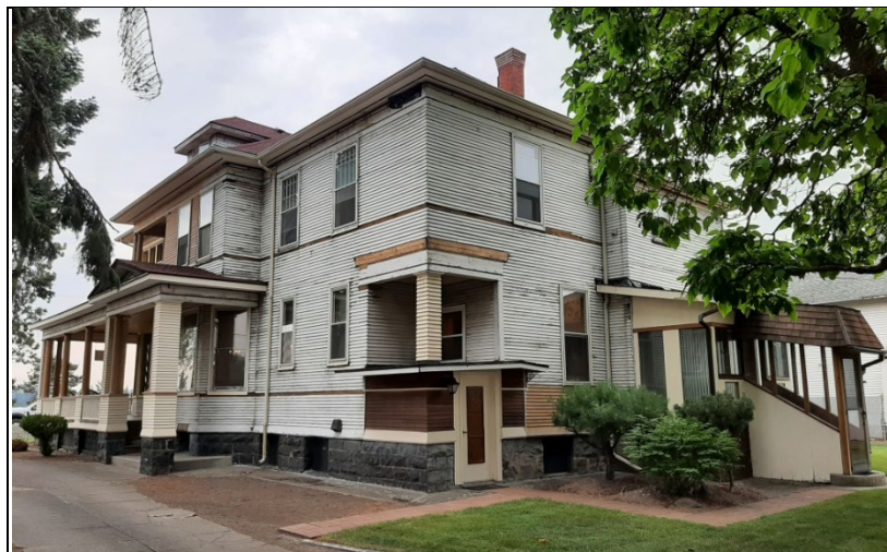
A 2022 photograph of the home's southwest rear corner, and south and west elevations
