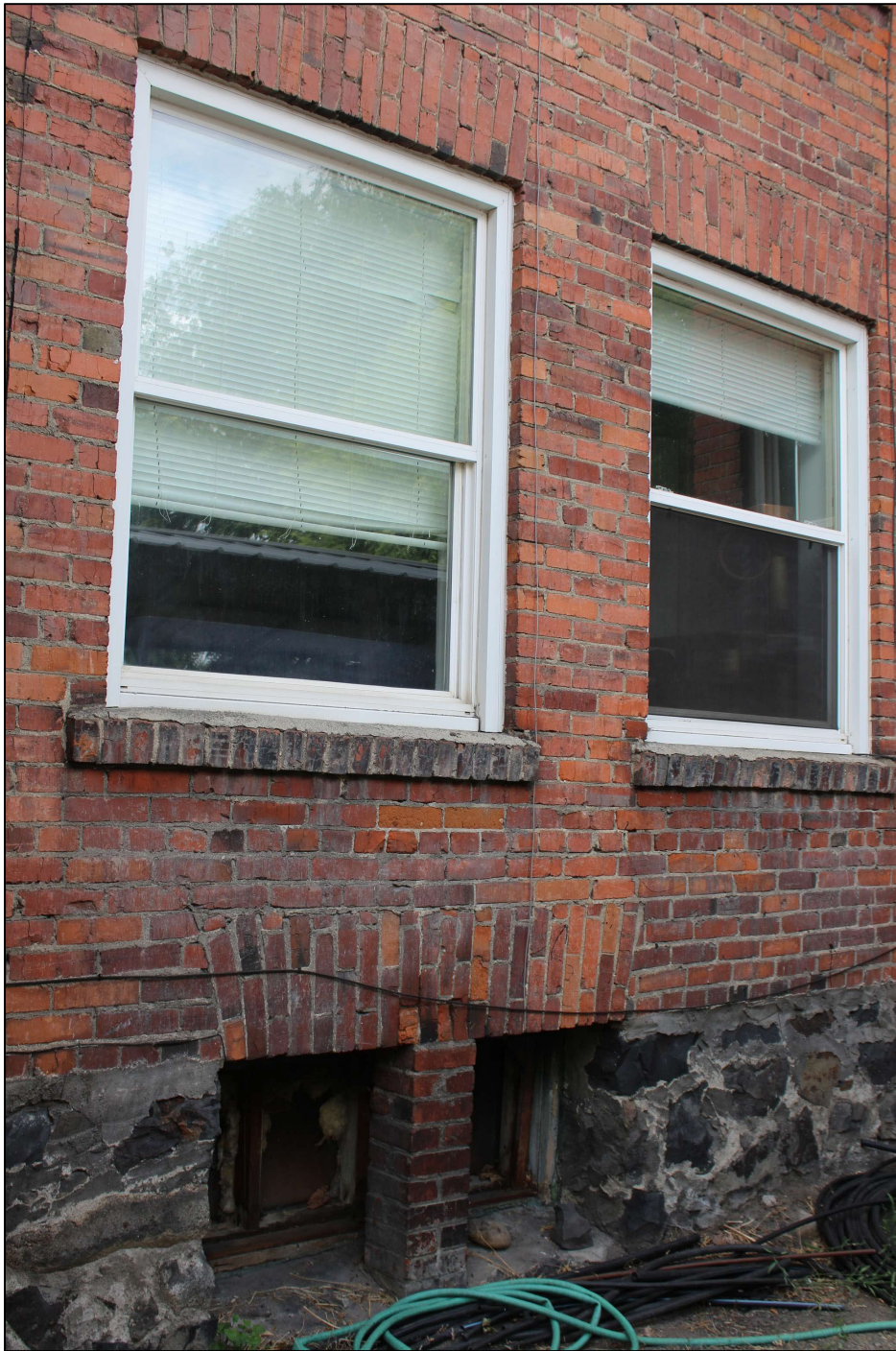
Photo 11: Typical windows, east façade
