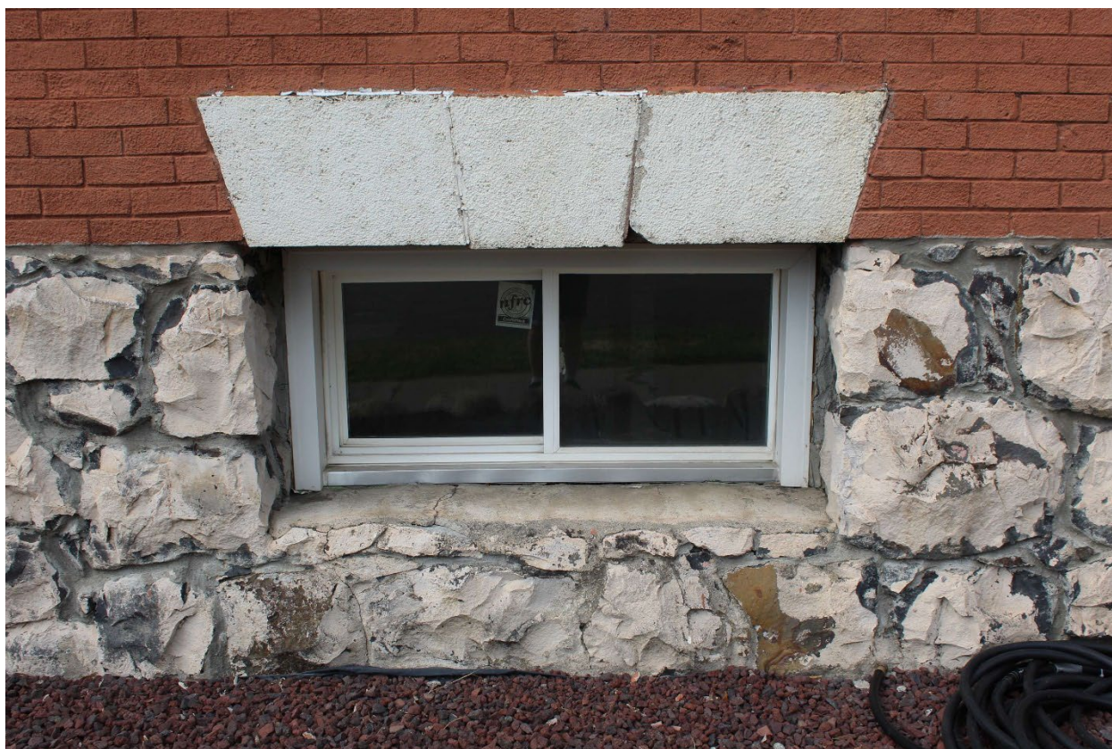
Photo 10: Basement window, typical
