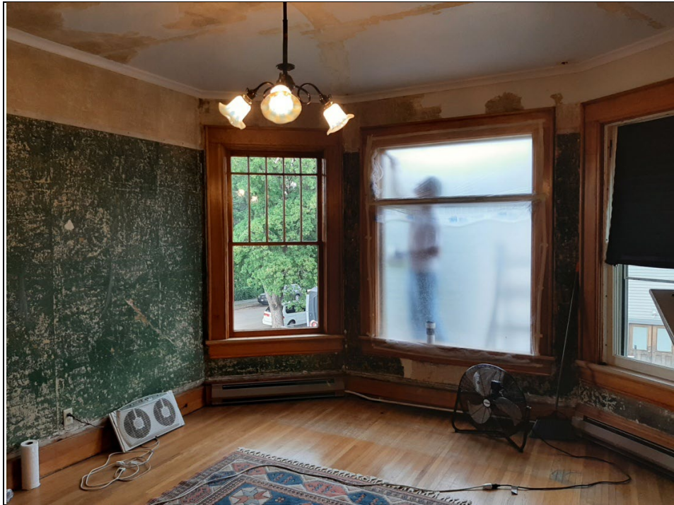
Photo 19 2022 photograph of the center east wall bedroom on the second floor
