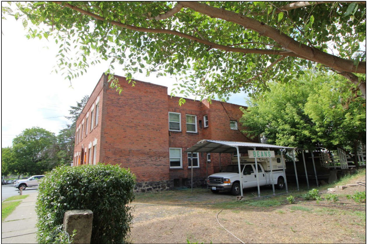
Photo 6: East façade, looking west
