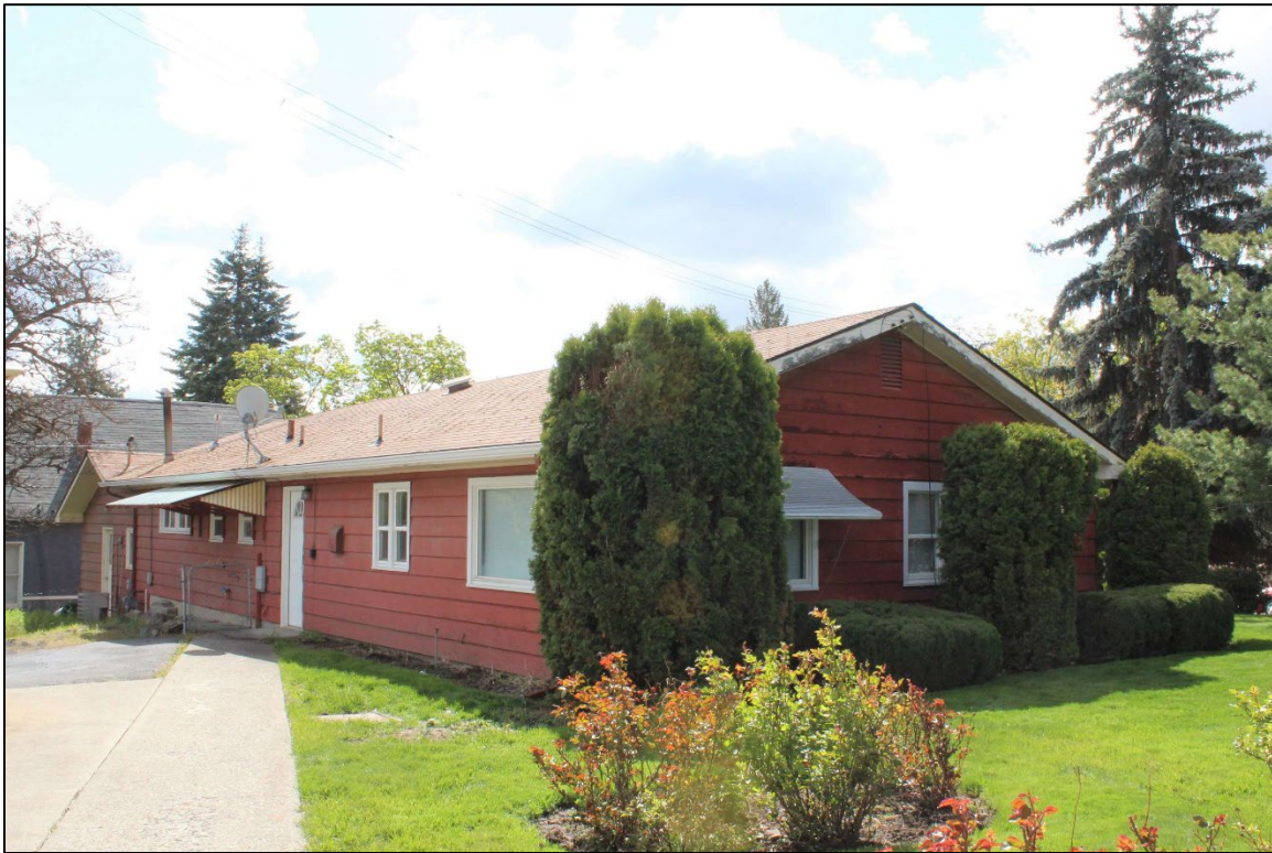
Parsonage, north (rear) and west façade, looking southeast
