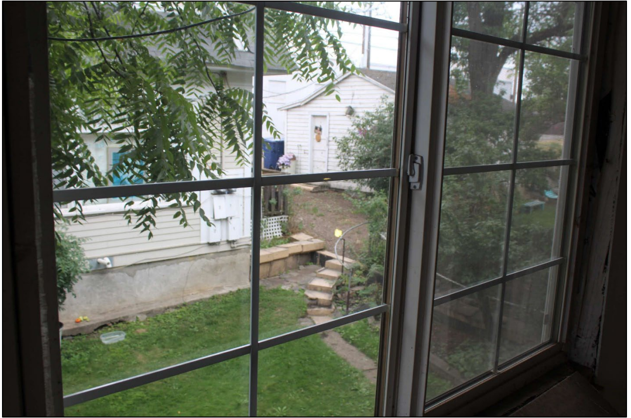
Photo 17: Looking toward back yard from north addition
