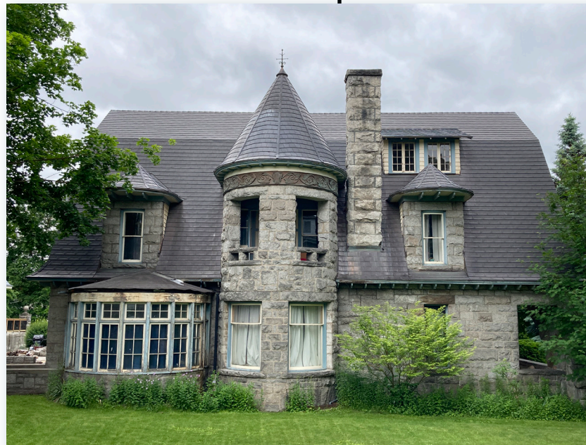
The house at 1323 W Eighth Avenue: the house is capped with a complex roof composed of a gambrel roof with tower, hipped and shed dormer roofs.
