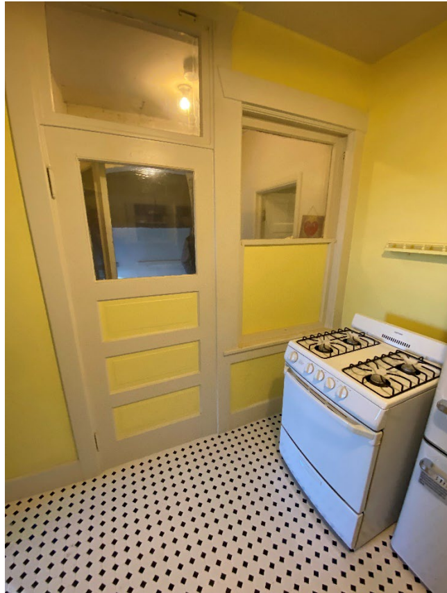
Kitchen in a rear studio apartment showing former entry door which remains, but is inoperable.
