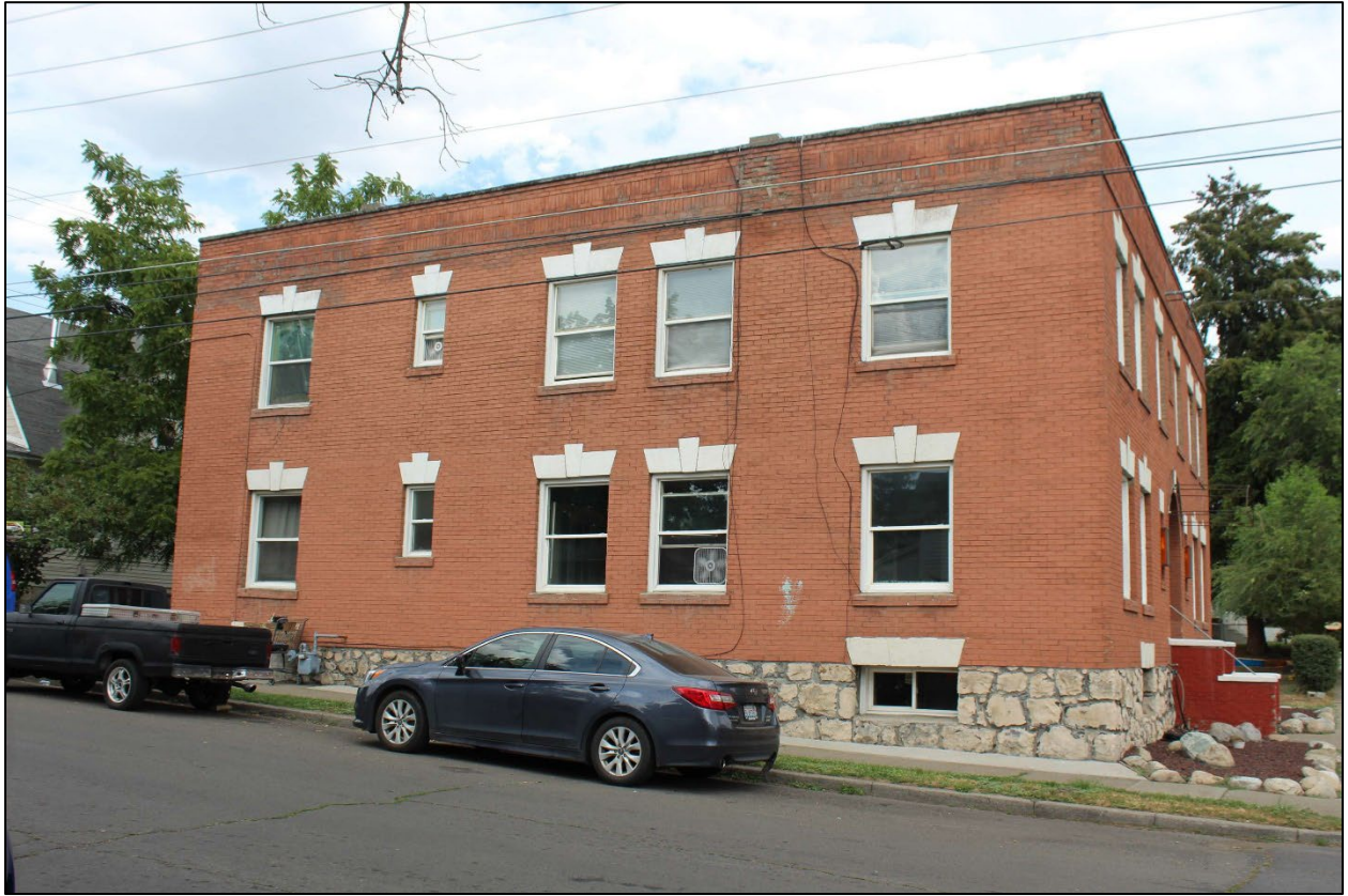
Photo 9: West façade, looking east
