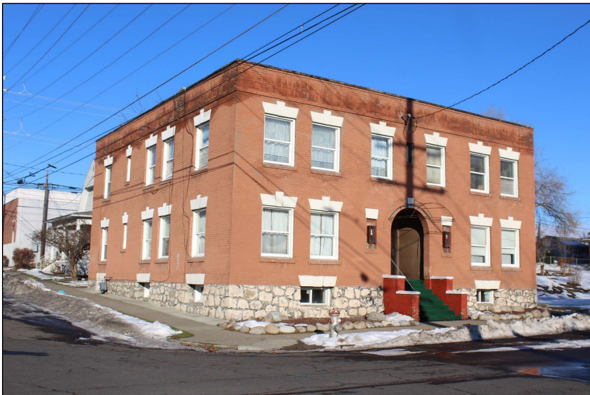
West and south facades, looking northeast
