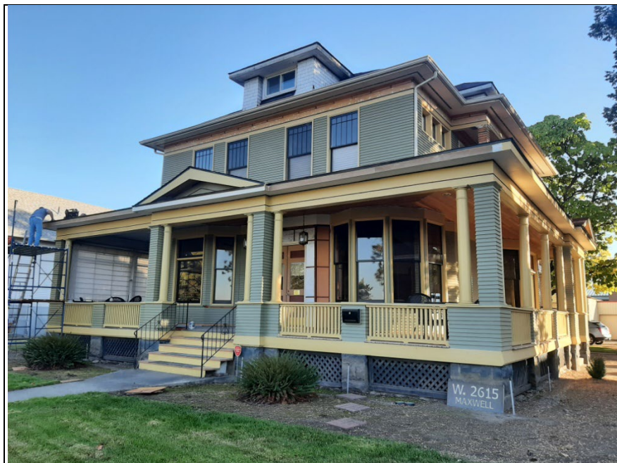
A 2022 photograph of the northwest corner of the house, looking south
