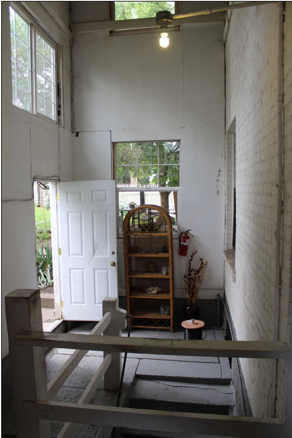
Photo 16: First floor, north addition, looking east
