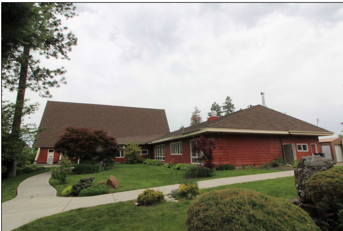
Photo 4: Butler Chapel (left), Ellis Hall (right), looking north
