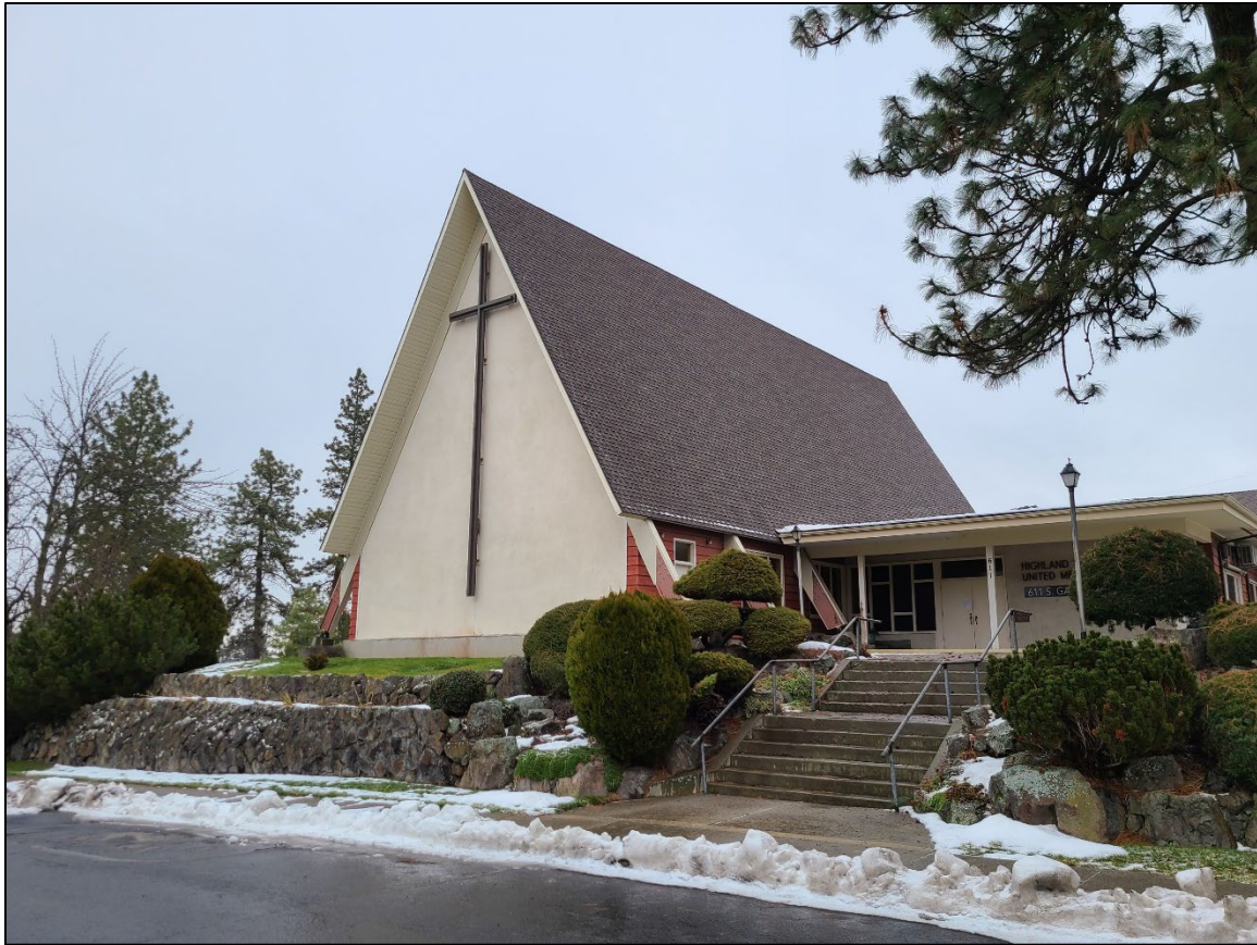
Butler Chapel (Sanctuary), front (west) façade
