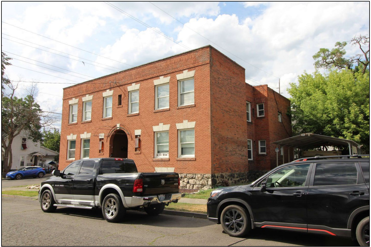
Photo 5: South and east facades, looking northwest
