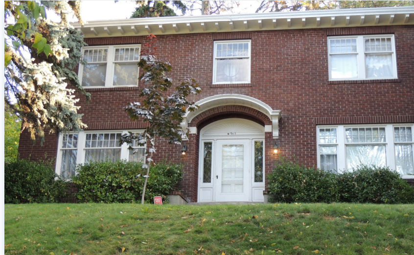
The Italian Renaissance style apartment building at 2306 W Pacific Avenue stands three stories tall in a rectangular plan that is capped with a flat roof edged with parapets exhibiting a dentilated cornice
