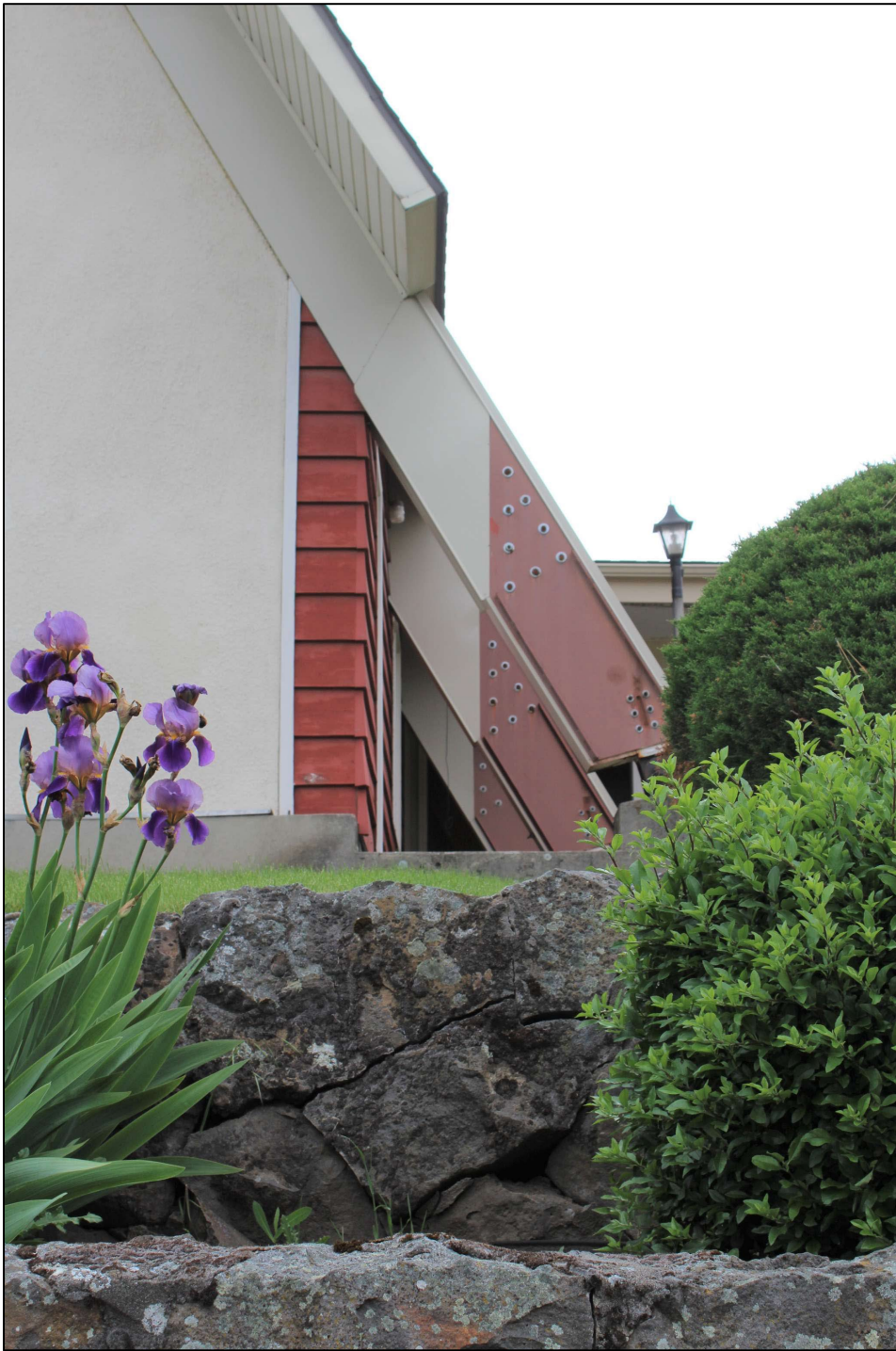
Photo 3: Beams touching down on south side of sanctuary
