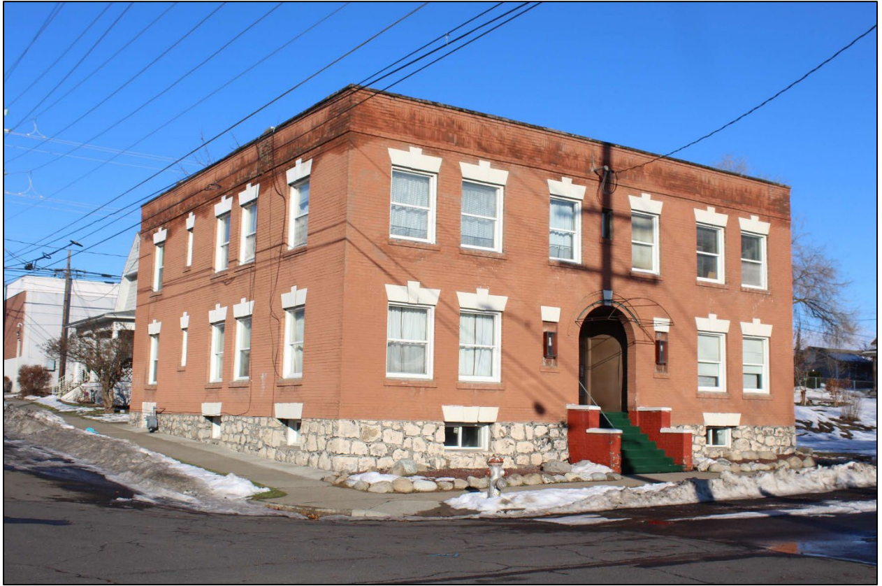
Photo 1: West and south (front) facades, looking northeast
