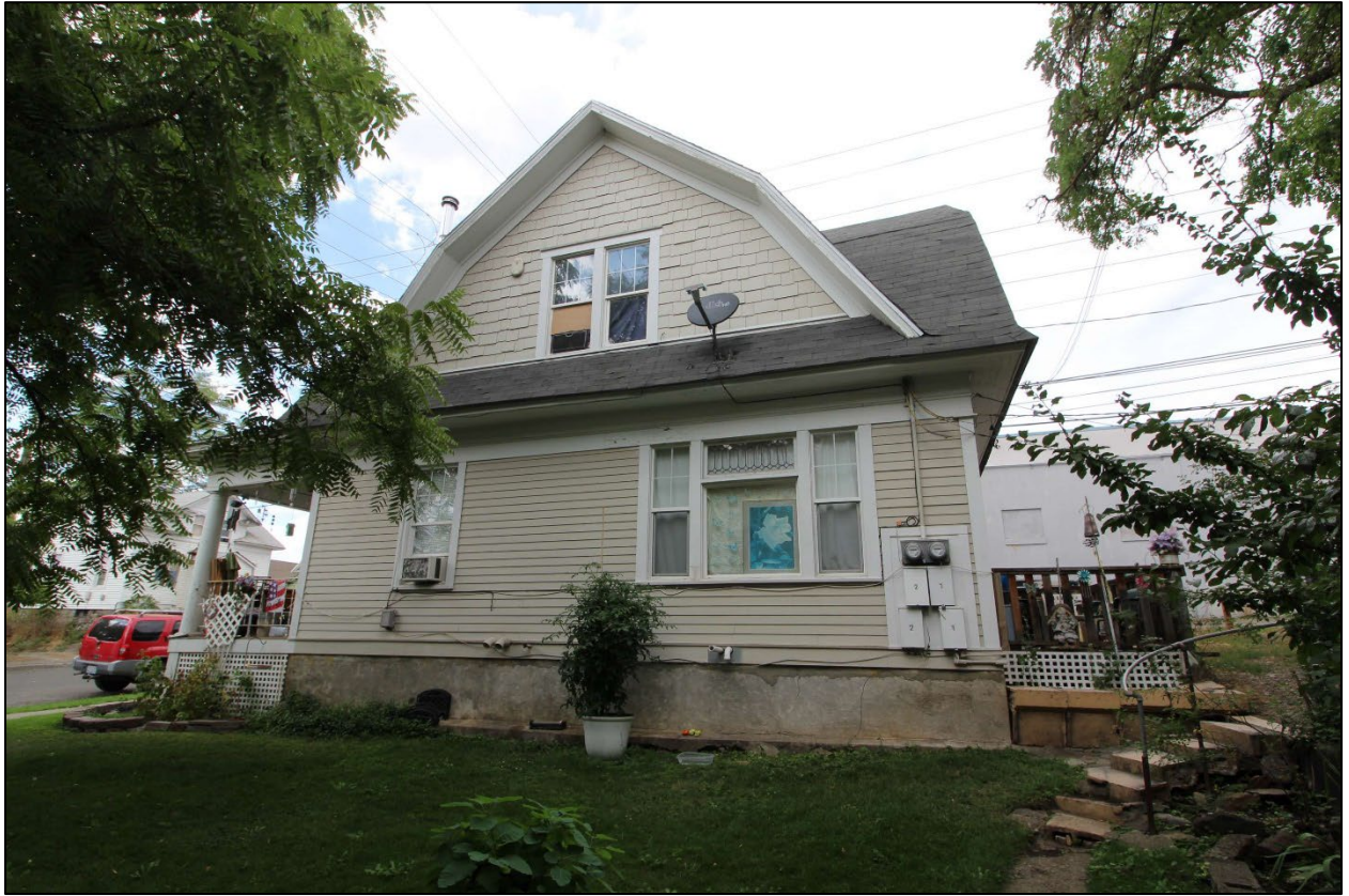
Photo 23: Duplex north of apartment building
