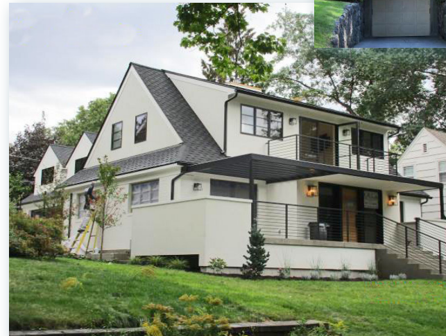
The house at 1925 S. Stevens is a 2018 remodel of 1940 house (above is the before). It is an example of invention within a side-gabled house with addition of a larger porch and second-story deck and additions to the rear.
