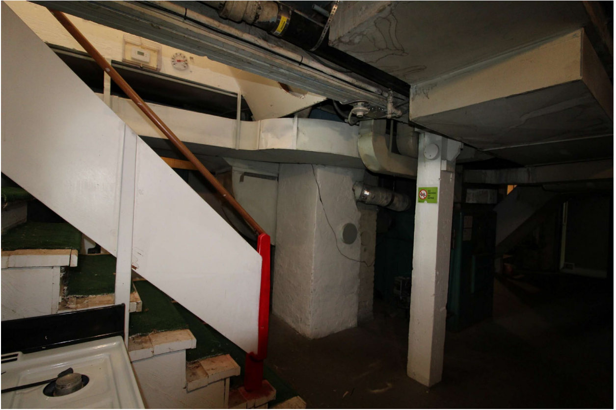
Photo 15: Basement, stair to left, furnace to right
