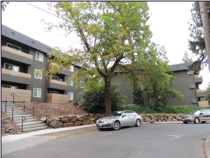
Left: The apartments at 815 S Lincoln are a contemporary addition to the district.
