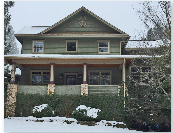
The house at 1826 E Pinecrest is an example of replication of a traditional Early-20th Century house with a porch.
