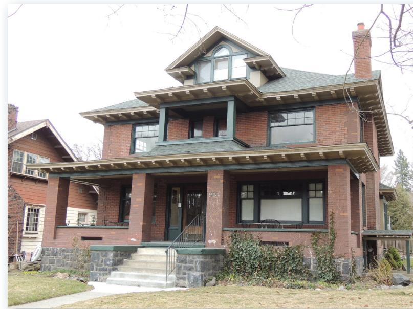
2927 S Adams Street: The full-width front porch is constructed with masonry columns and solid brick walls with drainage openings.
