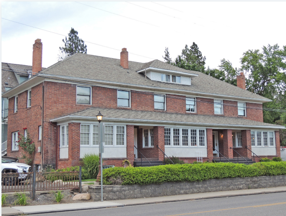
The apartment building at 823 S Monroe appears to have had open porches enclosed quite some time ago as is evidenced by the wood 6:9 paned windows.
