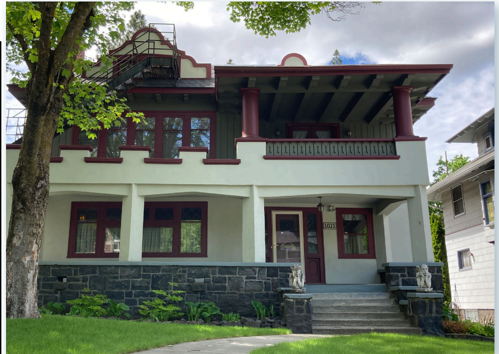
1021 W 8th - This home includes deep eaves, columns, stucco, vertical wood siding, unusual wood baluster details on the balcony, parapets and cut basalt foundation.
