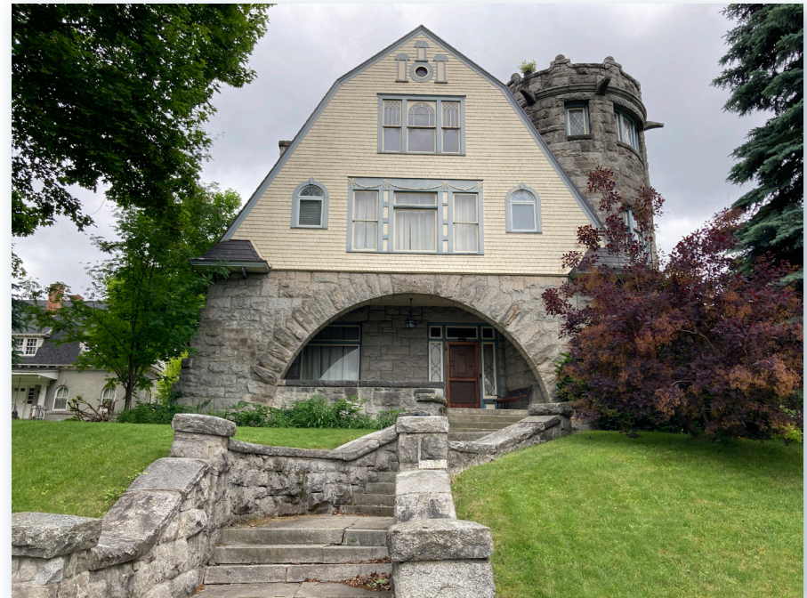
Above: The home at 1323 W Eighth includes impressive hardscaping that ties directly into the design of the house with cut stone lining the walkway.
