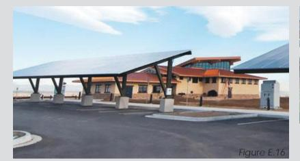
Solar panels built into shade structures, charging for electric vehicles, rain gardens to capture surface runoff, and permeable paving are all excellent ways to fascilitate sustainable parking.
