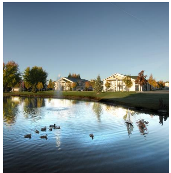
Adirondack Lodge Stormwater Facility (2007)
