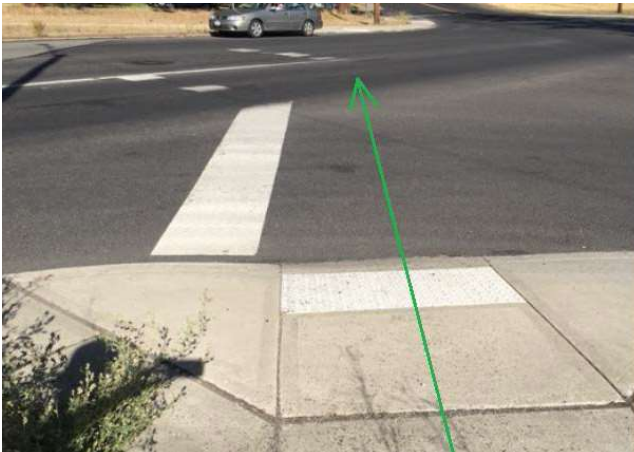
Figure 6 – Ramp running slope aligned with direction of pedestrian travel and ramp on opposite corner
