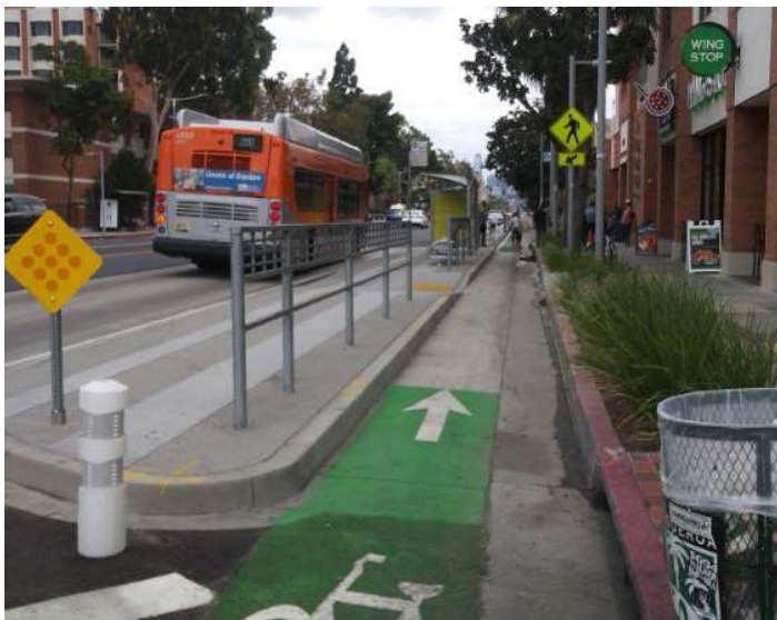
Figure 9 – Island bus stop separates bike lane from bus traffic
