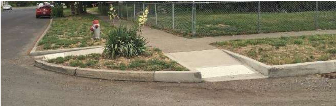
Figure 8 – Dual ramps with curbs instead of flares
