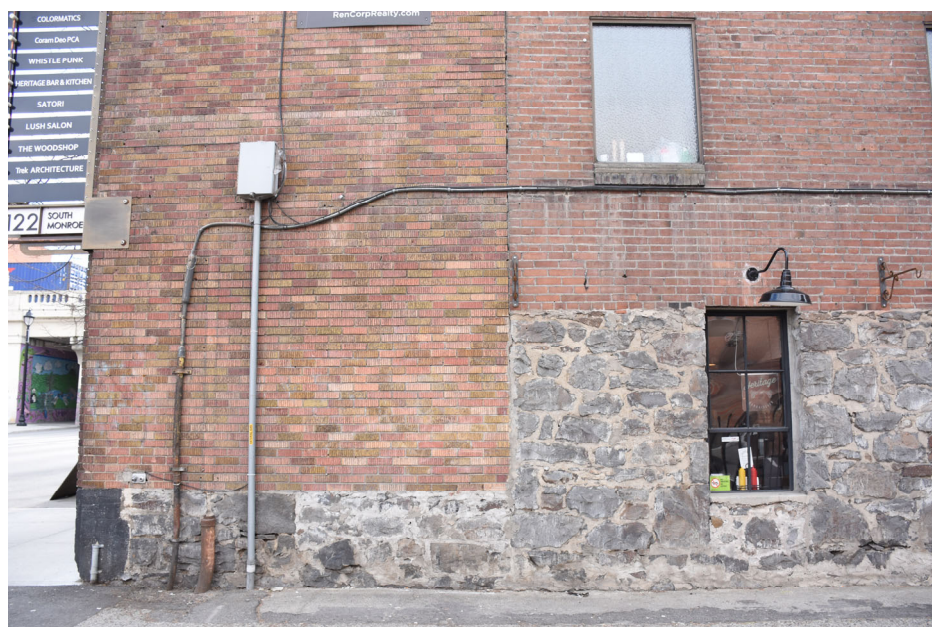
9. North facade-northeast corner showing wall juncture (1928 & 1910)
