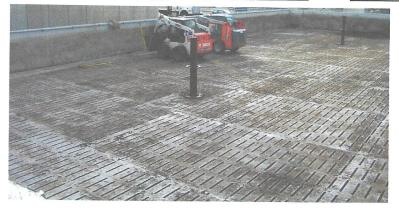
2) Geonet Mesh: Vendor must provide new goenet, thickness 200 – 250 mil. It is estimated that 5,720 square feet would be required.
