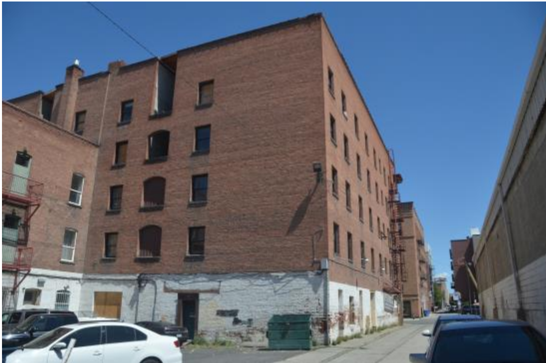
5. Southwest Corner, West Rear and South Alley Facades, Looking Northeast
