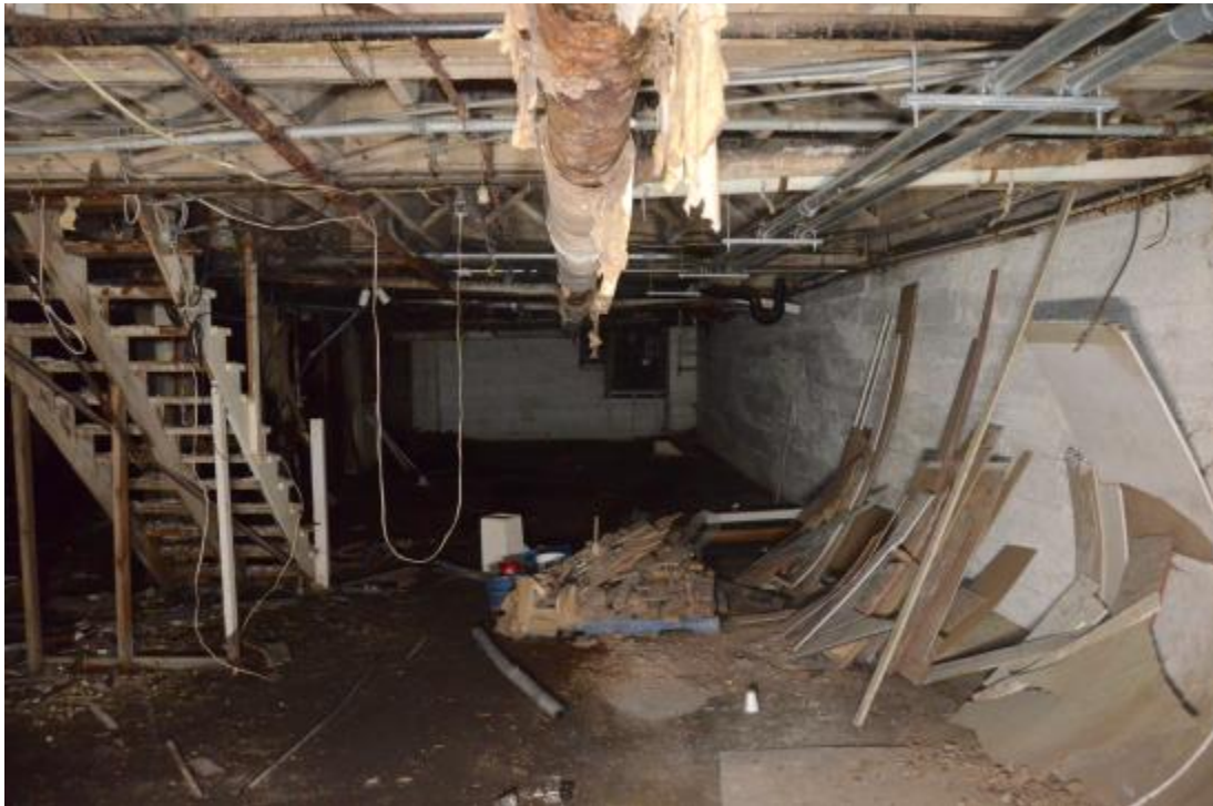
11. Basement, Looking North Along East Wall
