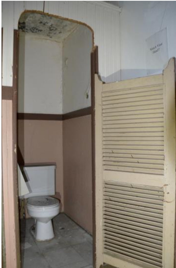
22. Common Restroom Showing Toilet Stall
