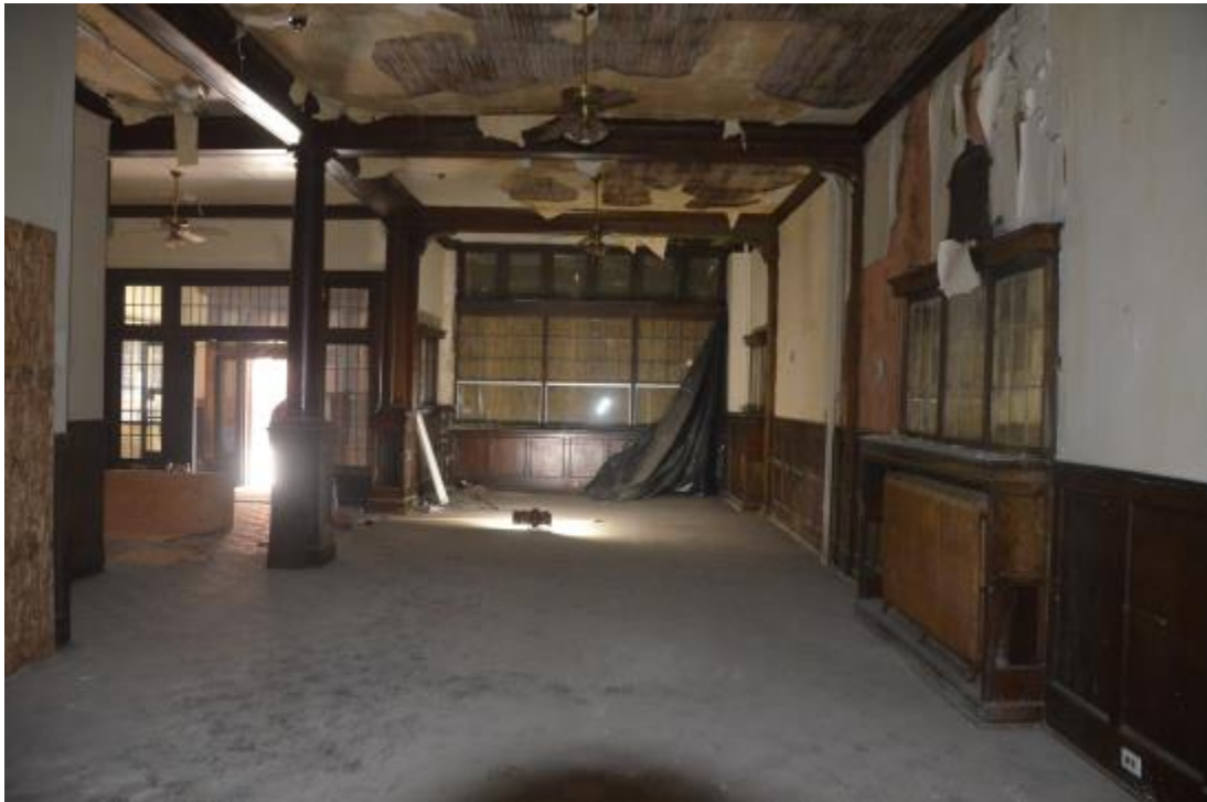
3. Lobby, Looking East Toward Main Entry
