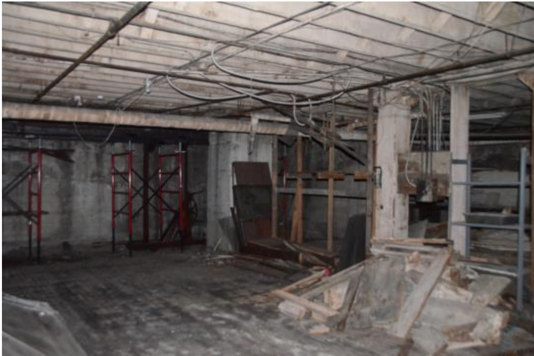
13. Basement, South Section, Looking Southeast Toward Sidewalk Vault Scaffold
