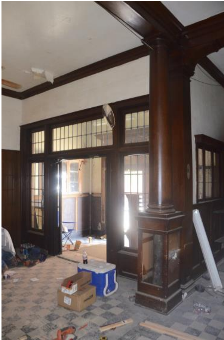
2. Lobby, Looking Northeast Toward Entry Vestibule
