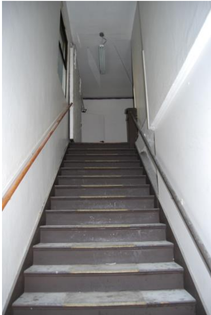
23. Central Stairway Between 4th & 5th Floors
