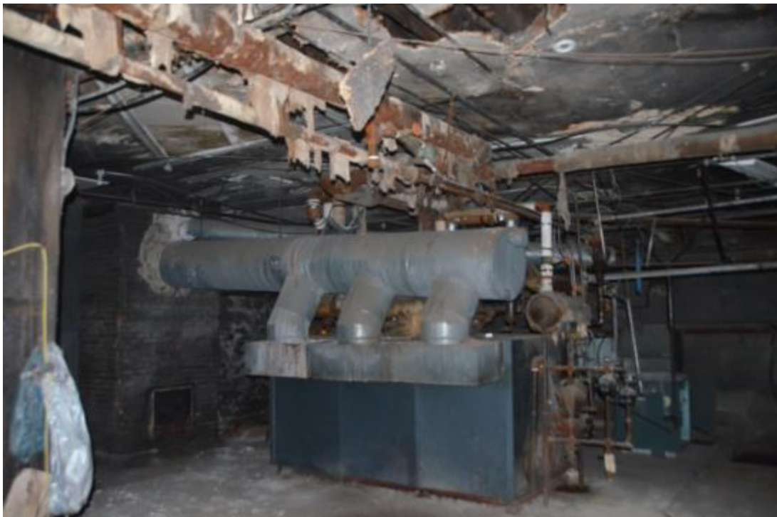
14. Basement, South Section, Looking Northwest Toward Boiler Room
