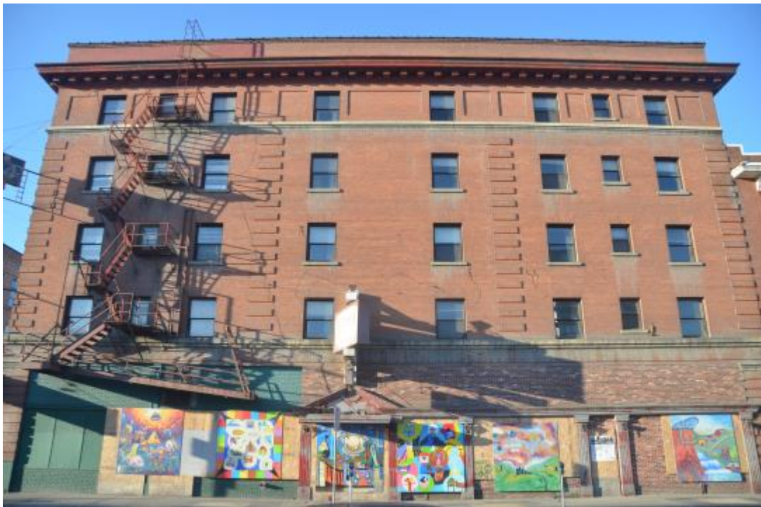
2. North-Front Facade Along First Avenue, Looking South
