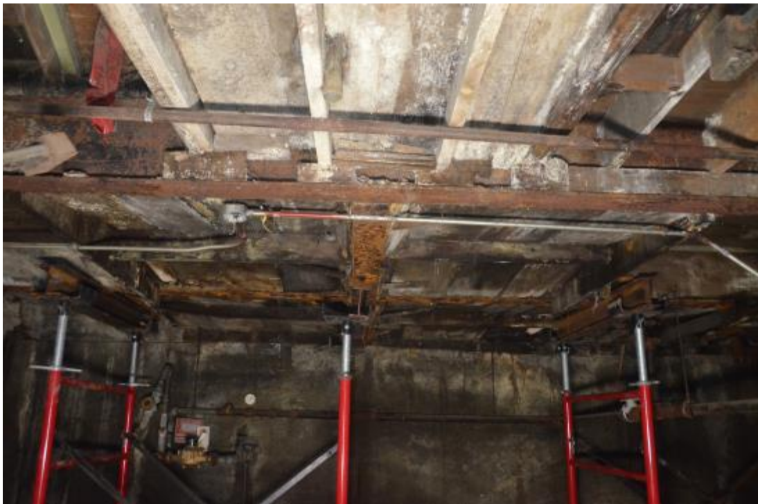
12. Basement - Supporting the Sidewalk, North Side
