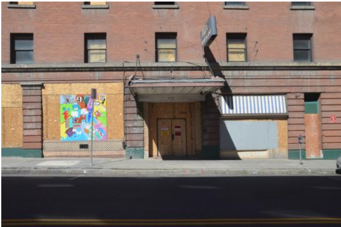
6. East Facade Hotel Entry & Lobby Front and North Side Commercial Bay
