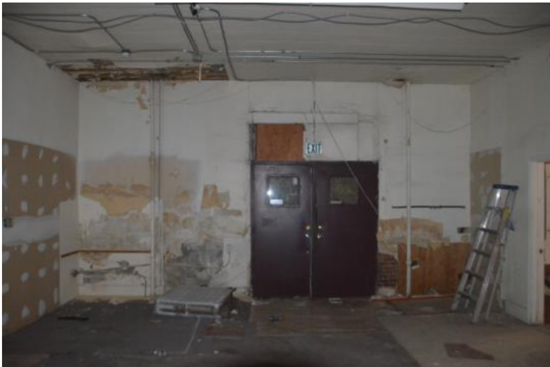
10. First Floor-South Commercial Bays, Looking South at Exit to Alley
