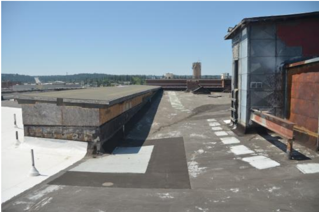
9. Penthouse and Shed Covering South Skylight Well, Looking West
