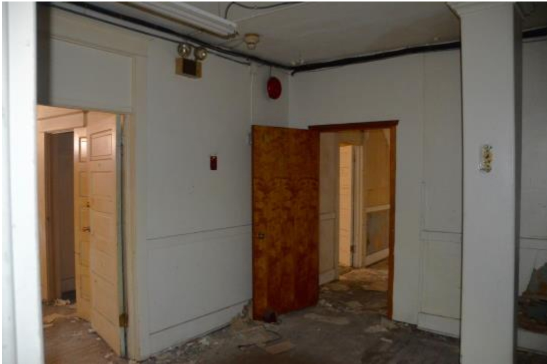
16. 2nd Floor Stair/Elevator Vestibule, Looking Southeast
