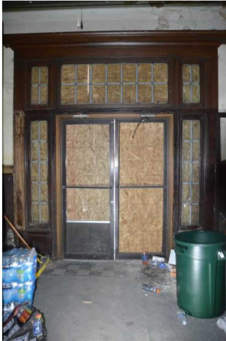
1. Lobby Vestibule-Inside of Main Entry Bay, Looking East Toward Madison Street
