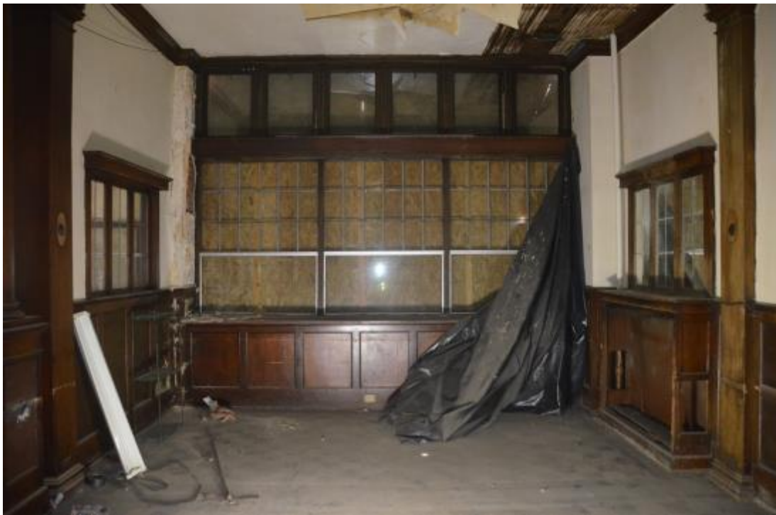
4. Lobby, East End, Looking East
