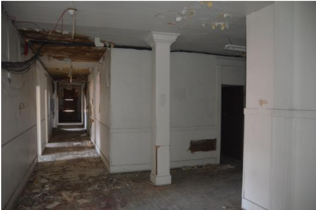
24. 5th Floor-Stair/Elevator Lobby, Looking South
