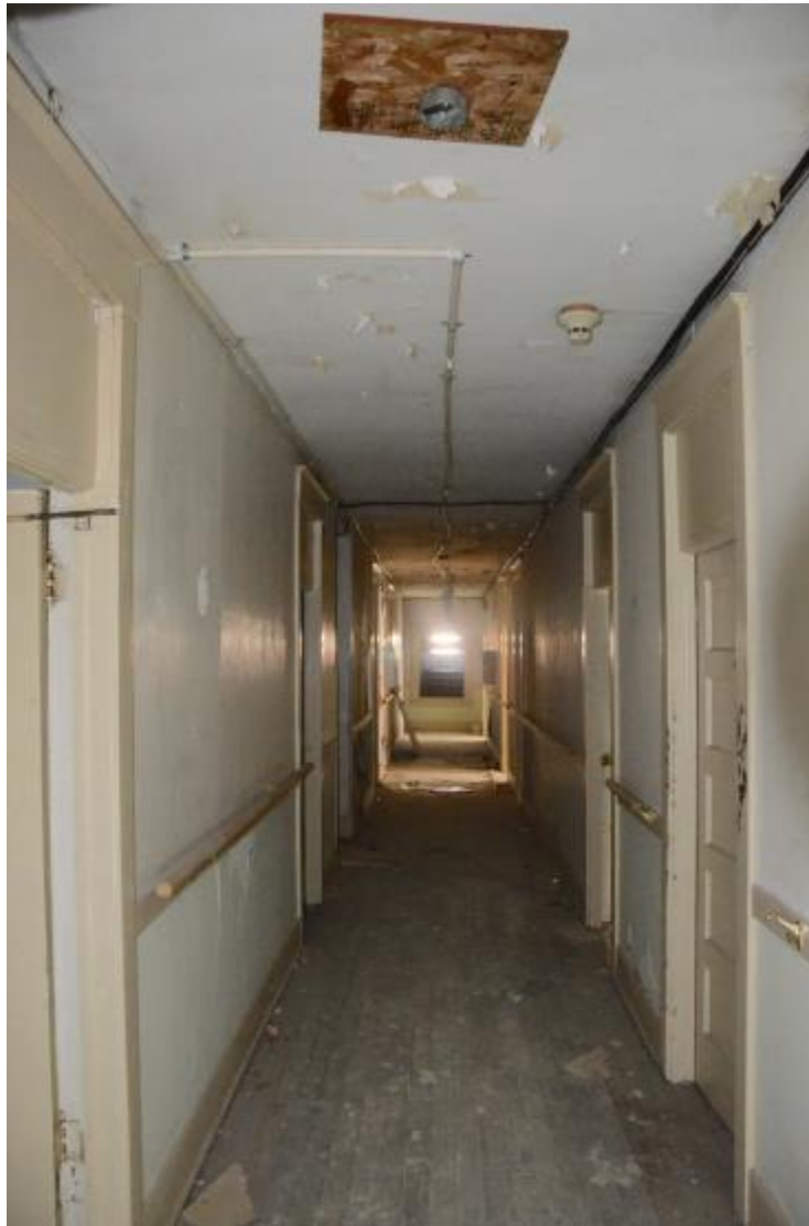
18. 2nd Floor, North-South Front Hallway, Looking North From Stair/Elevator Vestibule
