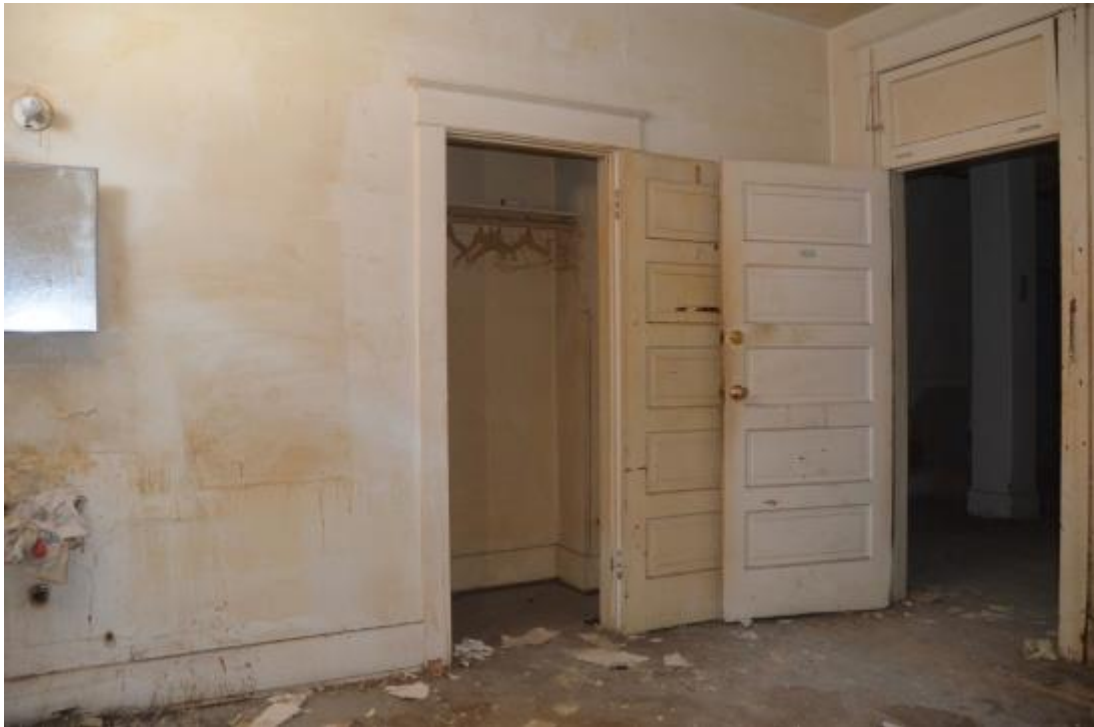
19. 2nd Floor, Typical Room on East Side
