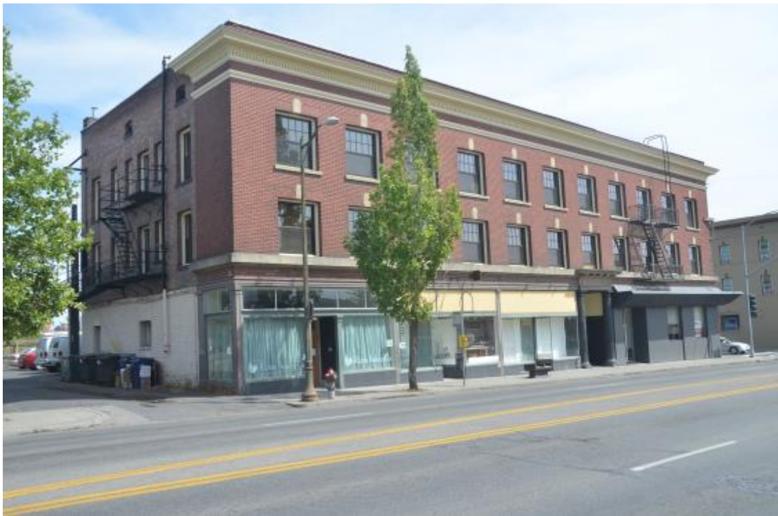
4. NE corner of building, north and west facades, view to the SE
