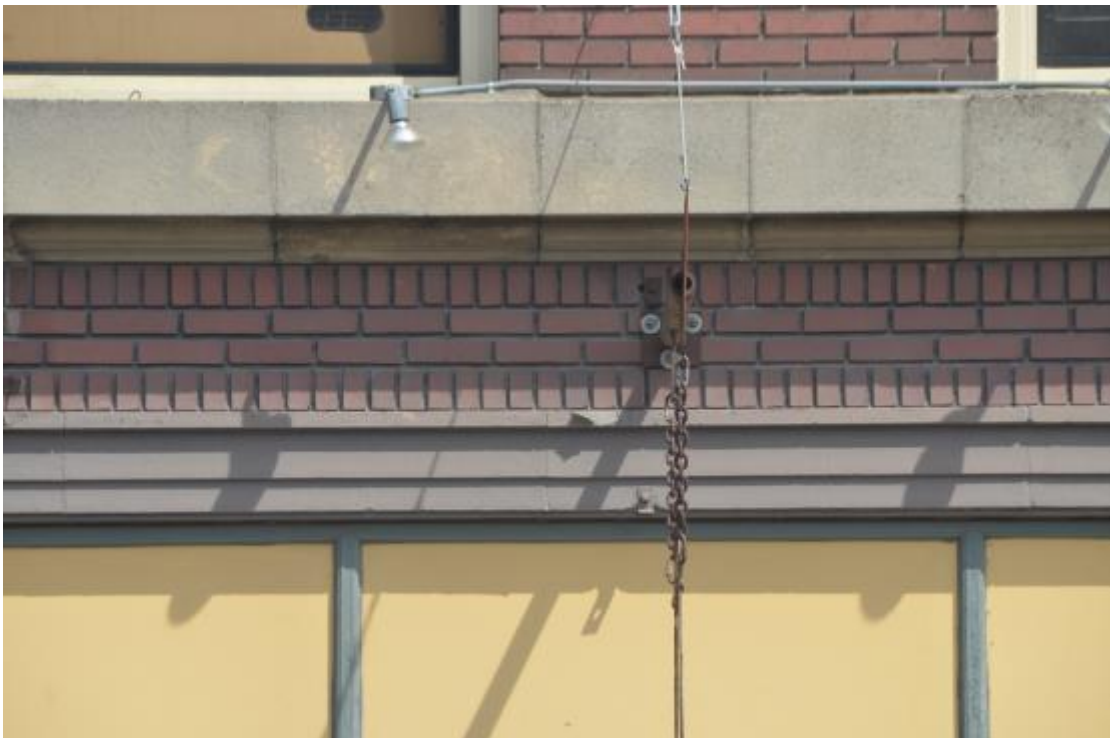
14. Detail of 2nd floor sill course, brick courses & header course
