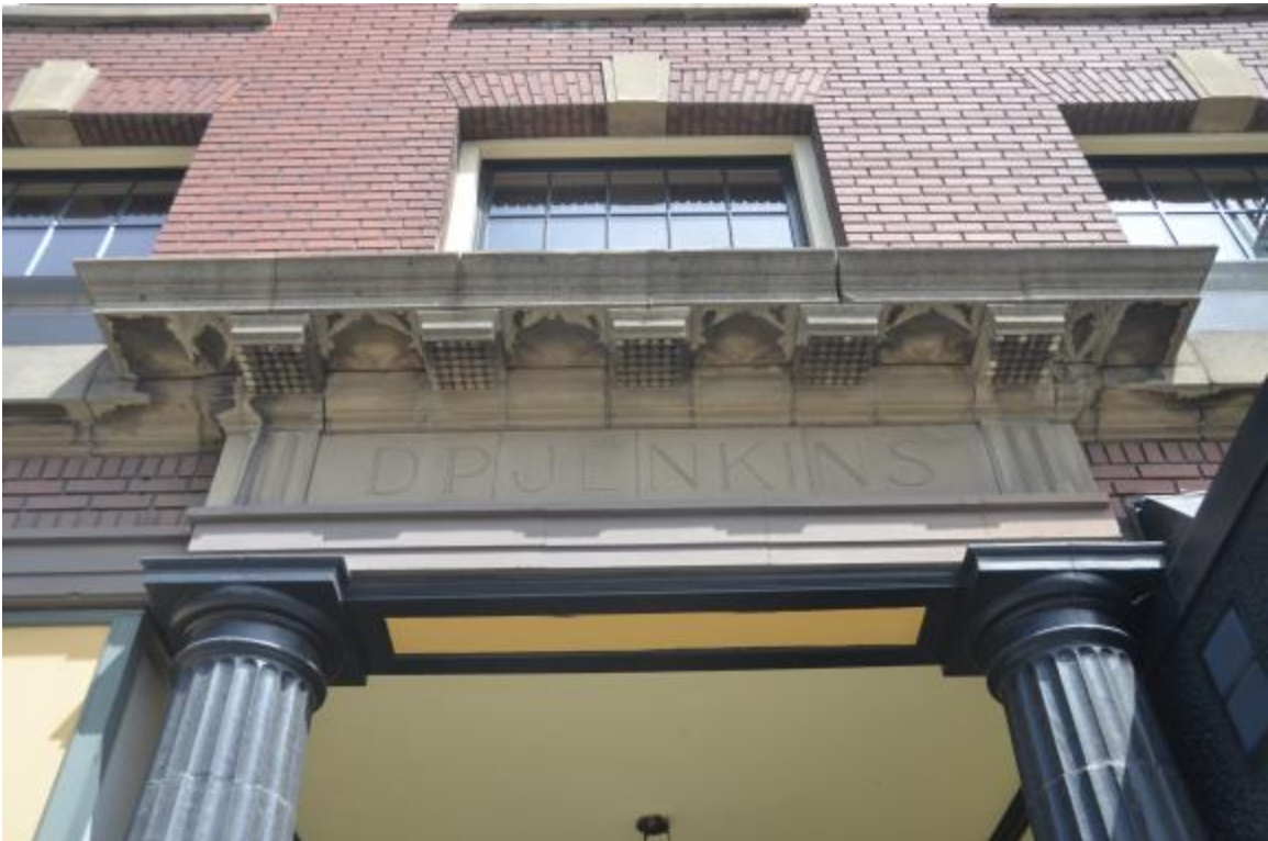
15. Detail of portico entablature, and window keystone
