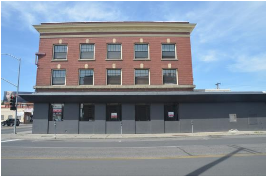
5. South facade, view to the north
