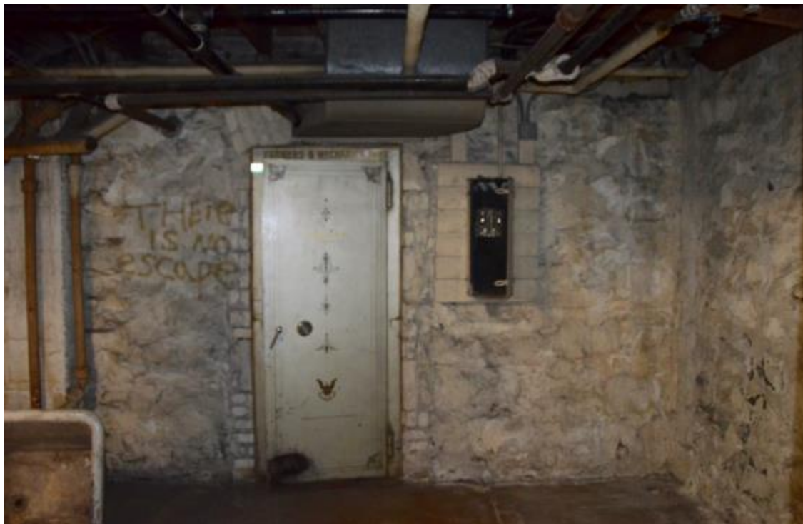
35. Farmers & Mechanics Bank door to vault room
