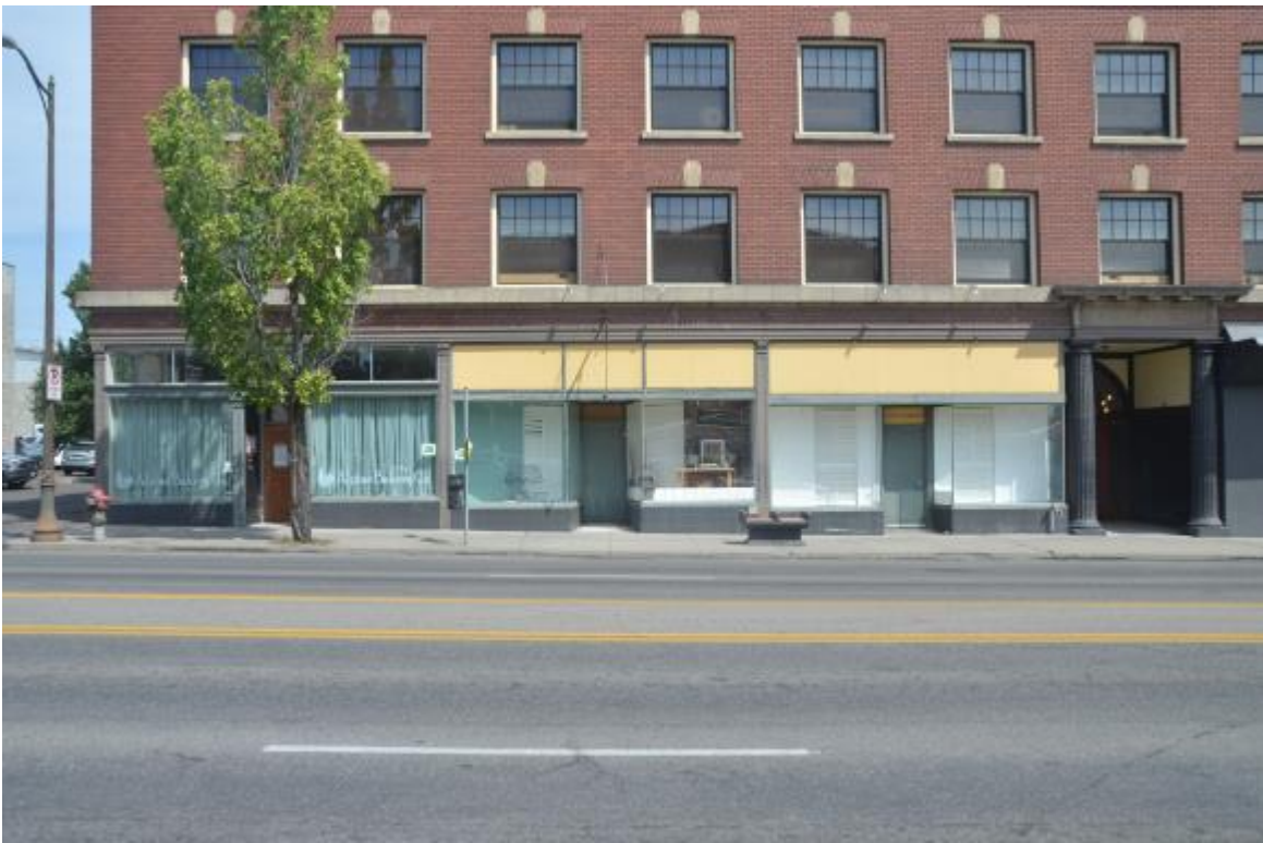
11. Retail bays 3, 4 & 5, and main entry, looking east
