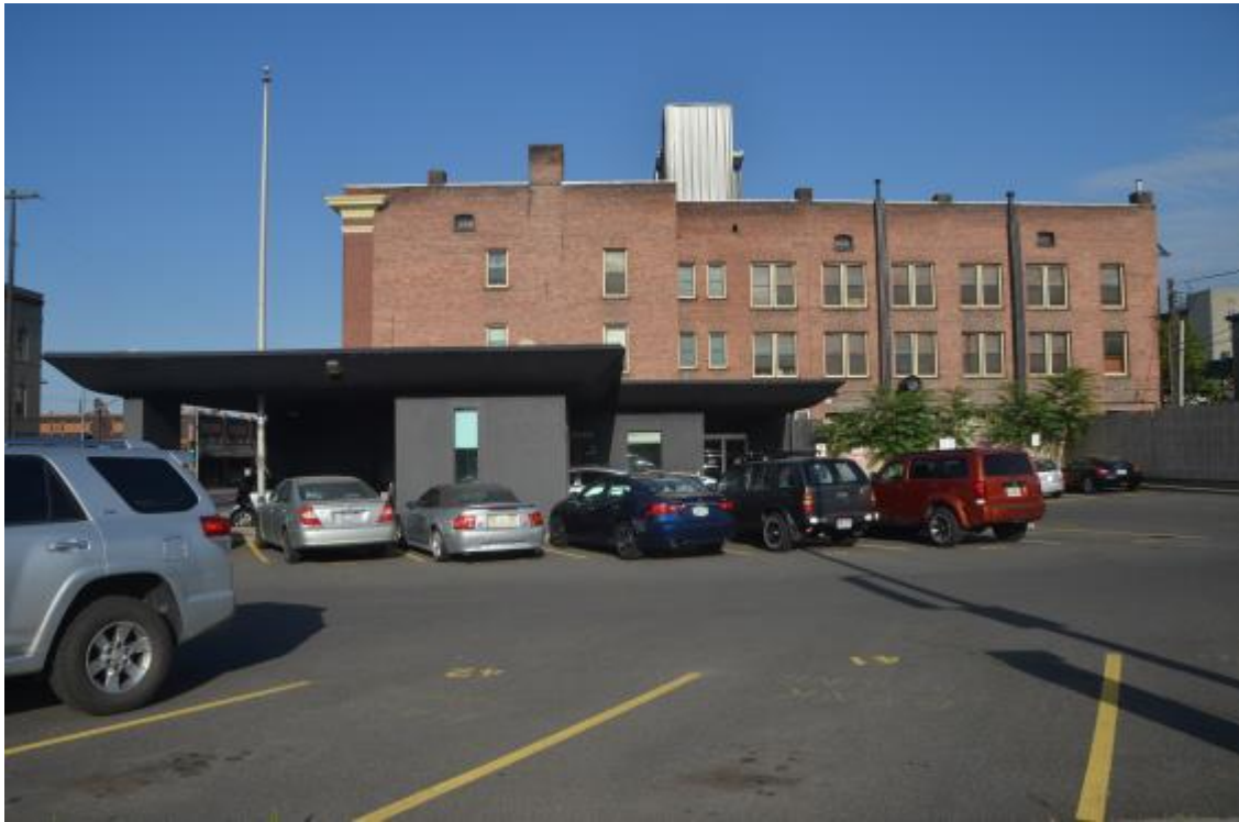
7. Rear facade, view to the west across parking lot
