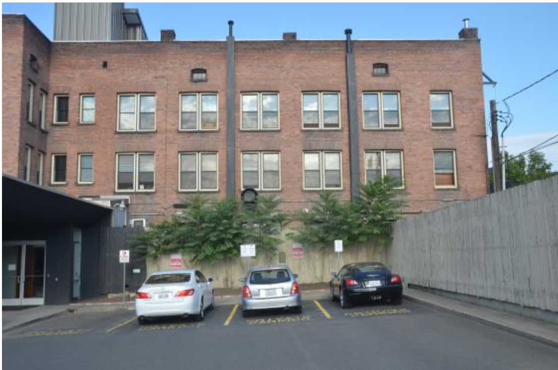
8. Rear facade (east), main wing, view to the west
