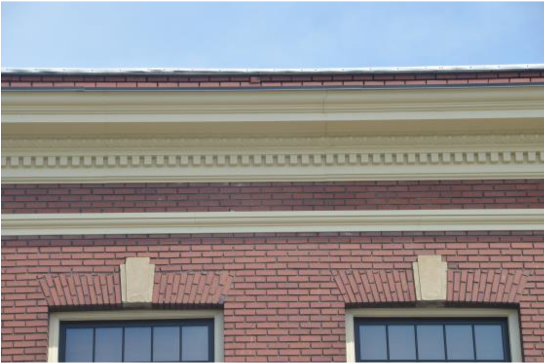
13. Detail of sheetmetal cornice and belt course, and 3rd floor window heads
