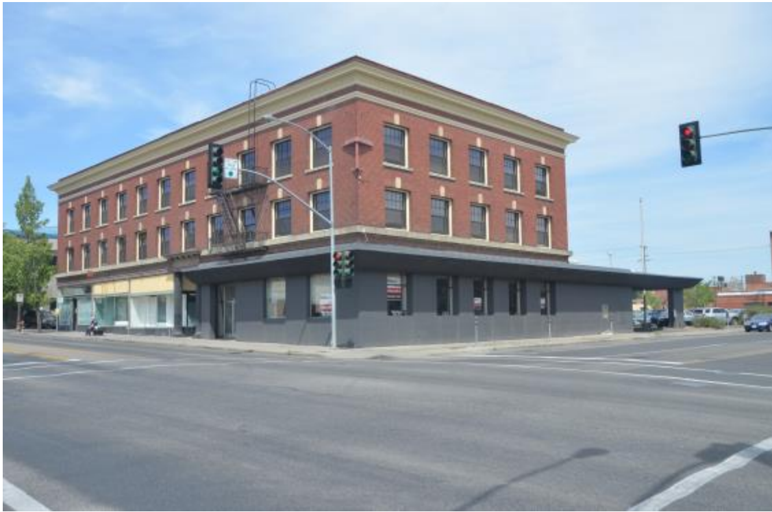
3. SW corner of building, west and south facades, view to the NE
