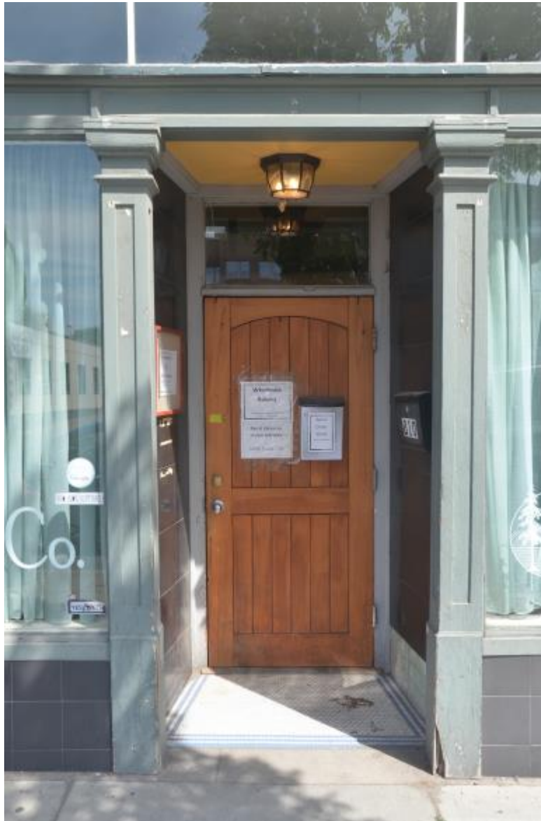
16. Entry to commercial bay at 510 N. Monroe (Alpine Bakery)
