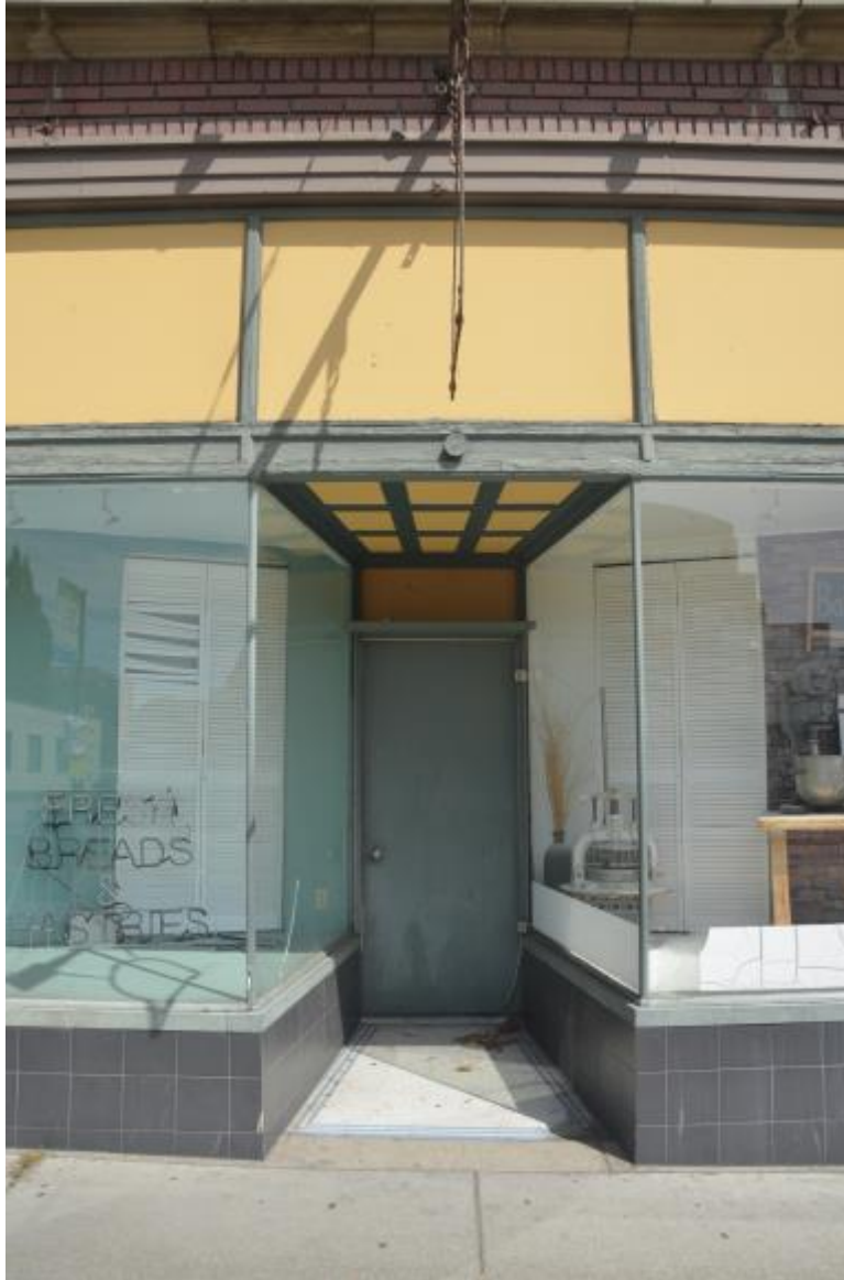
17. Entry to commercial bay at 508 N. Monroe (Alpine Bakery)
