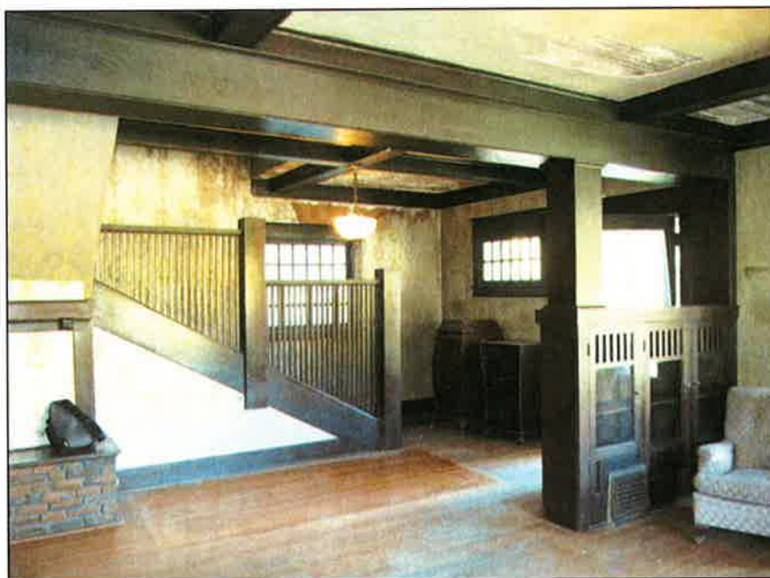
2015 photo of Eikenbary-Pierce House, showing original intact 1910 floor plan, lathe-and-plaster construction, oak floors, windows, and Craftsman-style woodwork, including built-ins, colonnade walls, and fireplace inglenook.
