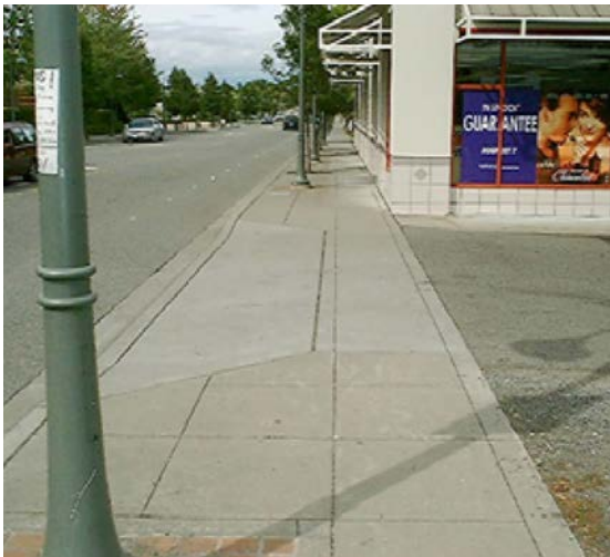
Figure 5.2.1 - Curb cuts and driveways may not interrupt sidewalk material and pattern requirements. Ramps may not encroach on Clear Pedestrian Zones.
