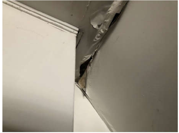
Photo #8 View of apparent mold and water intrusion in the shop areas ceiling at #3 at 2824 North Nevada Street.
