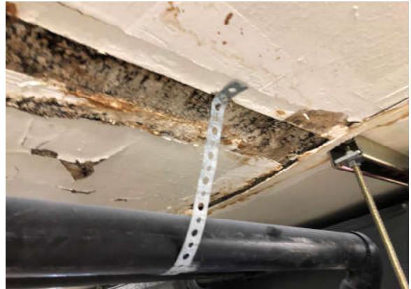
Photo #4 View of mold in loft at 2828 N. Nevada.
