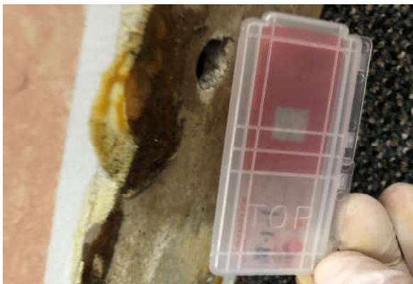
Photo #5 View of mold in breakroom at base of wall at 920 Wolverton Court.
