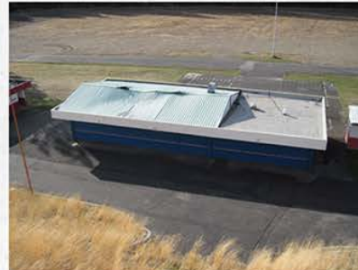
Concession roof has failed
