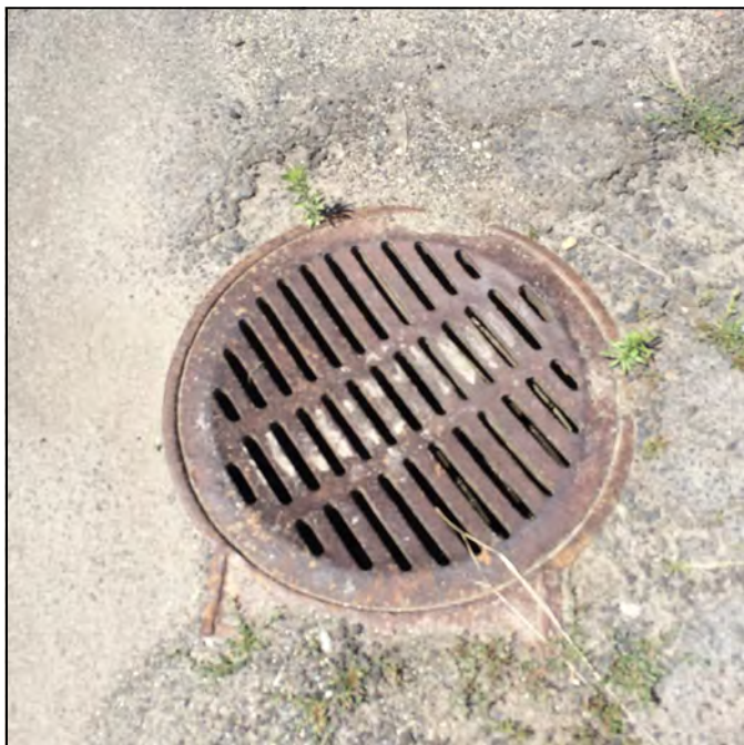
Photo 1: Shallow drywells (4 total) located at east bay doors of annex basement.
