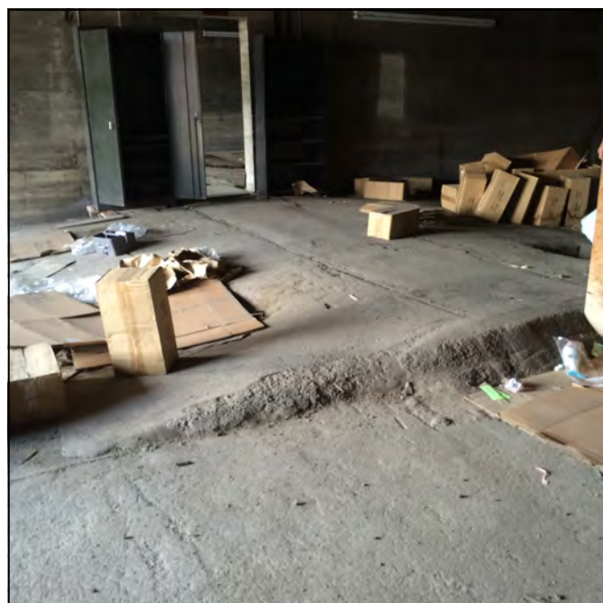
Photo 8: Center concrete ramp covers central chase in Mission Street sheds.
