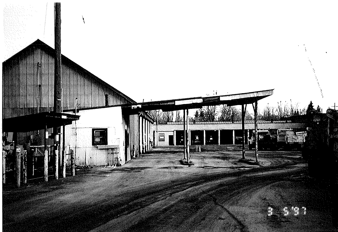
The diesel UST system before we started to excavate. The diesel fueling shed and pump islands were removed, along with the tank. The tank fill pipe is under the orange traffic cones in the background.
