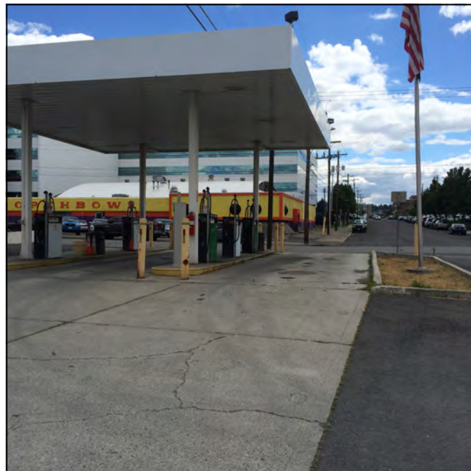
Photo 10: Active fleet fueling station on west end of Fleet building. Two in-use USTs under slab, five fuel pumps, grass swale with drywell on right of photo.
