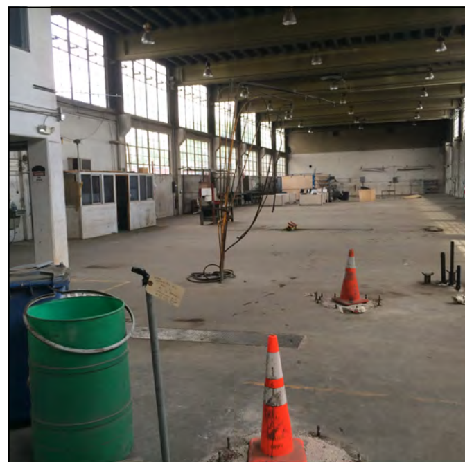
Photo 8: Main maintenance area of Fleet building on main floor, with 8 bays. Note hydraulic tubing penetrating floor in center of photo.
