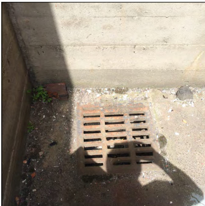
Photo 9: Grated sump in stairwell to Annex boiler room (northwest corner of building).
