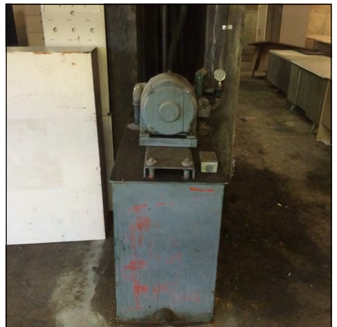
Photo 4: Two bays of the basement included hydraulic lift machinery, including this reservoir with oil stains around it.
