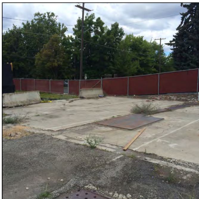
Photo 7: Metal plate on slab covers abandoned steam pipe chase.
