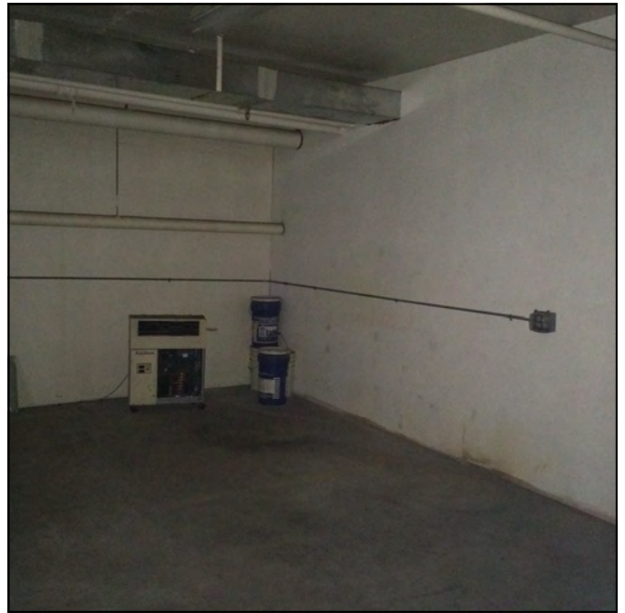
Photo 2: Some of the pipe insulation in the Fleet building basement may have asbestos.
