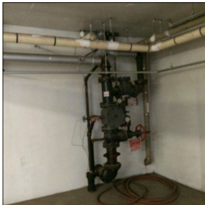
Photo 6: Additional pipe insulation in the basement that may be asbestos-containing.
