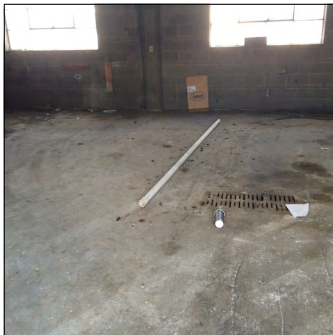
Photo 2: Sump in wash bay floor.
