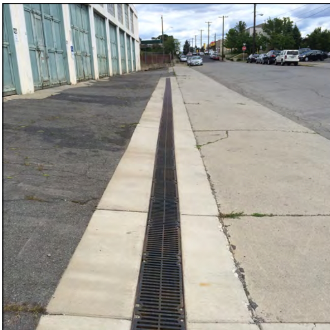
Photo 13: Trench drain along south entry to main floor of Fleet building maintenance bays. Drain is connected to combined sewer in West Sinto Avenue to right.
