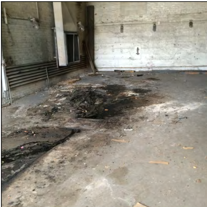
Photo 11: Thick petroleum deposit, possibly from asphalt truck parking, bay on west side of shop building ground floor.
