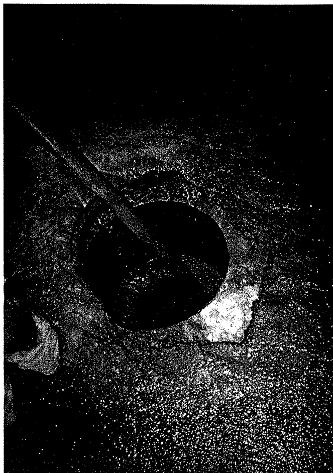
This picture was taken showing the backfill sand slurry mixture being deposited within the tank.
