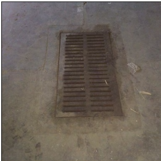
Photo 3: Several floor drains are spaced regularly in the bays of the Fleet building basement, but none of them appear to have oil stains.
