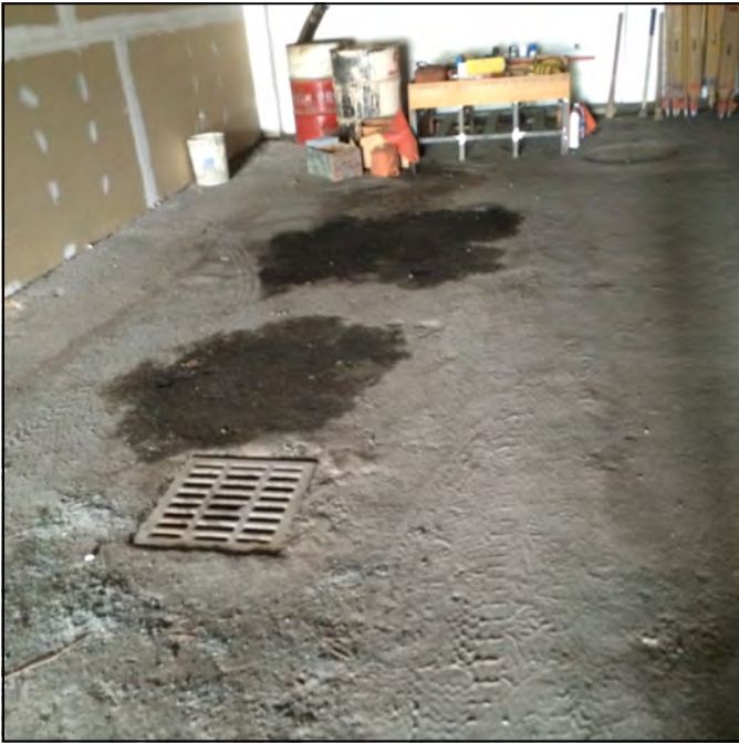
Photo 17: Oil stains near interior grated sump, annex basement, surveyor's storage bay.
