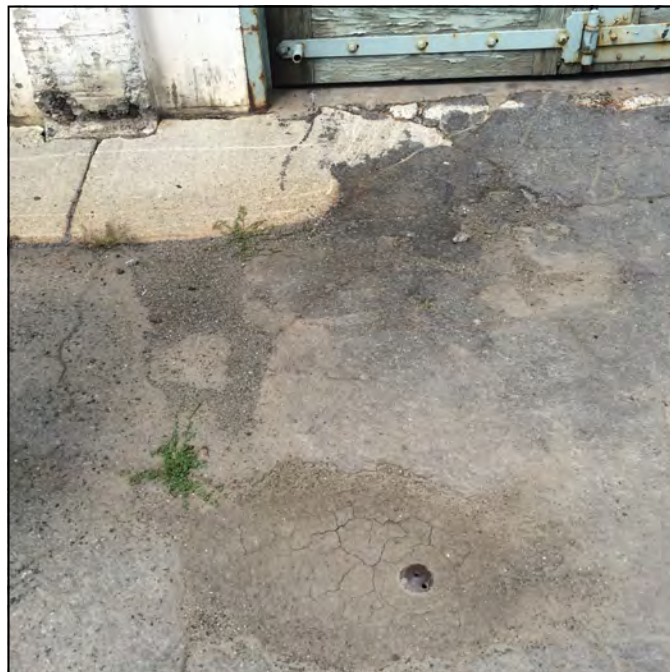
Photo 14: Black spot in lower center of photo is in sump and is sediment-covered area drain at south entry to east-most bay of Fleet building main floor.
