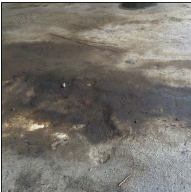
Photo 1: Extensive staining of south wash bay floor.
