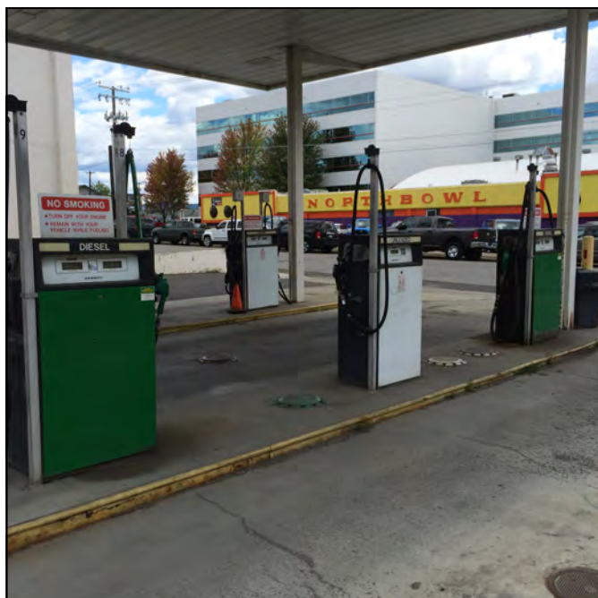
Photo 11: Some staining of concrete slab under fuel canopy.
