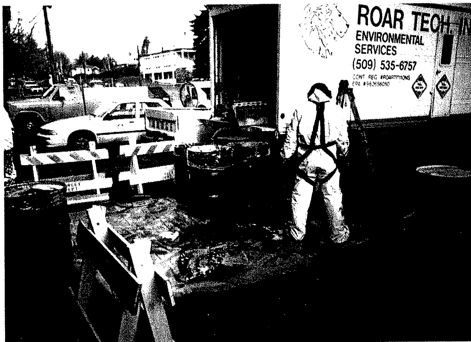
Picture shows the removal of the remaining PS300 heating fuel from the tanks. This picture was taken looking in a northerly direction.
