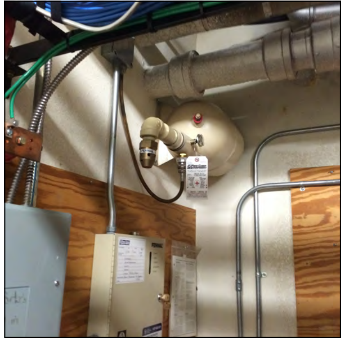
Photo 18: Chemical fire suppression system in basement IT room.
