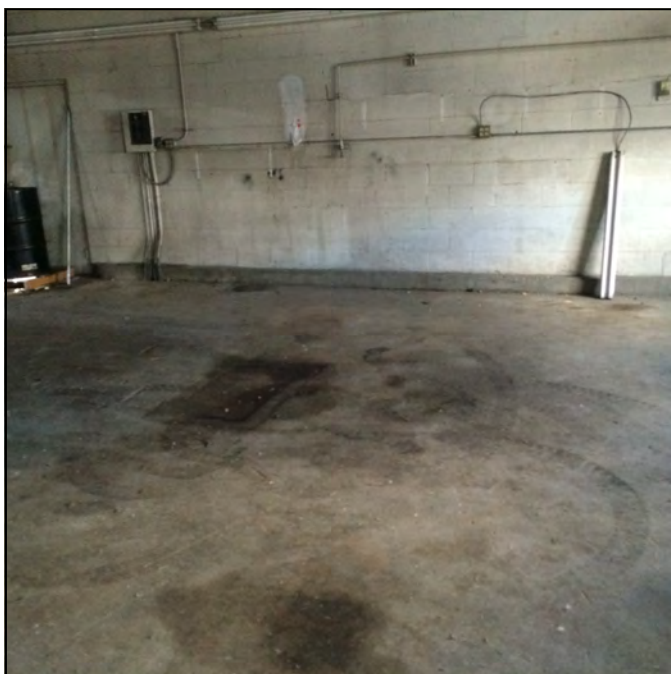
Photo 9: More of small vehicle maintenance floor ; 55-gallon oil drum without secondary containment at far left.
