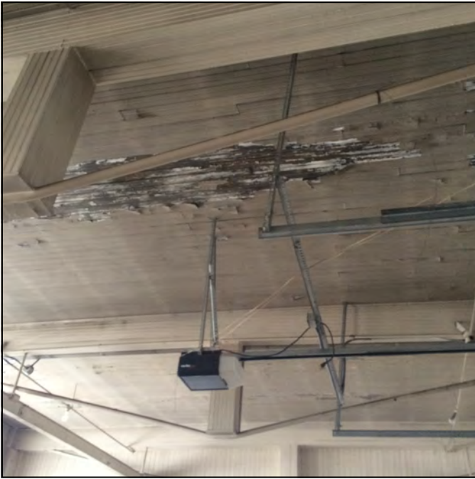
Photo 5: Ceiling of top floor with peeling paint.
