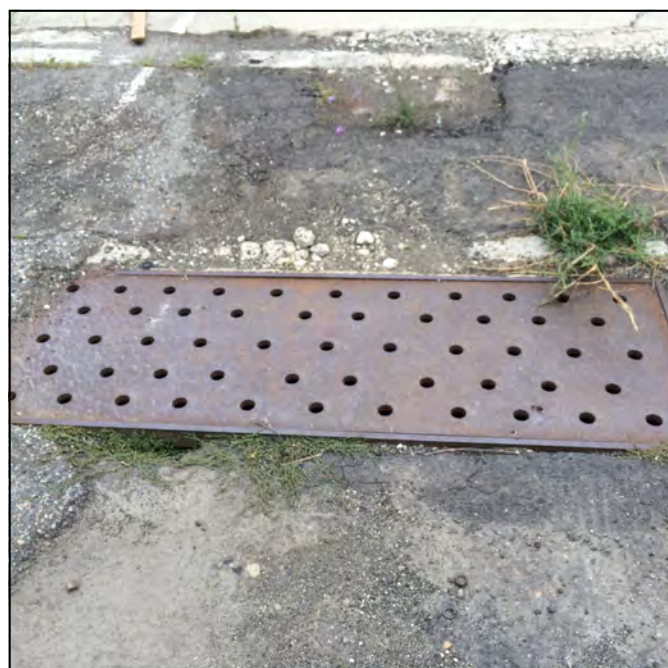
Photo 8: Perforated plate grate at entry to demolished shop.
