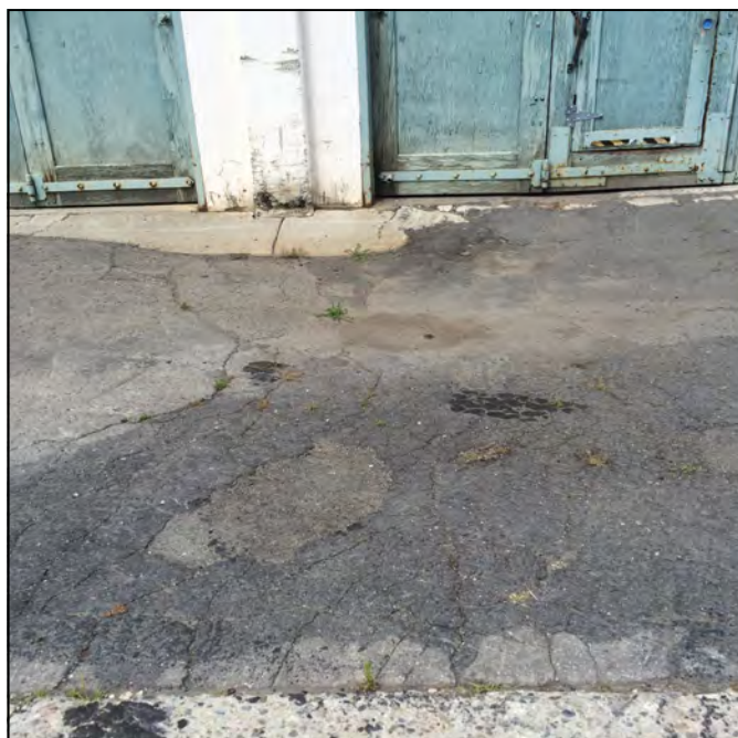
Photo 15: Staining of apron on south side of main floor of Fleet building.
