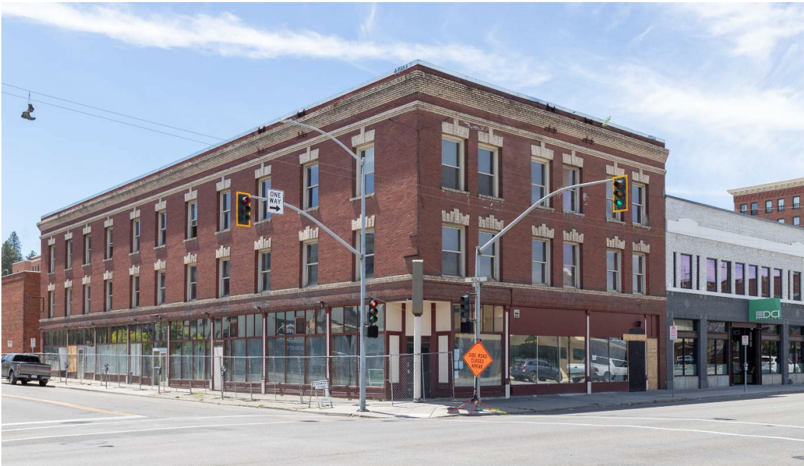
Photo 0002. Exterior, northeast corner, intersection of South Wall Street and West Second Avenue.
