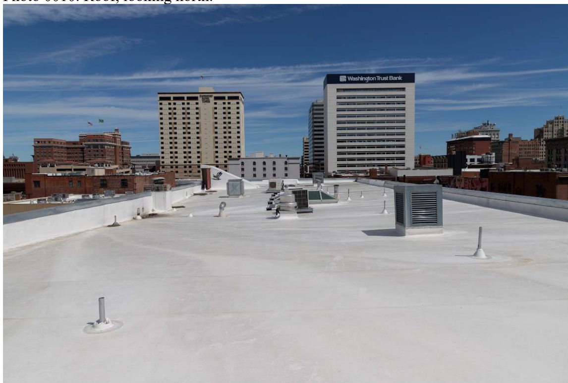
Photo 0010. Roof, looking north.
