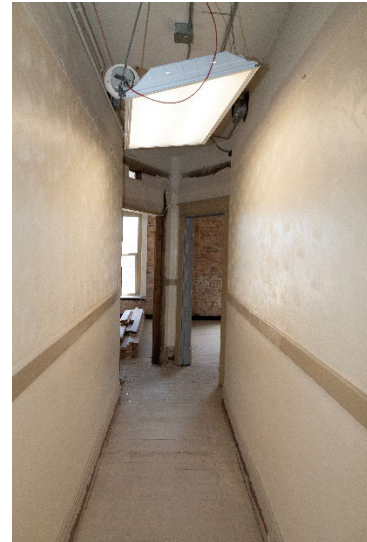
Figure 17. Second floor typical branch hallway.
