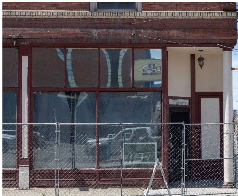
Figure 3. East facade, cast iron post (left edge of photo) and cast iron column (right edge of photo) view.
