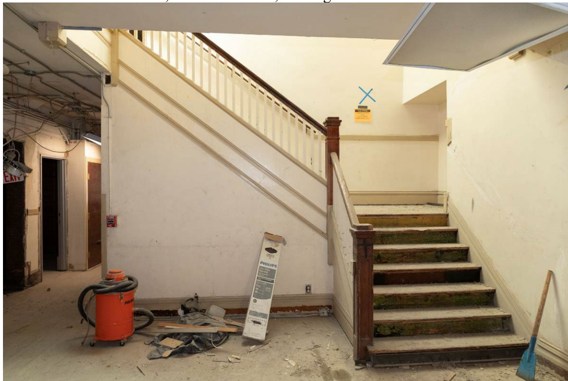
Photo 0024. Second floor, central stairwell, looking north.
