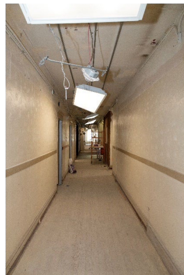
Figure 18. Second floor, main hallway.
