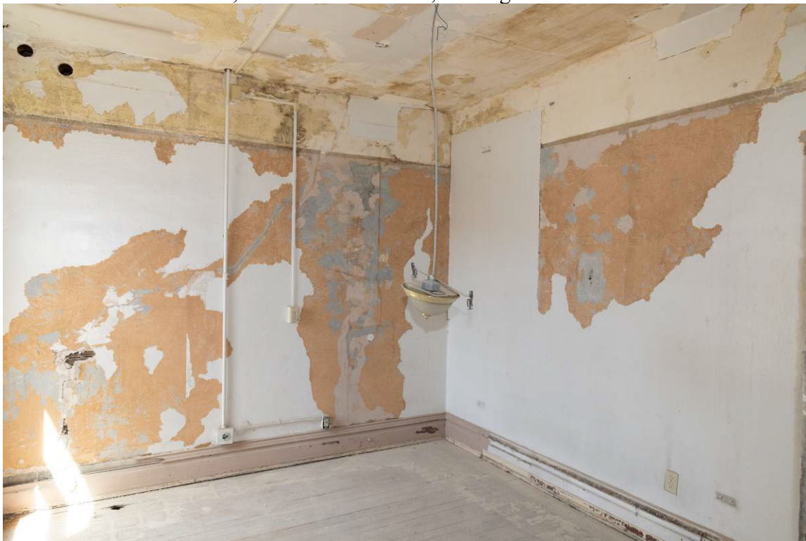
Photo 0034. Second floor, southeast corner unit, looking northwest.
