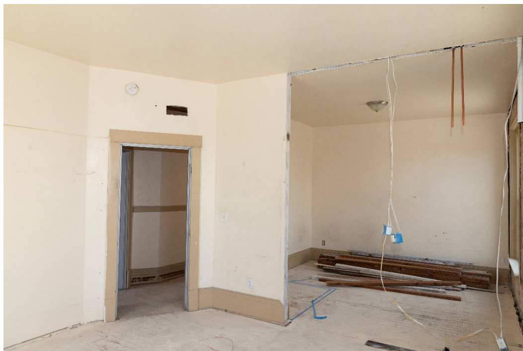
Figure 21. Third floor, showing typical unit finishes.
