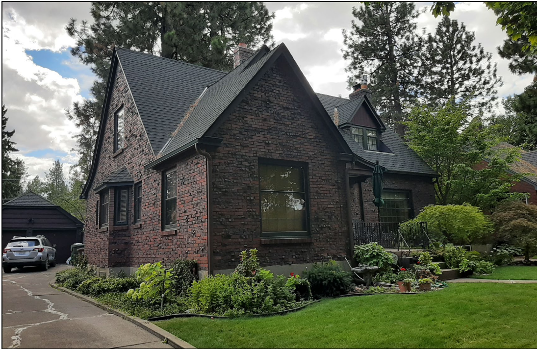
Looking south at the northeast façade corner of the Cooke House
