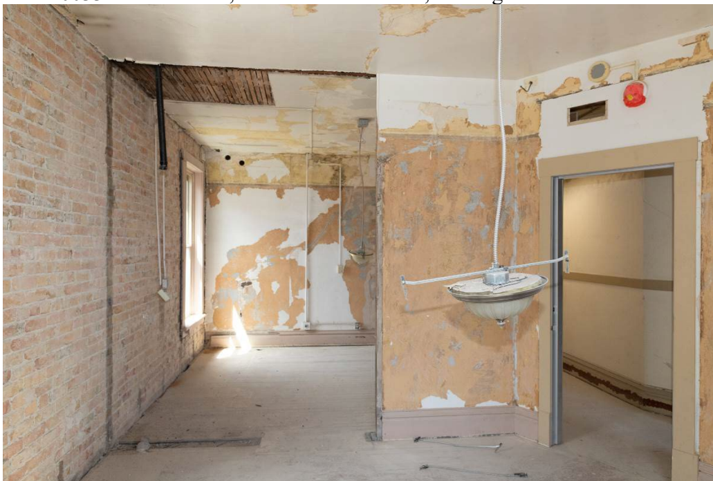
Photo 0033. Second floor, southeast corner unit, looking west.
