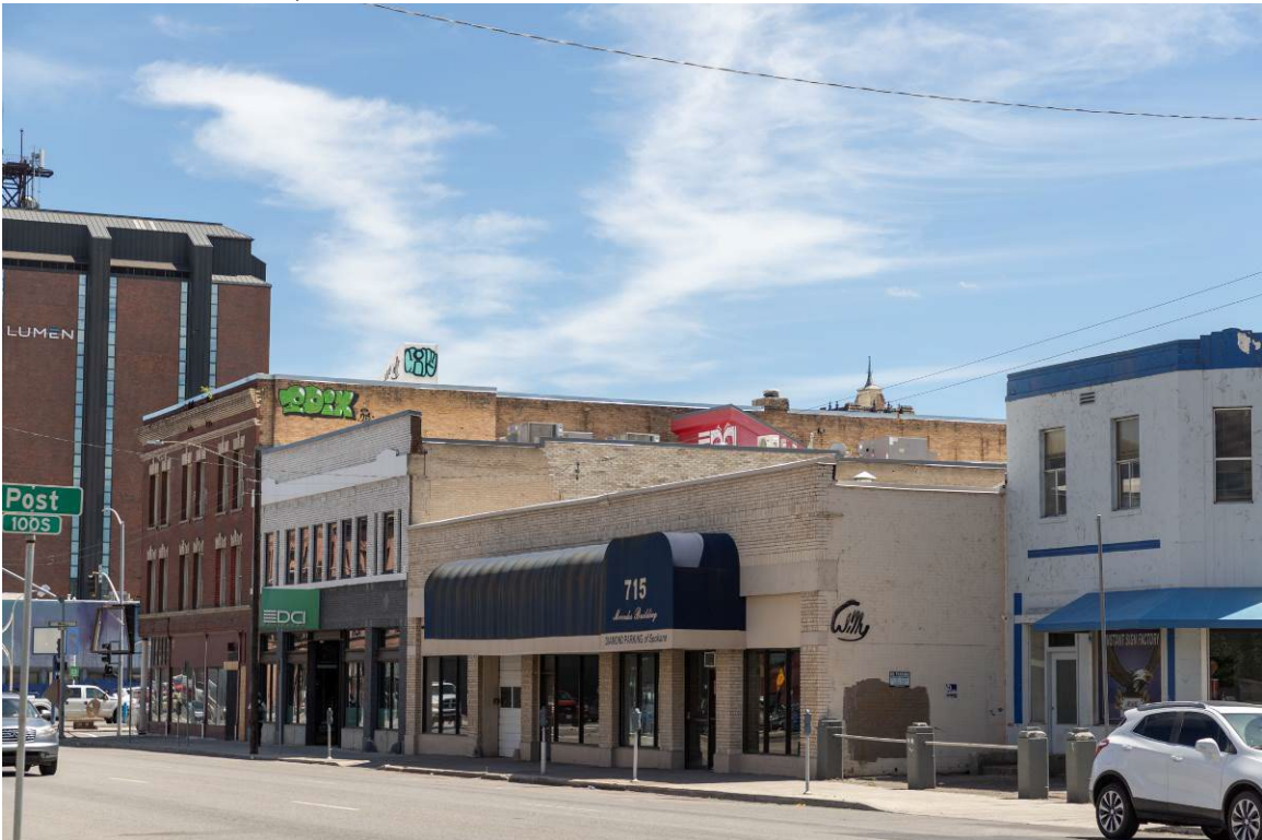
Photo 0005. Exterior, west facade.
