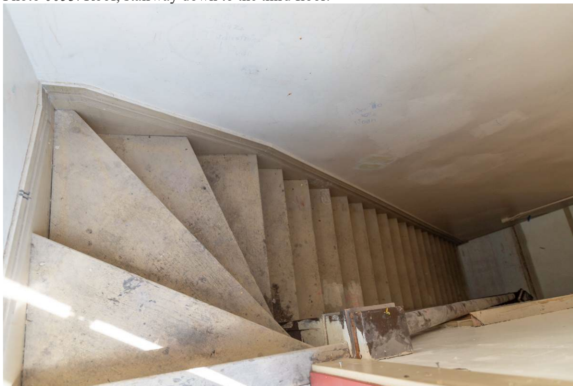
Photo 0053. Roof, stairway down to the third floor.
