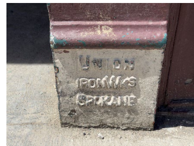
Figure 2. Cast iron pedestal detail showing factory stamp.
