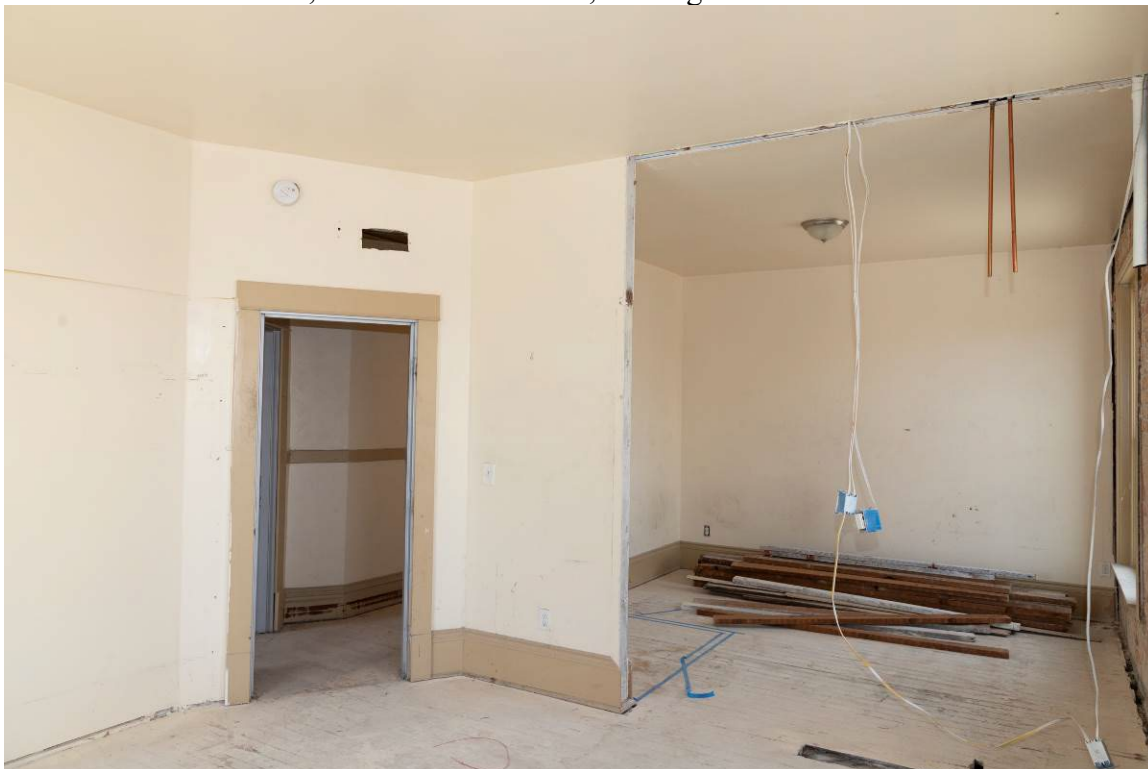
Photo 0048. Third floor, northeast corner unit, looking southwest.
