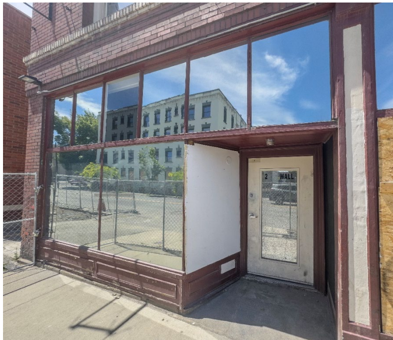
Figure 8. 212 South Wall Street storefront, showing original design.
