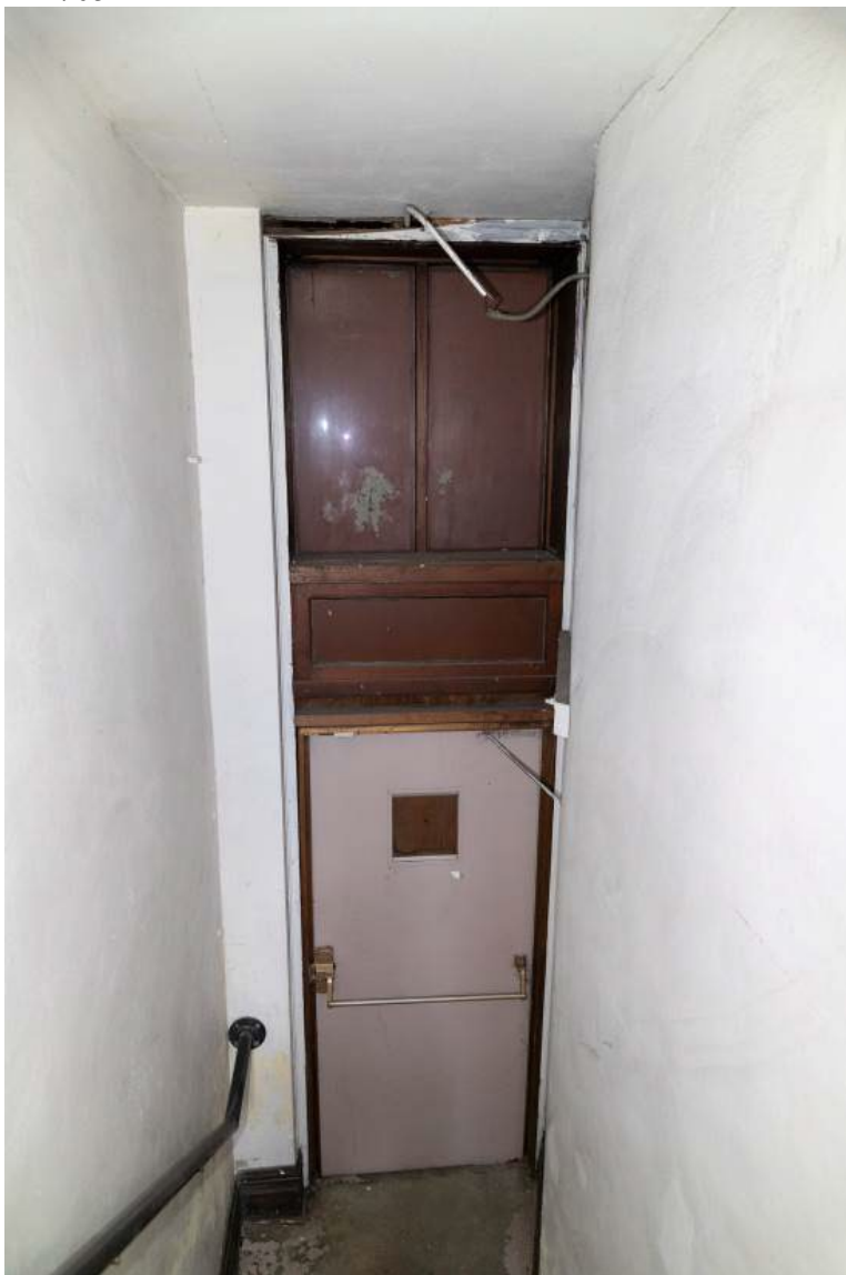
Photo 0038. Second floor, northwest stairwell, down up from the intermediate landing at the 705-1/2 West Second Avenue entrance.
