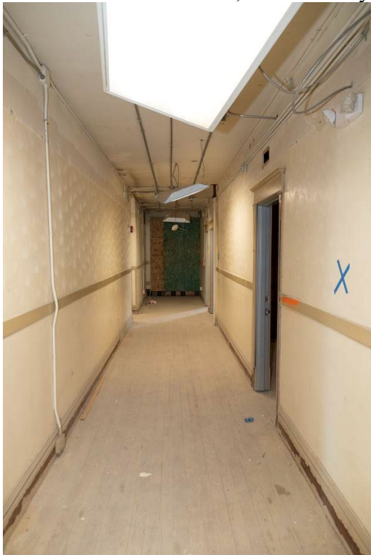
Photo 0028. Second floor, main hallway, looking south.
