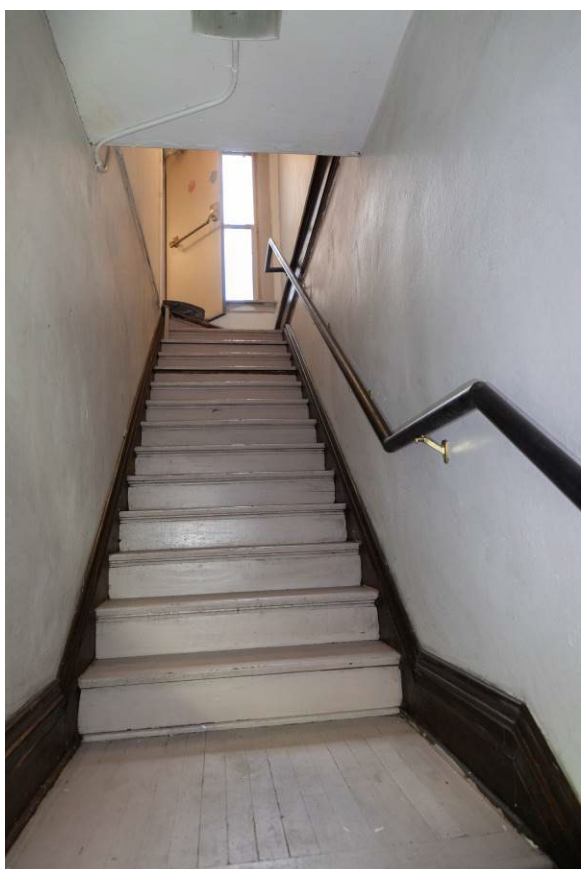
Photo 0037. Second floor, northwest stairwell, looking up from the intermediate landing.
