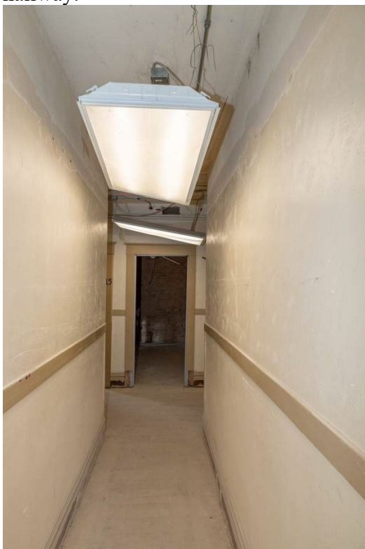
Photo 0032. Second floor, typical branch hallway, looking west towards the main hallway.
