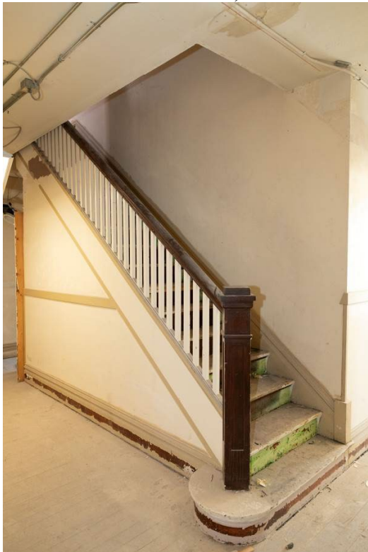
Photo 0039. Second floor, northwest stairway, looking northwest.
