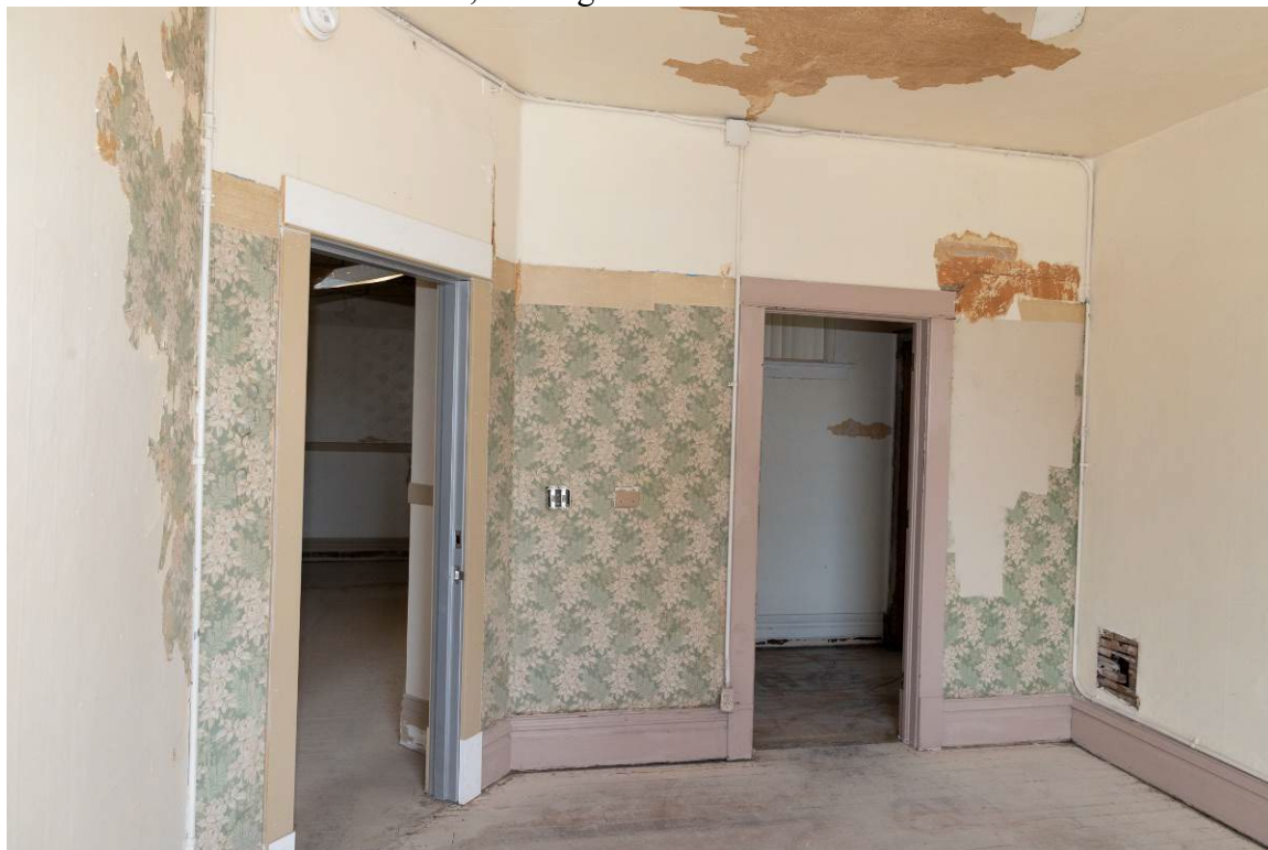
Photo 0052. Third floor east unit, looking west.
