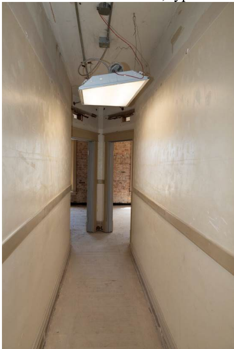
Photo 0030. Second floor, typical branch hallway extending east of the main hallway.
