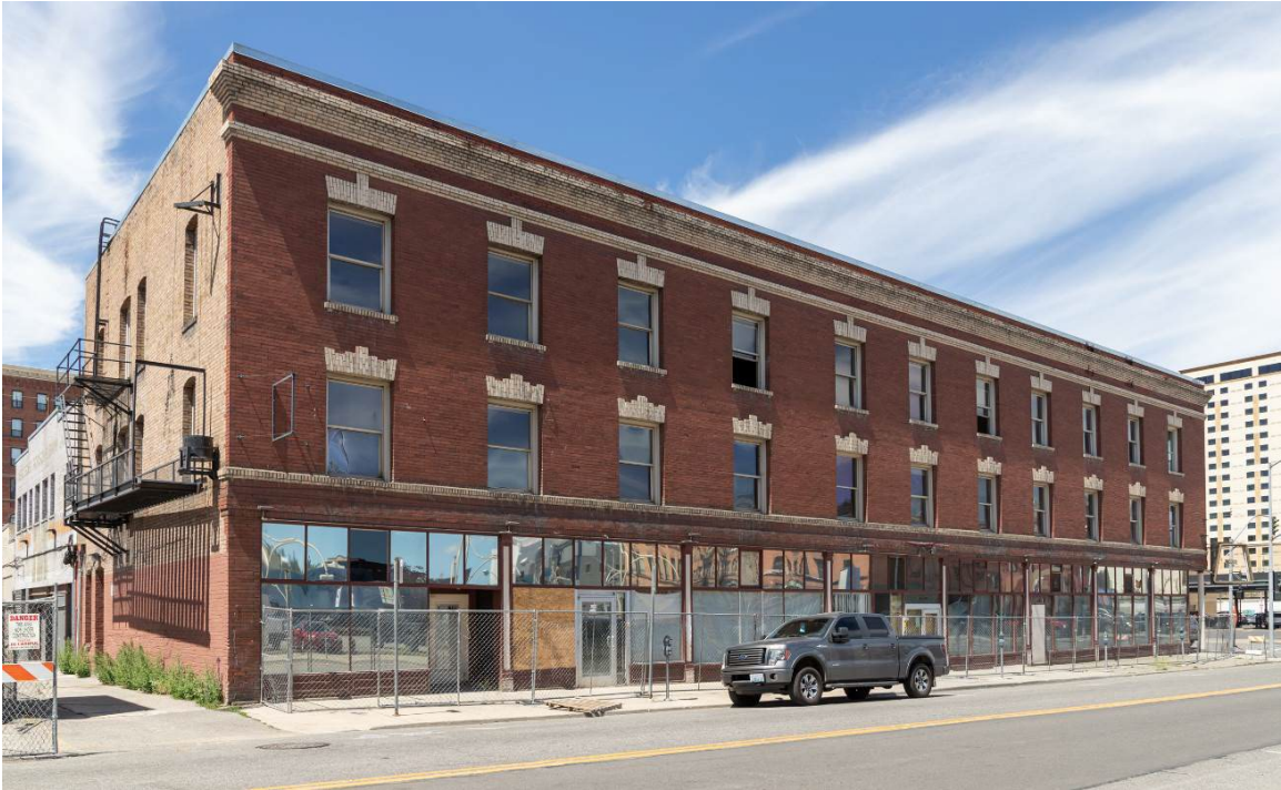
Photo 0004. Exterior, southeast corner.
