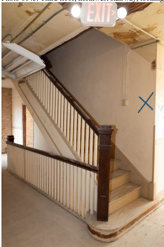
Photo 0045. Third floor, northwest stairway, looking northwest.
