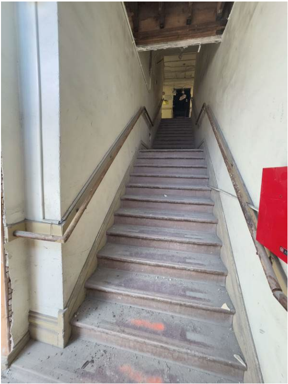
Photo 0022. First floor, central stairway, looking up from the 204 South Wall Street entrance.
