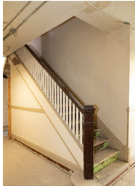
Figure 13. Northwest stairway looking up from the second floor (right).
