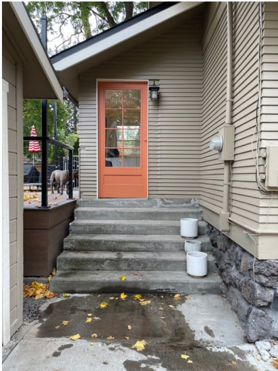
Figure 7: Rear steps to mudroom and back entry in 2024
