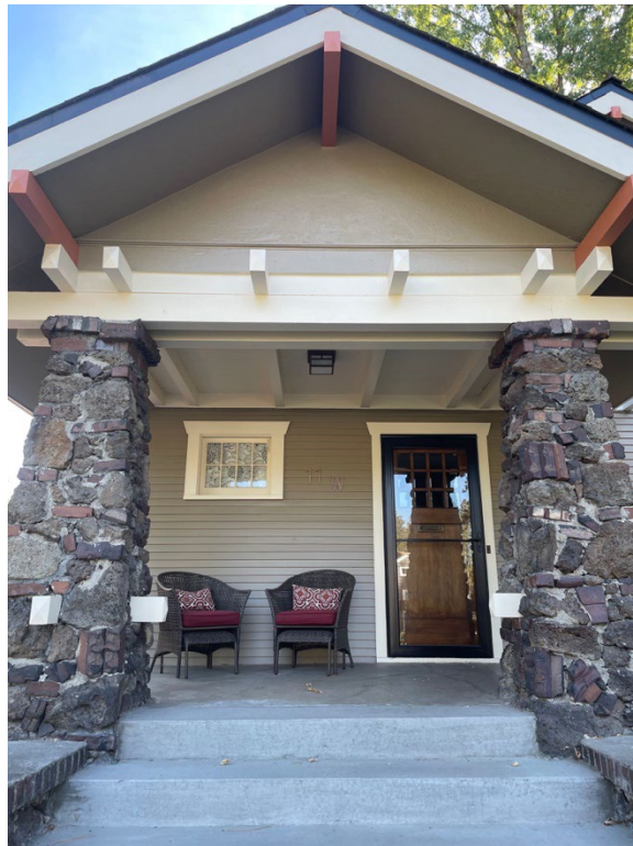
Figure 4: Porch roof and gable in 2024
