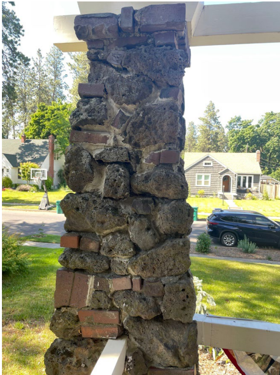
Figure 2: Rubblemix column at west end of front porch
