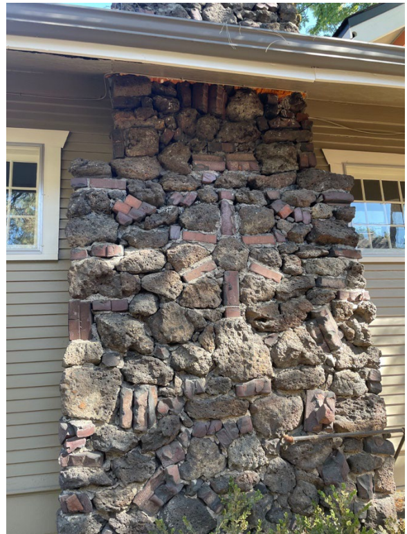
Figure 6: Decorative brick inlay in chimney
