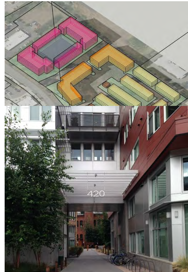
Figure 19. A through-block connection featuring a cantilevered building extending over a portion of the connection.
