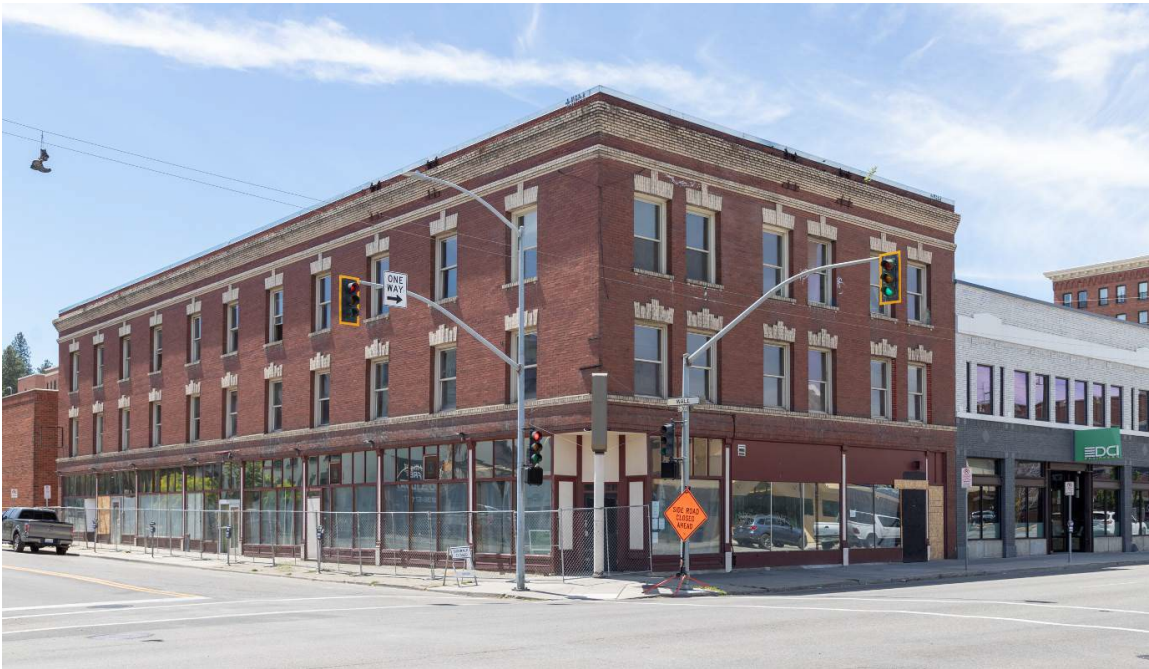
Photo 0002. Exterior, northeast corner, intersection of South Wall Street and West Second Avenue.
