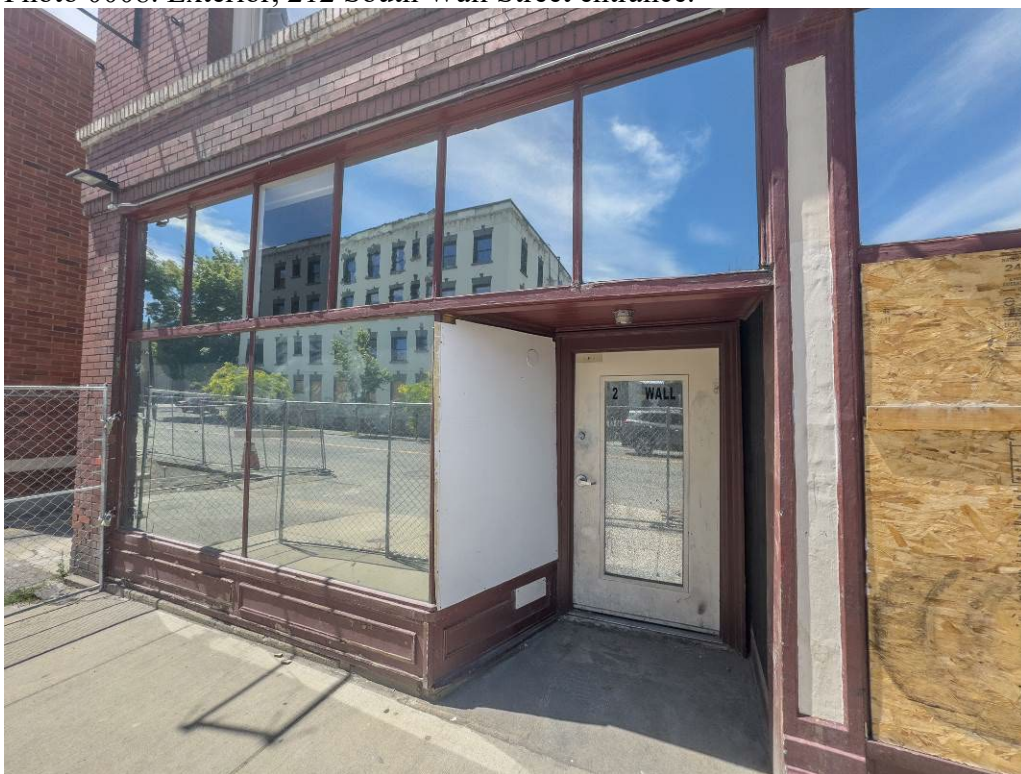
Photo 0008. Exterior, 212 South Wall Street entrance.
