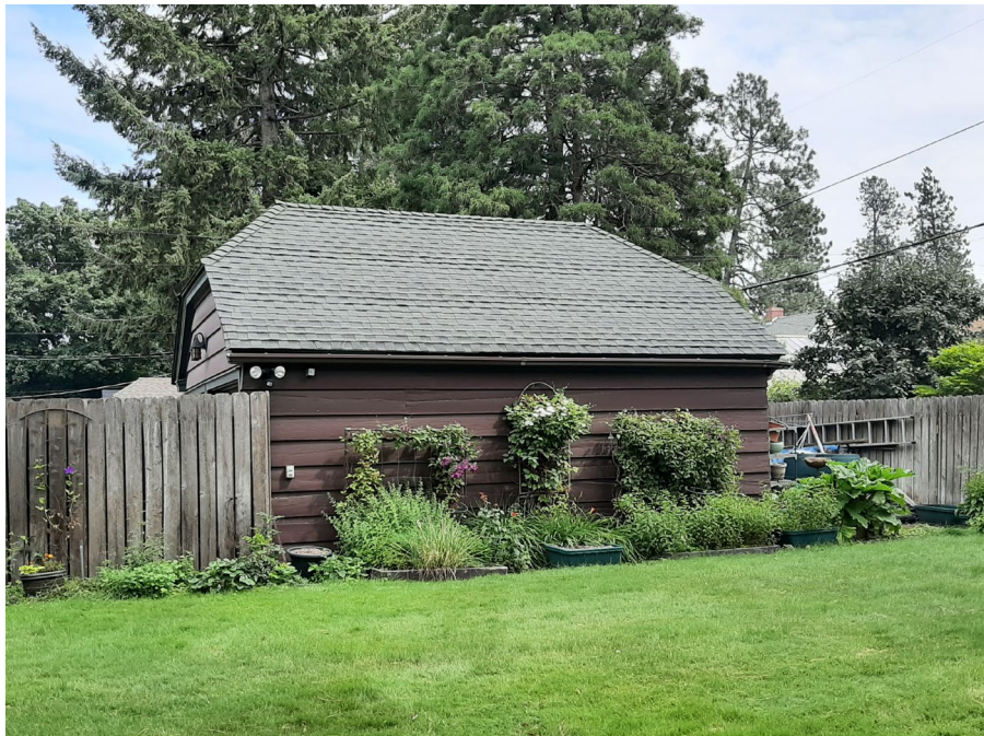
Photo 6 2024 photo facing east at the west elevation of garage
