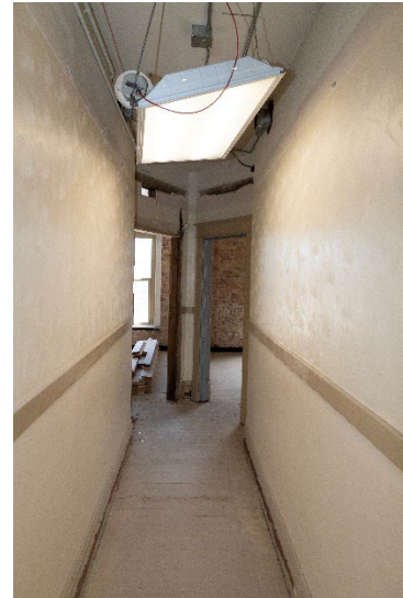
Figure 17. Second floor typical branch hallway.
