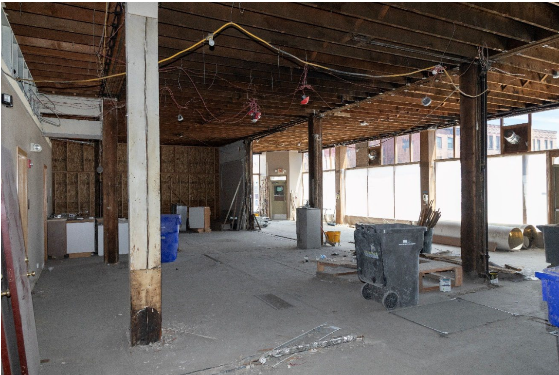
Figure 16. First floor, looking northeast.
