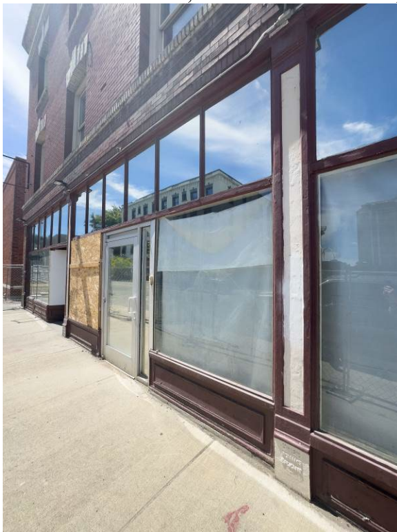
Photo 0007. Exterior, east facade storefronts, looking south.
