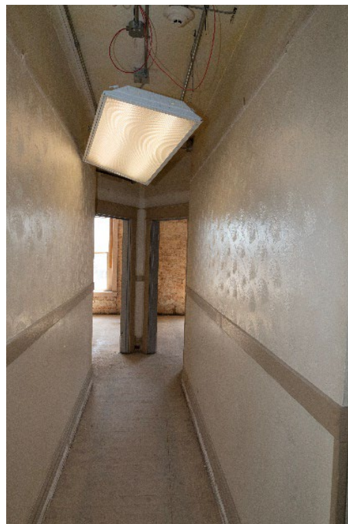
Figure 22. Third floor, typical branch hallway.
