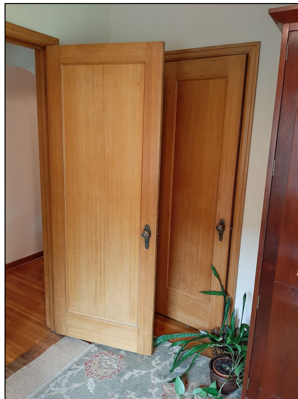
Photos 15 and 16 2023 photographs of built-in phone niche and interior doors on first floor—the original niche and doors are made of gumwood
