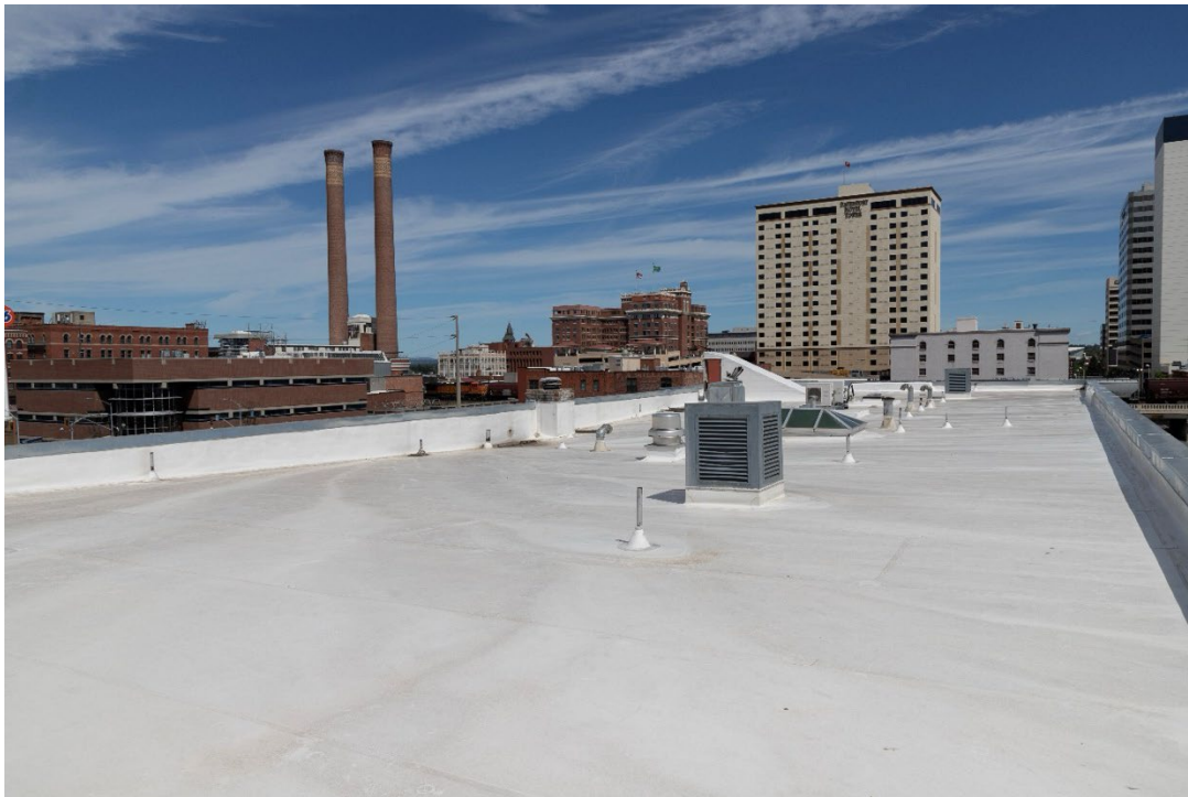
Figure 4. Roof, looking northwest.
