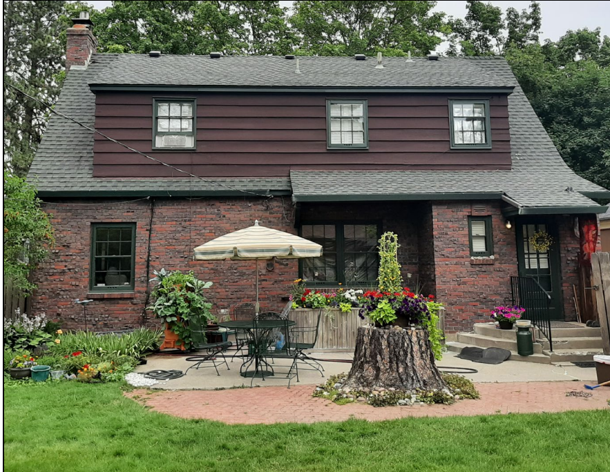
Photo 4 A 2024 photograph of the south rear face of the Cooke House
