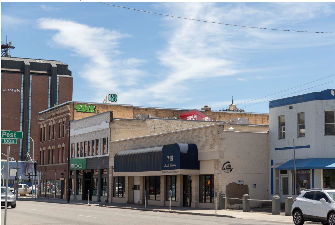
Photo 0005. Exterior, west facade.
