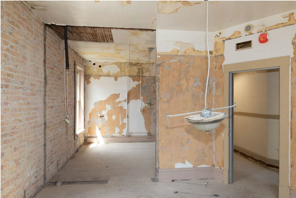
Photo 0033. Second floor, southeast corner unit, looking west.
