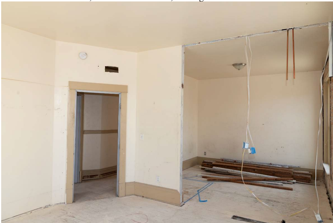
Photo 0048. Third floor, northeast corner unit, looking southwest.
