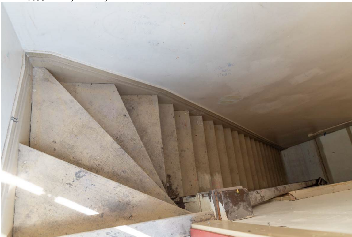
Photo 0053. Roof, stairway down to the third floor.
