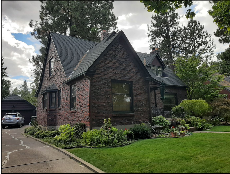
Photo 3 2023 photograph of north façade and east wall along driveway of Cooke House
