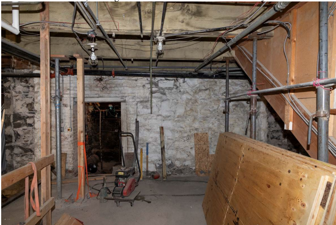
Photo 0013. Basement, looking west towards the boiler room doorway.
