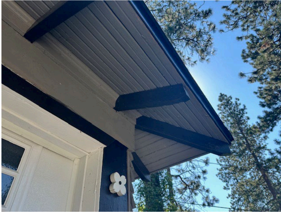
Photo 7 2024 photo of garage's eaves at south façade and west elevation
