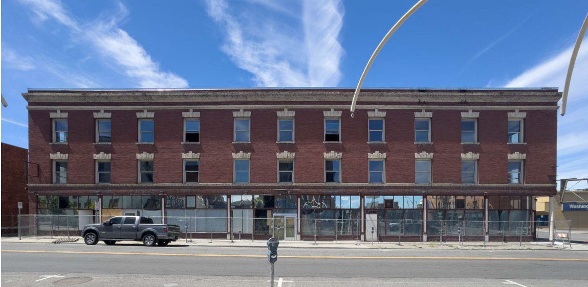
Photo 0003. Exterior, front east facade, South Wall Street.
