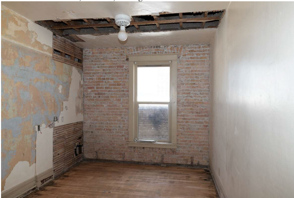
Photo 0050. Third floor, west unit, looking west.
