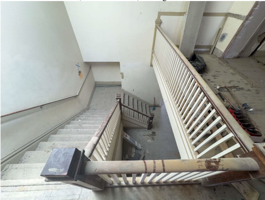
Photo 0040. Third floor, central stairwell, looking east and down.
