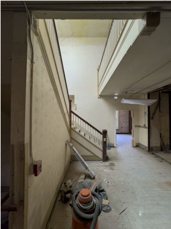
Photo 0025. Second floor, central stairwell, looking east.
