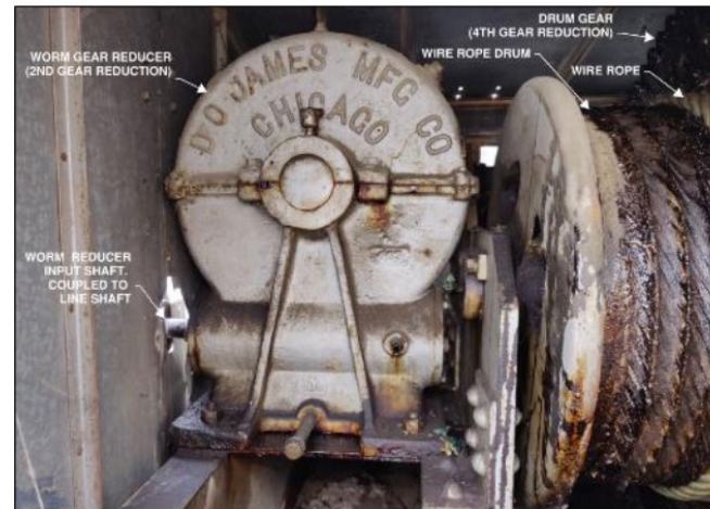
Project: Gate and hoist replacement
