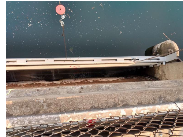
Project: Stoplog Replacement
