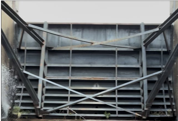
Project: Gate and hoist replacement
