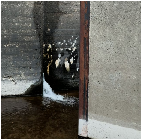
Project: Seepage mitigation
