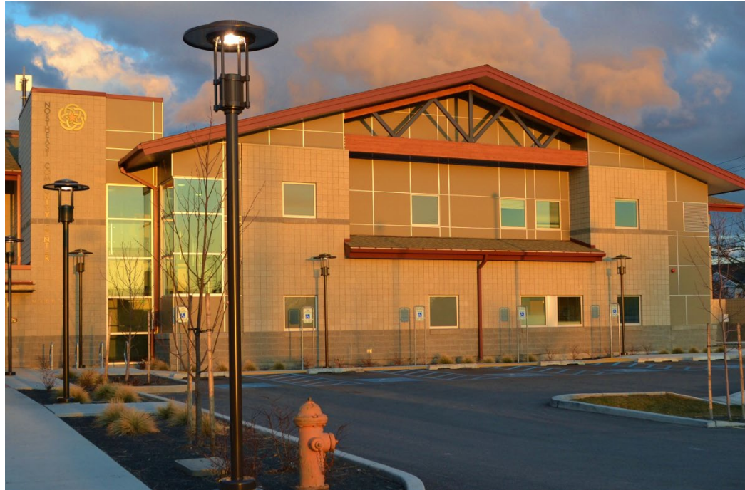
Northeast Community Center
