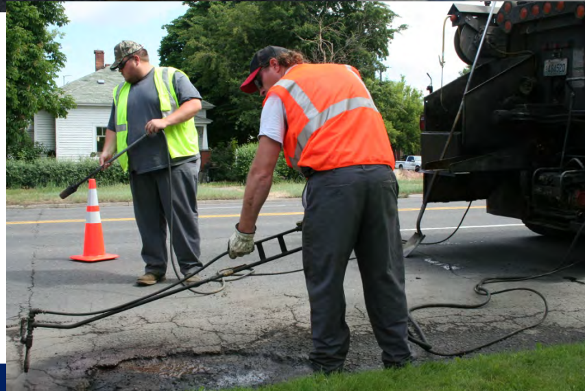
Pothole Repairs
