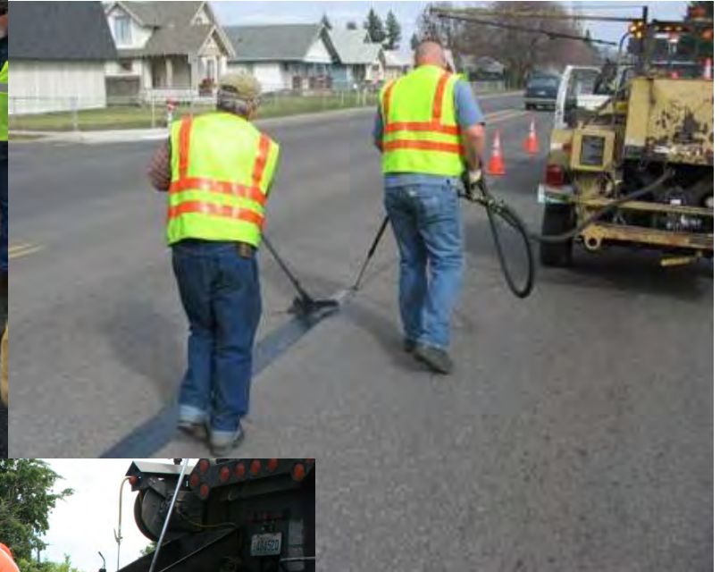
Crack Sealing
