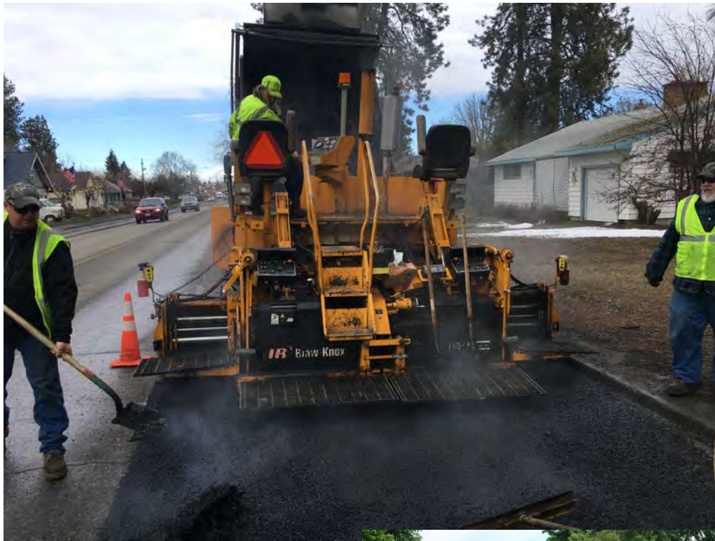
Patch Repairs
