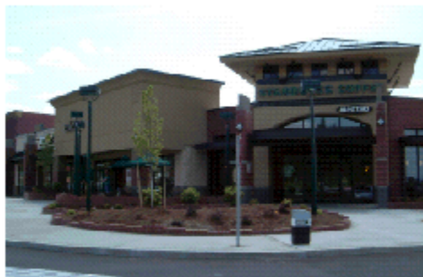
Plaza located at main entrance
