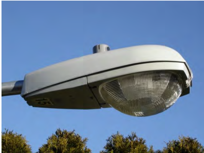
Typical cobra head light
