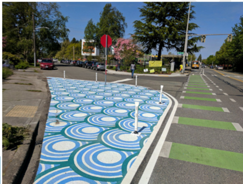
Curb Extension, Seattle Right-of-Way Improvements Manual
