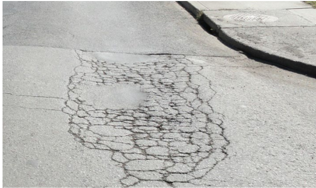
Alligator Cracking
