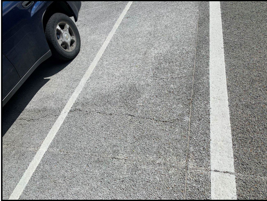
Linear Cracks
