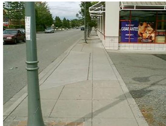
sidewalk pattern is visibly continuous
