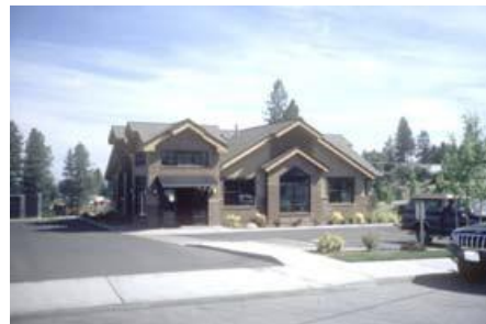
6 inch vertical curb defines pedestrian connection
