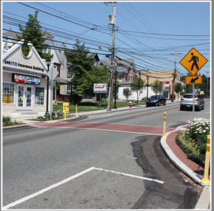
BULB-OUT CROSSWALK Bulb-outs, also known as curb extensions, enhance pedestrian safety by increasing pedestrian visibility, shortening crossing distances, slowing turning vehicles, and visually narrowing the roadway.
