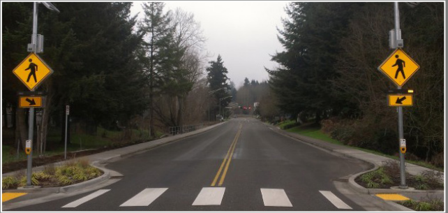
RECTANGULAR RAPID FLASHING BEACON (RRFB) These pedestrian-initiated signals can enhance safety by reducing conflicts between vehicles and pedestrians at unsignalized intersections and mid-block crossings. Design can include bulbouts to improve visibility of pedestrians.
