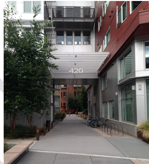
Figure 19. A through-block connection featuring a cantilevered building extending over a portion of the connection.
