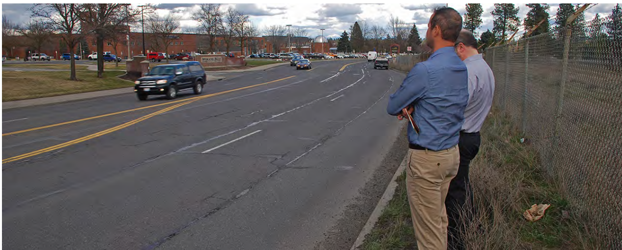
Figure 1.09 – Current conditions favor through-traffic, featuring four travel lanes (no turn lane), little landscaping, no bicycle lanes, sidewalks that abut the curb to the north, and extensive gaps where sidewalks do not exist on the south. Speeding along the corridor is a persistent issue, and just one crosswalk exists along the 1.2-mile stretch within the study area. (Image: Studio Cascade, Inc.)
