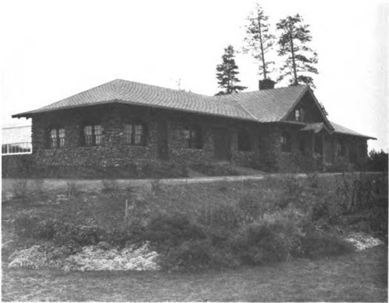
Tool House and Work Room, Manito Park
