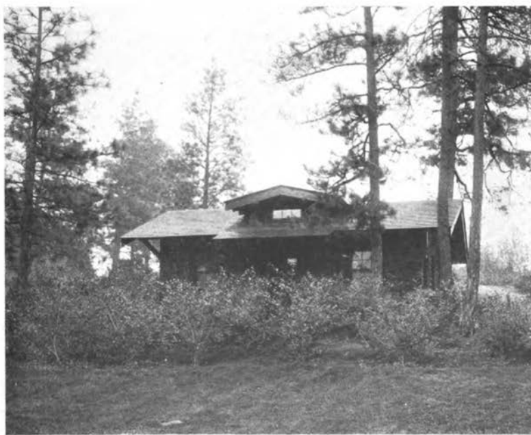
Lavatory Building, Cliff Park
