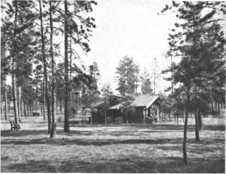
Lavatory Building, Franklin Park
