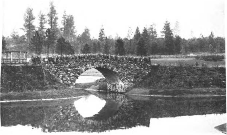
Rustic Bridge, Cannon Hill Park
