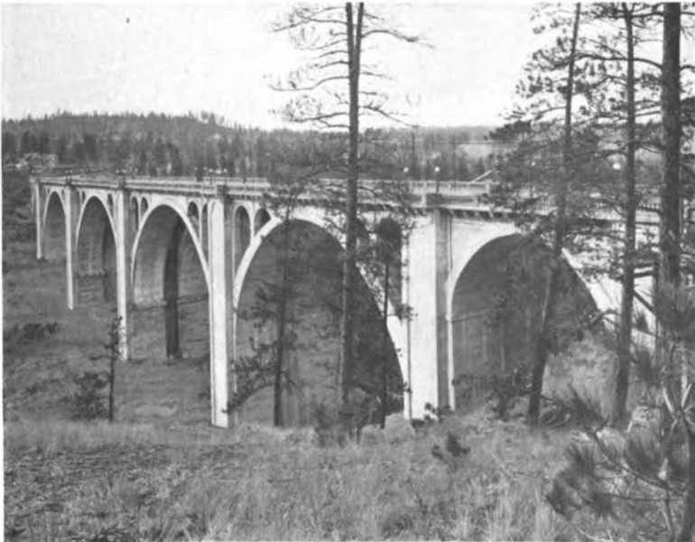
Latah Bridge, High Bridge Park
