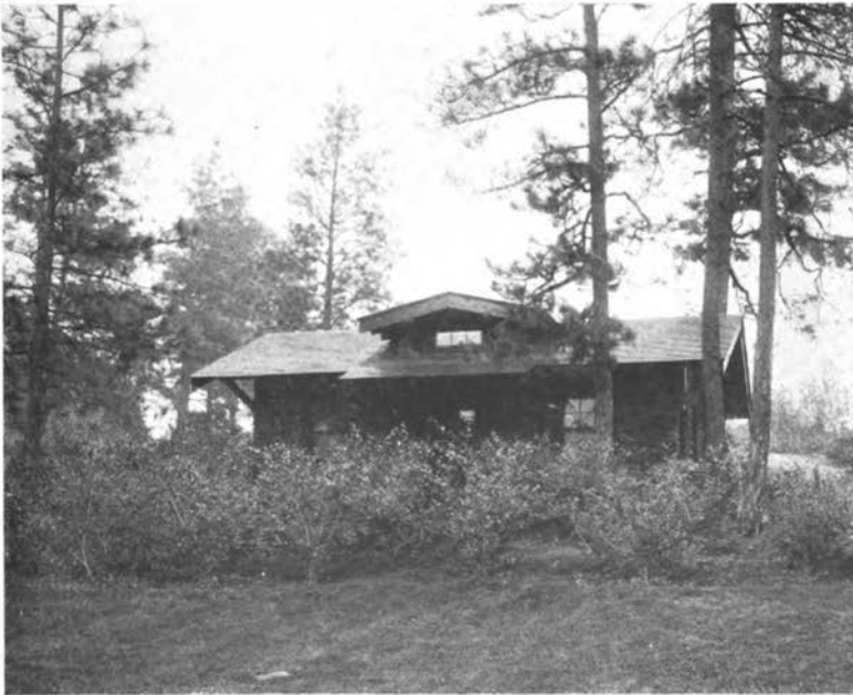
Lavatory Building, Cliff Park
