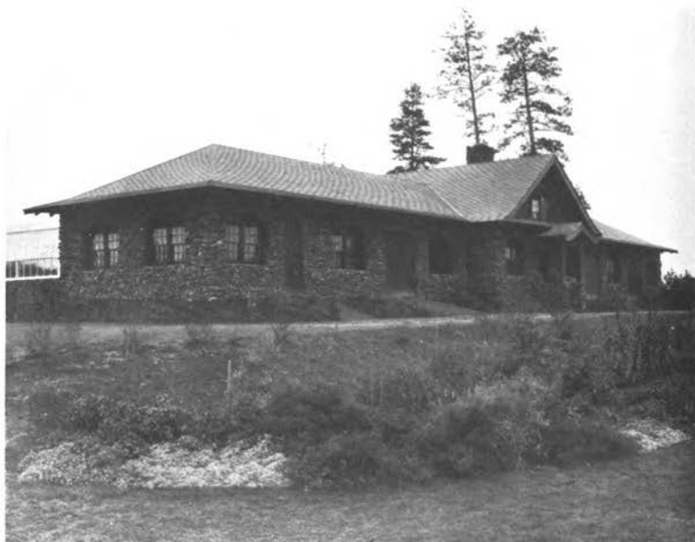
Tool House and Work Room, Manito Park
