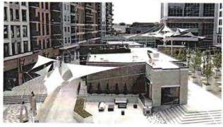
An interesting feature is a suspended floating strut placed into the fabric structure in order to avoid having to place a post to the ground, while simultaneously creating an opportunity for 3d shaping which offers more stability and strength across the system.
