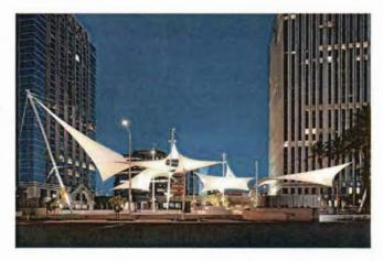
The project held many challenges being an existing site build spanning over an existing parking garage. One of the more unique features of this project is the double cone shown in the photo. This large stable shape provides dramatic interest and large shade with minimal structure. The shade and accompanying plantings along with a coffee bar has brought the plaza to life.
