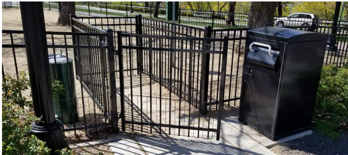
Image B.4 - The entry corral at the Downtown Spokane Dog Park is small, but includes locking latches and a paved surface up to the gate. A trash receptacle, drinking fountain, and street light are located immediately around the entry for a safe experience and convenient use.
