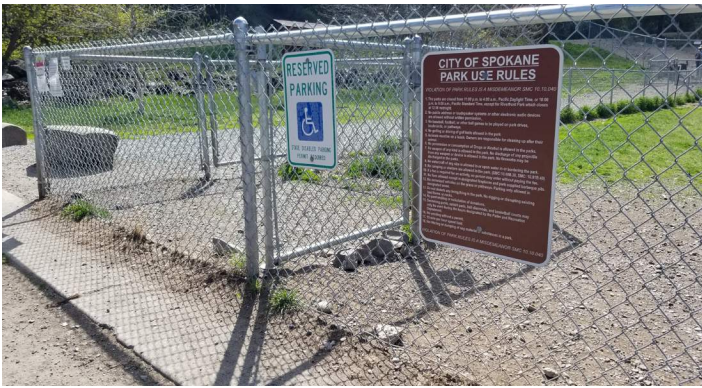
Image B.5 - The corral at the small dog park area for High Bridge Park. The gravel surface has eroded leaving large gaps under the fence small dogs can escape through. There is no paved access to the gates.
