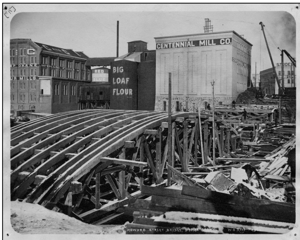
Figure 3-2. 1908 photograph showing construction of the Howard Street North Channel Bridge (Courtesy of Washington State Archives).
