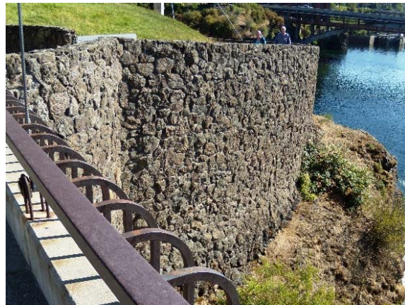
18. Examples of infrastructure – concrete retaining walls, planters on South Channel and basalt retaining wall at the end of Suspension Bridge.
