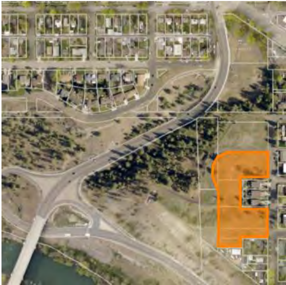
Downriver Stormwater Facility 2.8 acres
