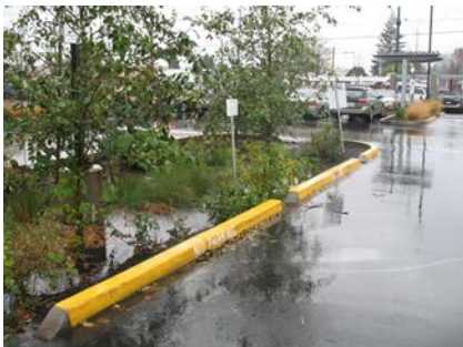
Curbs can be constructed to allow unconcentrated distribution of stormwater flow into swales.
