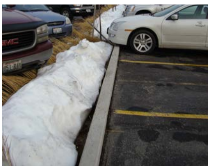
Integrate snow storage with stormwater facilities, or preferably designate parking stalls or other paved areas adjacent to stormwater facilities for snow storage.
