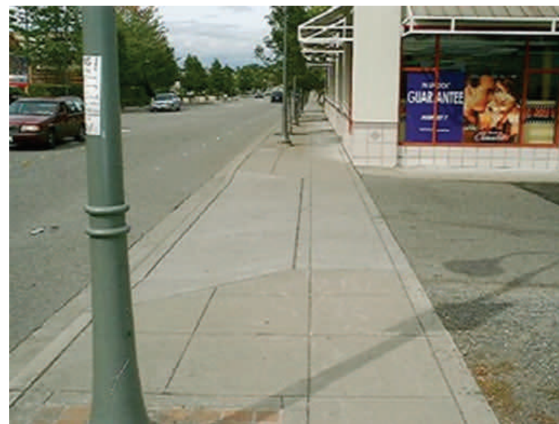
Sidewalk pattern is visibly continuous
