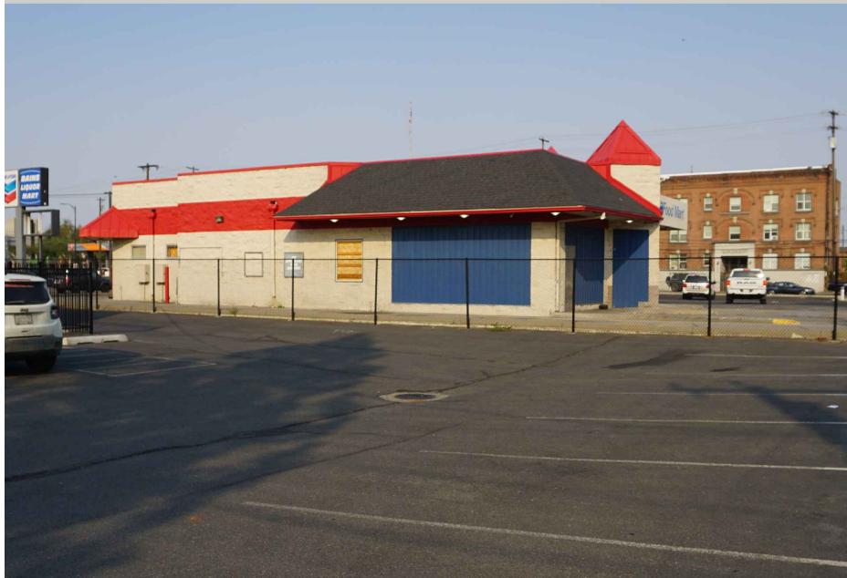
2 VIEW FROM 4th AVE FACING SOUTH
