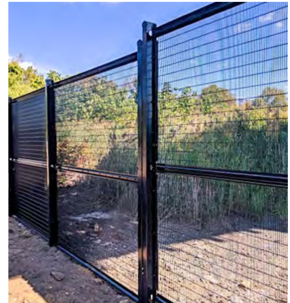
STEEL STANCHION WITH WELDED WIRE MESH INFILL
