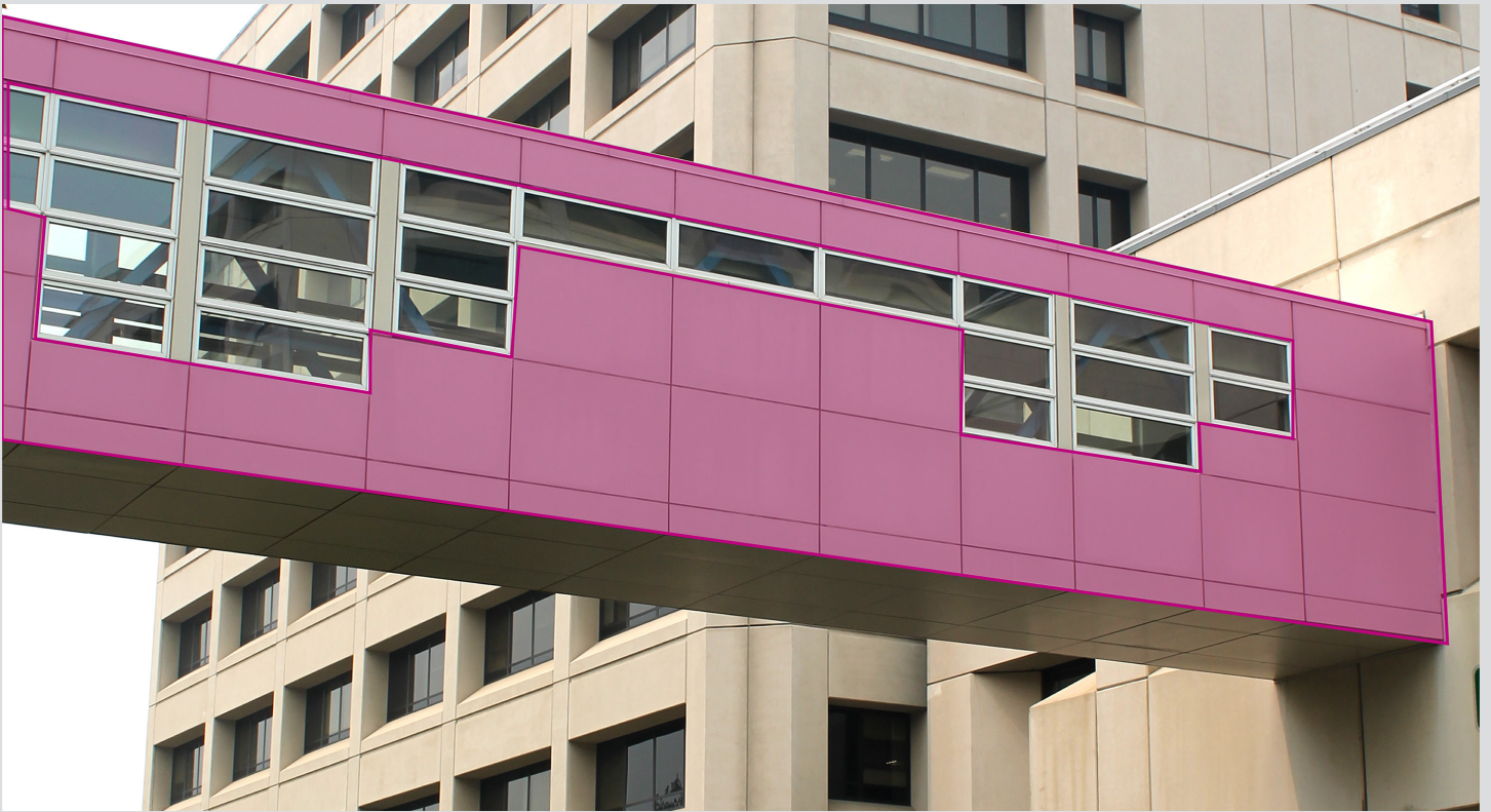
An example of a skywalk using a more insulated exterior wall.
