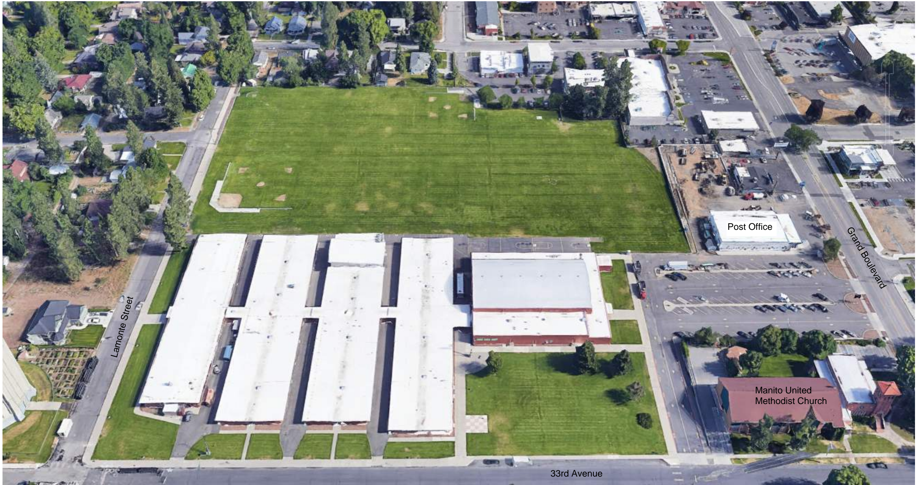
Overall site, looking north
