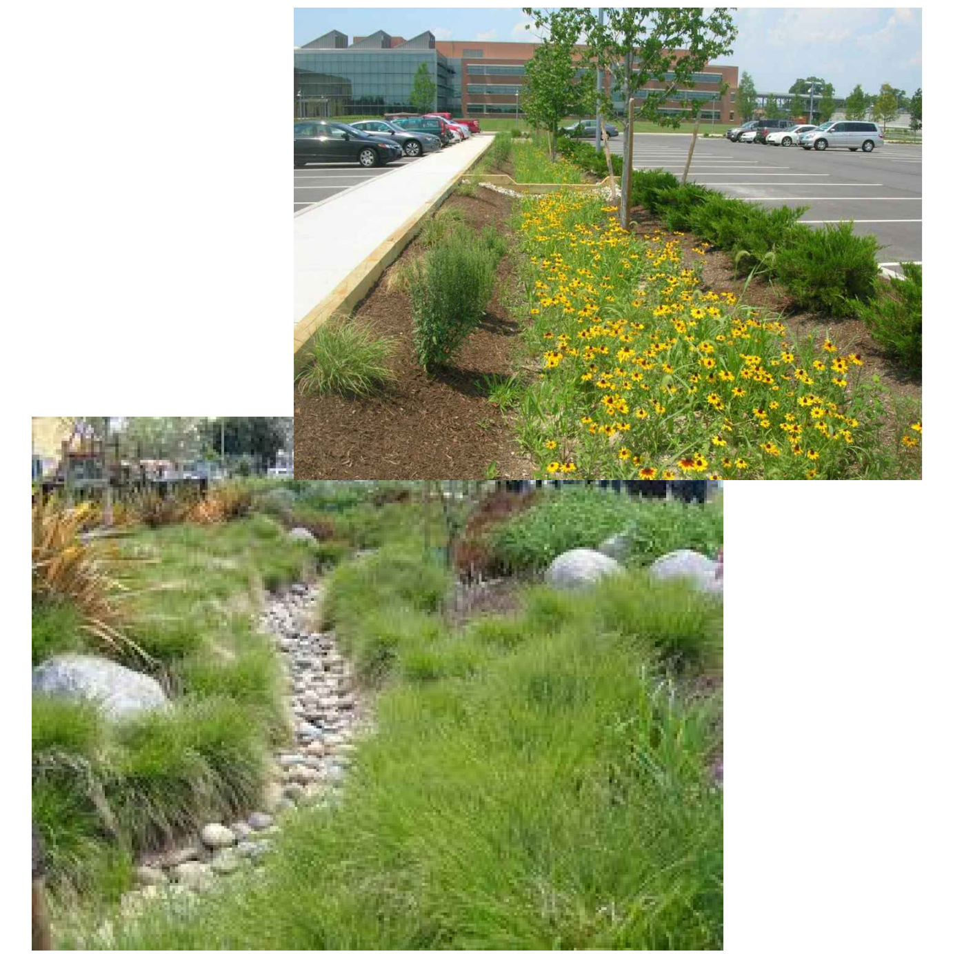
BIORETENTION STORMWATER SWALE CHARACTER
