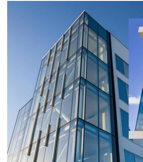
Curtain Wall System w/ clear and spandrel glass
