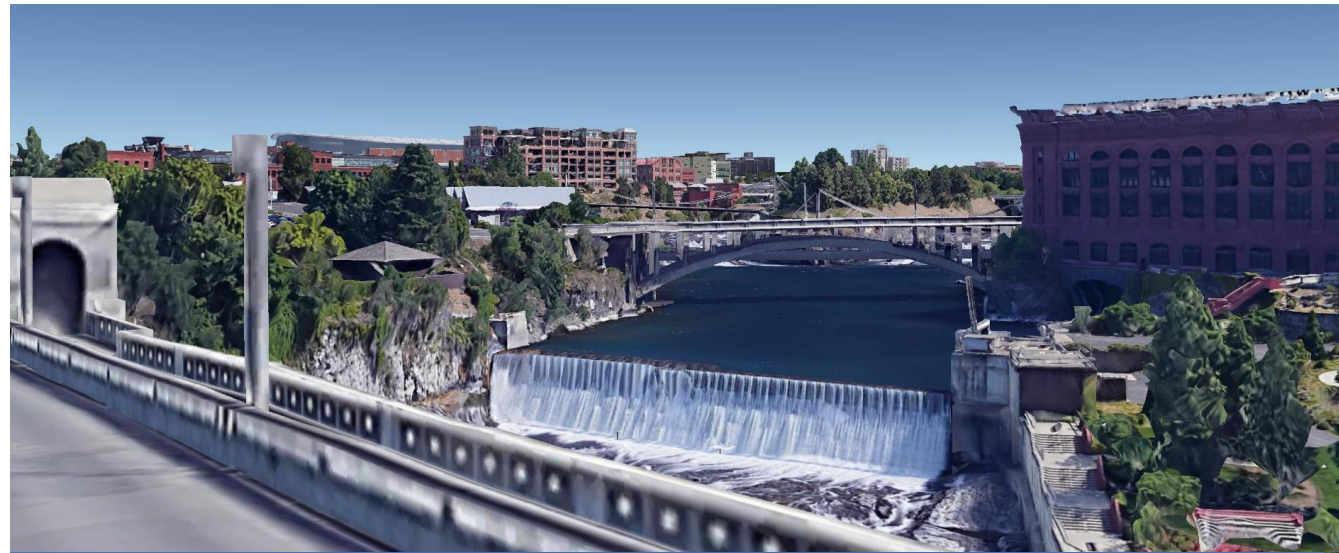
View from Monroe Street Bridge – Looking East
